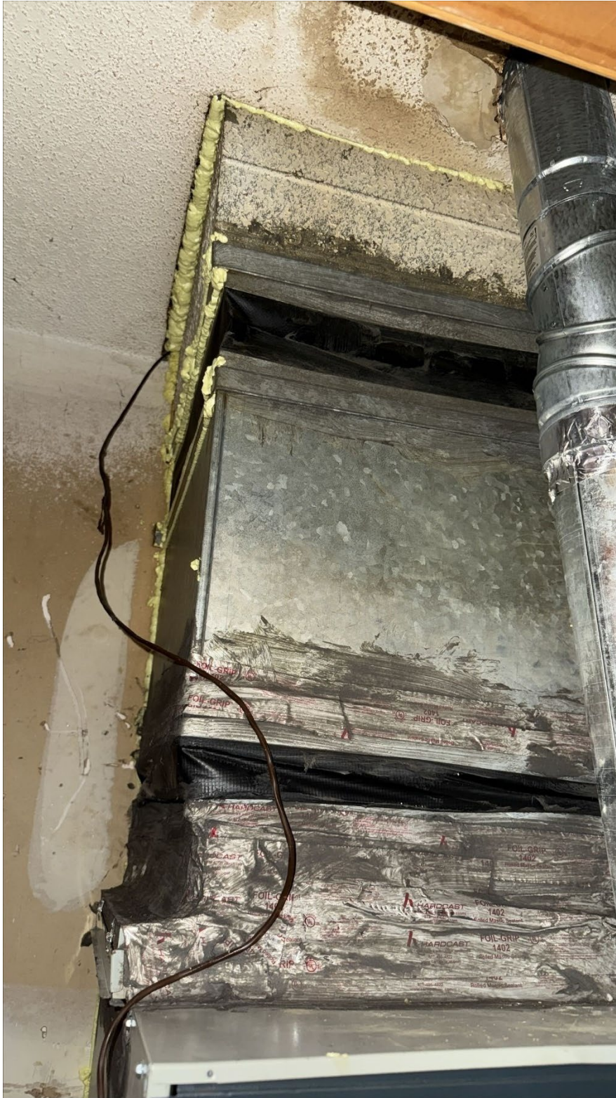
Figure 11-2: Duct Sealing Project- Mastic, Mastic Tape & Spray foam on Air Handler
