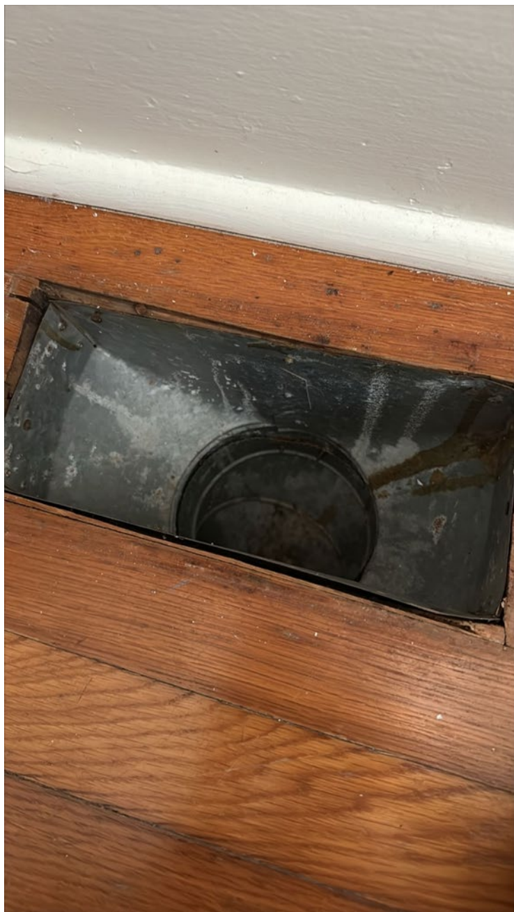
FIGURE 0-3 EA-0004064776, EA-0004831640 AOGWP DUCT SEALING PROJECT
