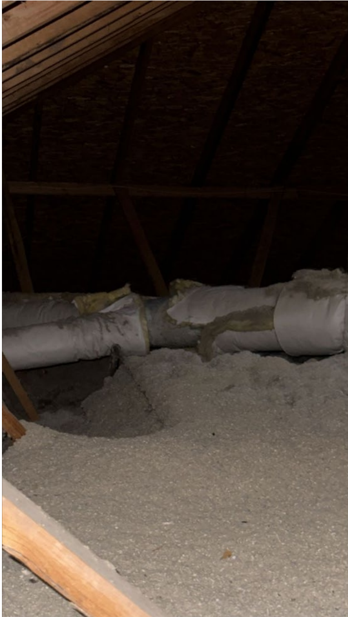
FIGURE 0-1 EA-0004215774 AOWP DUCT SEALING PROJECT
