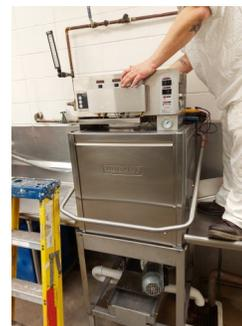
The HVAC class installed a new dishwasher in the kitchen. The class soldered all the copper pipes from the ceiling to the floor.
