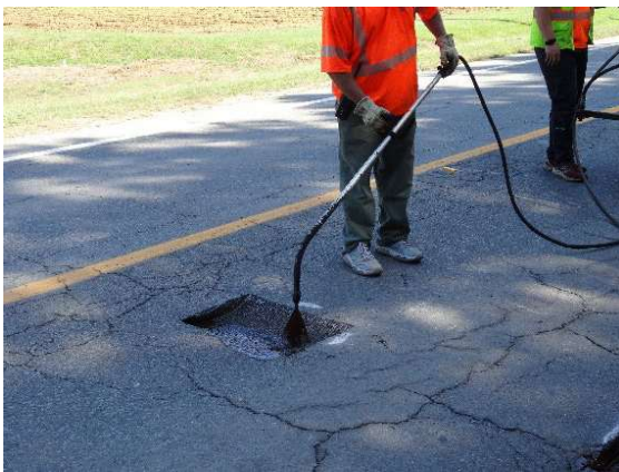
(c) Spraying Tack Coat on a Grooved Milled Patch
