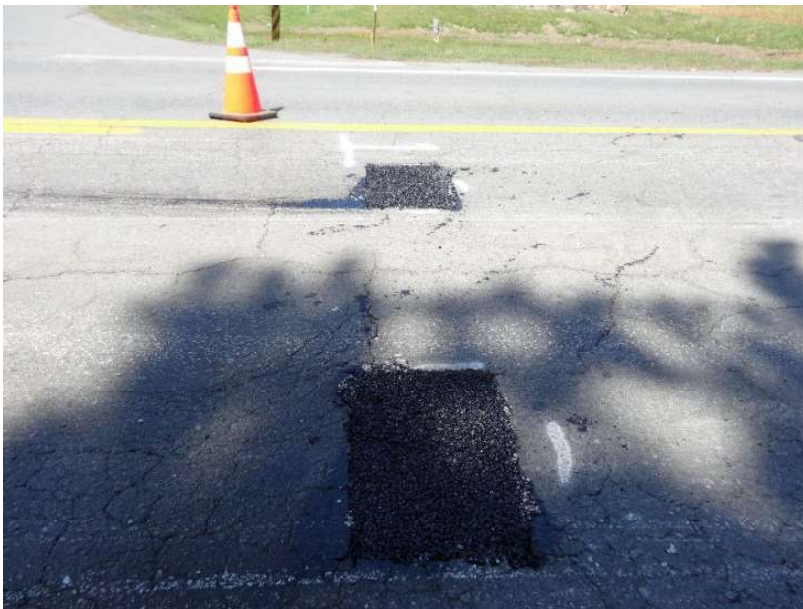
Figure 12. HPCM Material After Placement and Compaction
