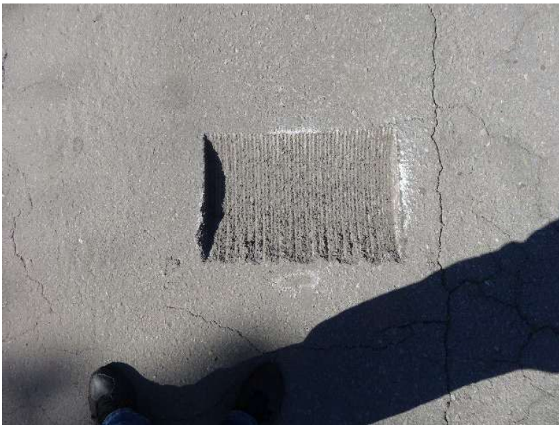
Figure 4. Clean Rectangular Groove After Milling
