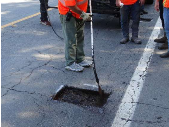
(a) Spraying Tack Coat on a Rectangular Cut
