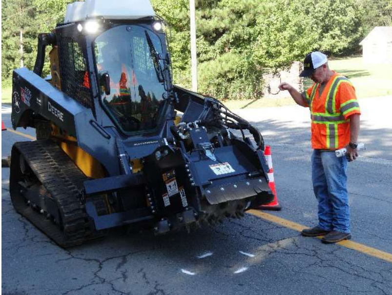
Figure 3. Pothole Creation by Milling
