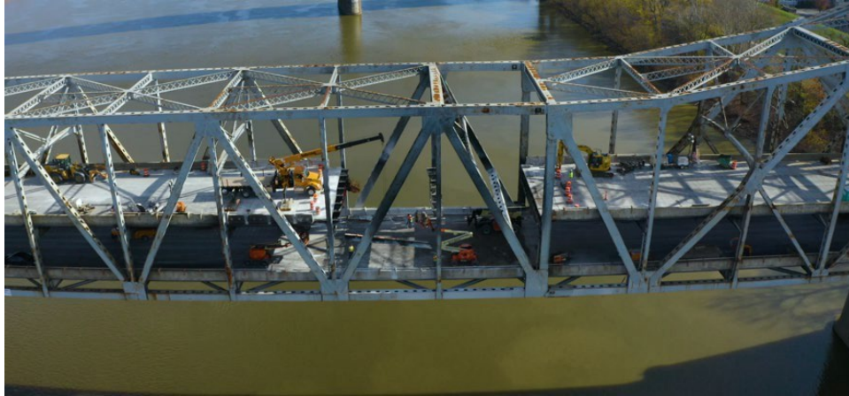
(a) Span of the Brent Spence Bridge under repair (Ref: WDRB)
