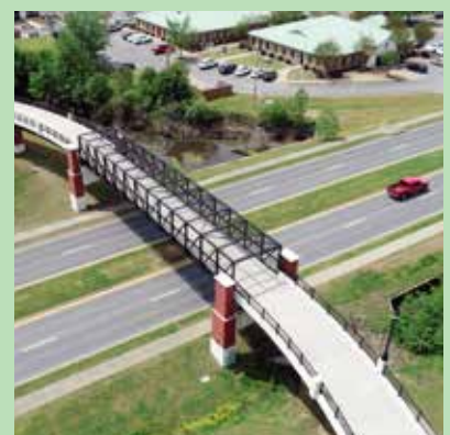
Dave Ward Drive Pedestrian Overpass Conway, Arkansas
