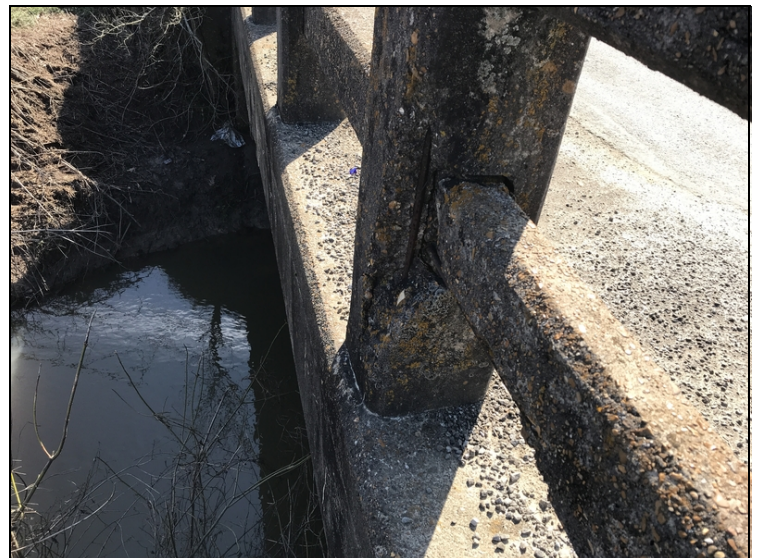
3rd concrete post on Left is cracked & spalled with 2' of rebar exposed.
