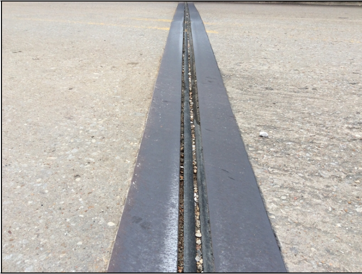
Bent #1 compression joint seal-Adhesion failure.
