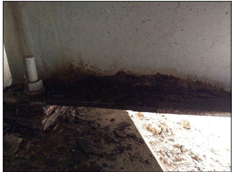
Abutment #2, Beam #3 corrosion with flaking rust to web and bottom flange.
