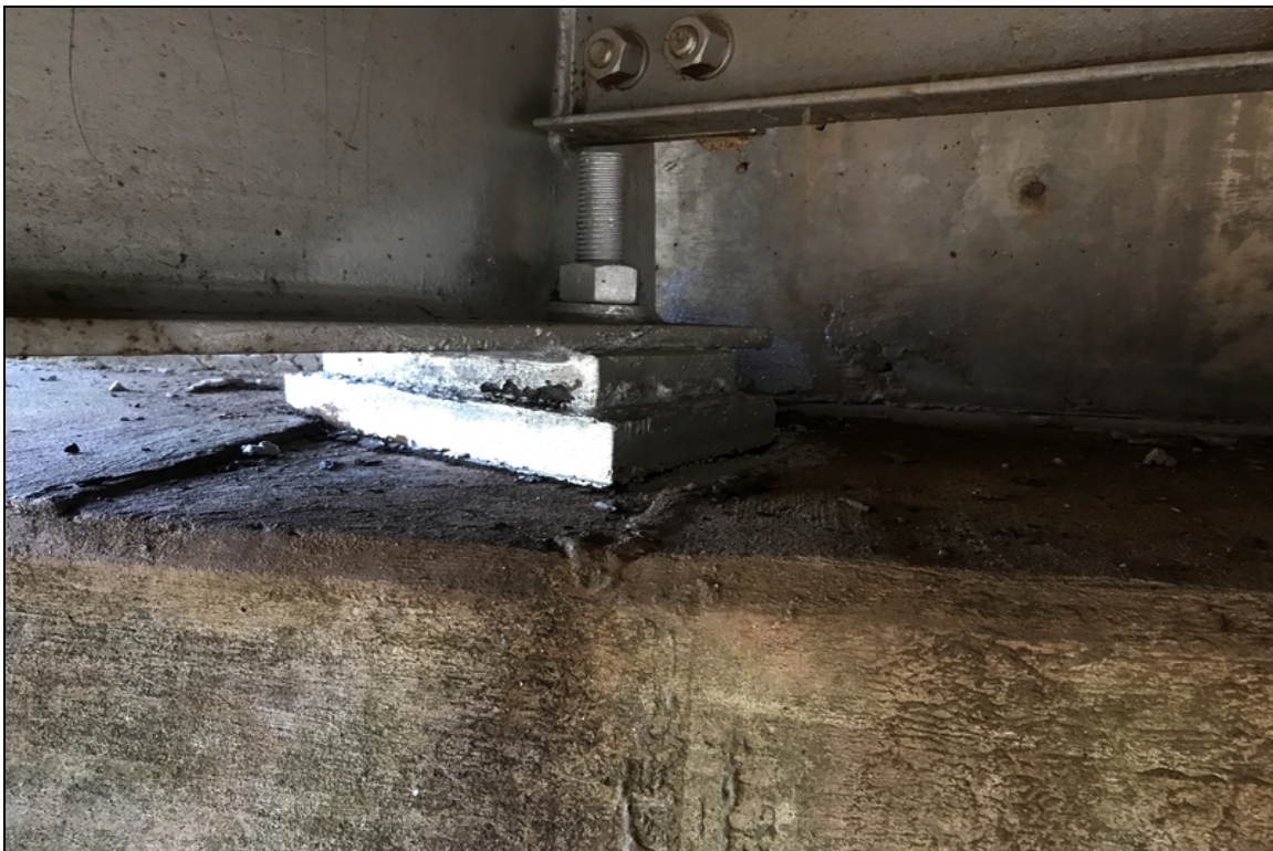
Abutment #2 bearing paint repair attempt
