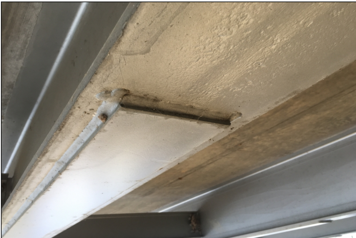
Typical cover plate detail.
