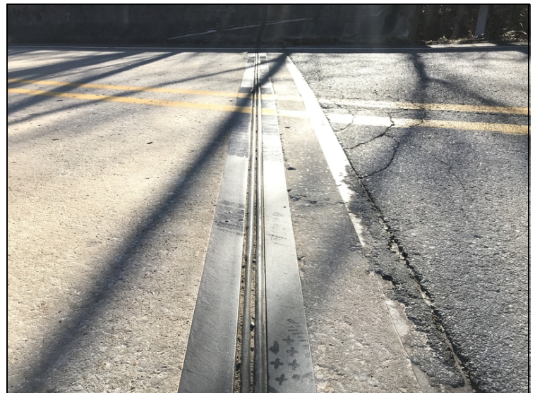
Abutment #1 joint material.
