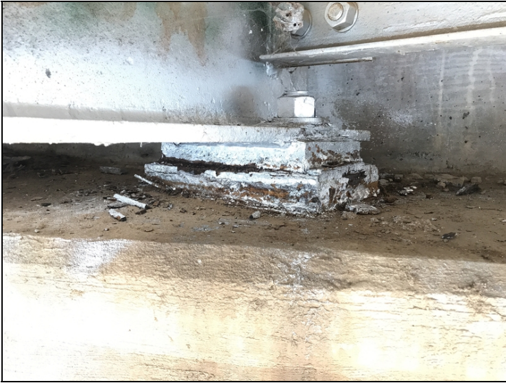
Abutment #2 bearing #3 flaking with a failed paint repair.
