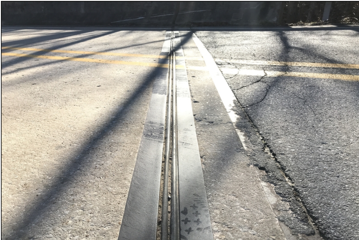
Abutment #1 joint material.
