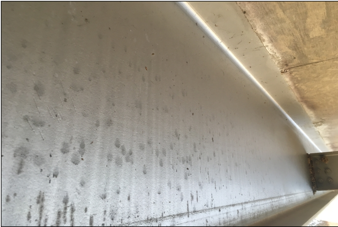
General paint condition except at the beam ends.
