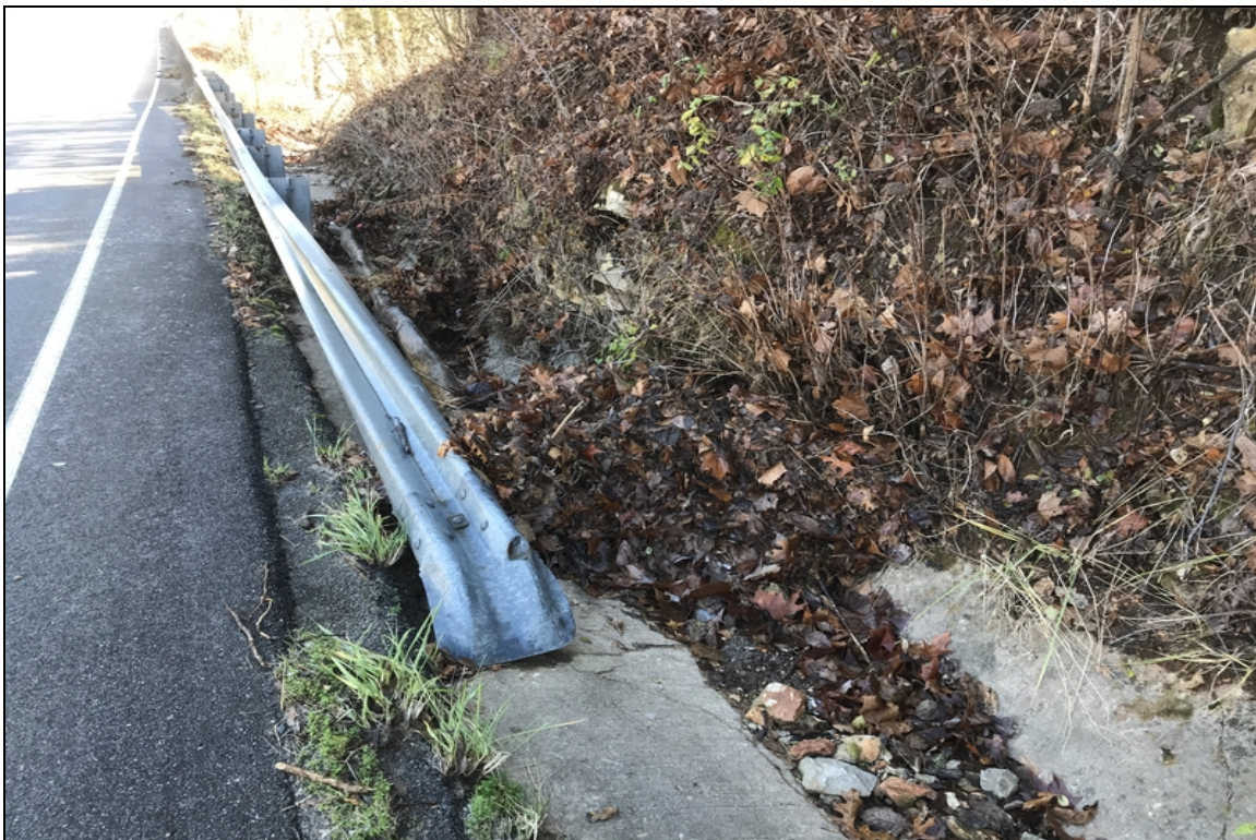
Drift accumulation in ditch paving possibly redirecting water to roadway.
