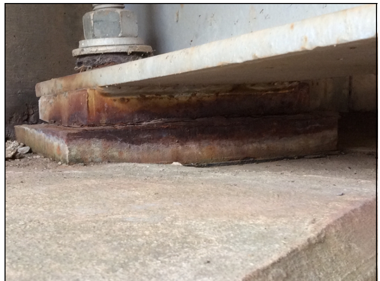
Abutment #2, bearing #1-Corrosion with flaking rust.
