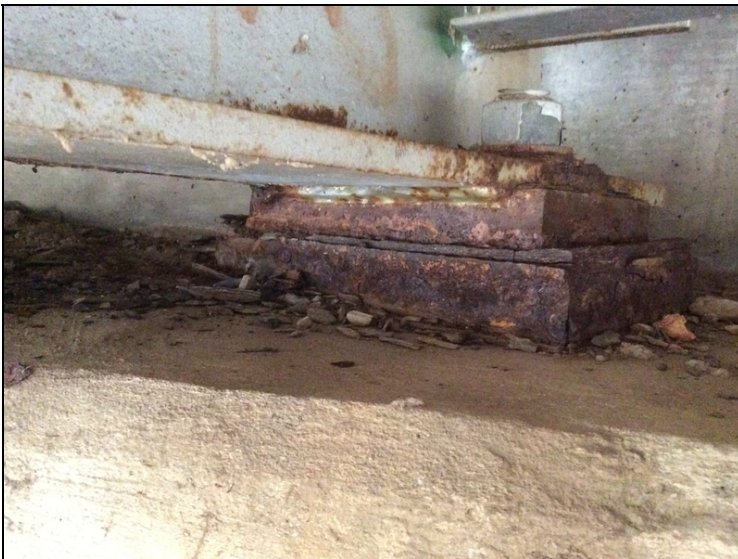
Abutment #2, bearing #3-Corrosion with heavy flaking rust.
