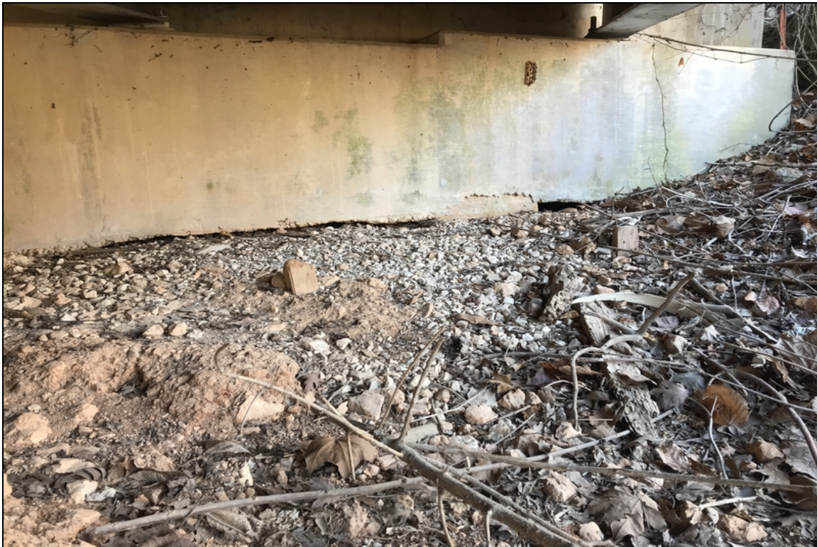
Abutment #1 left signs of embankment settlement.
