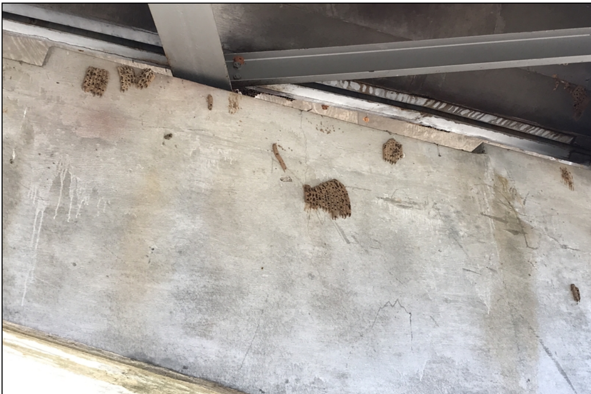
Pier #2 behind and ahead vertical face of hammerhead cap at bearing #3 has a short duration vertical crack.
