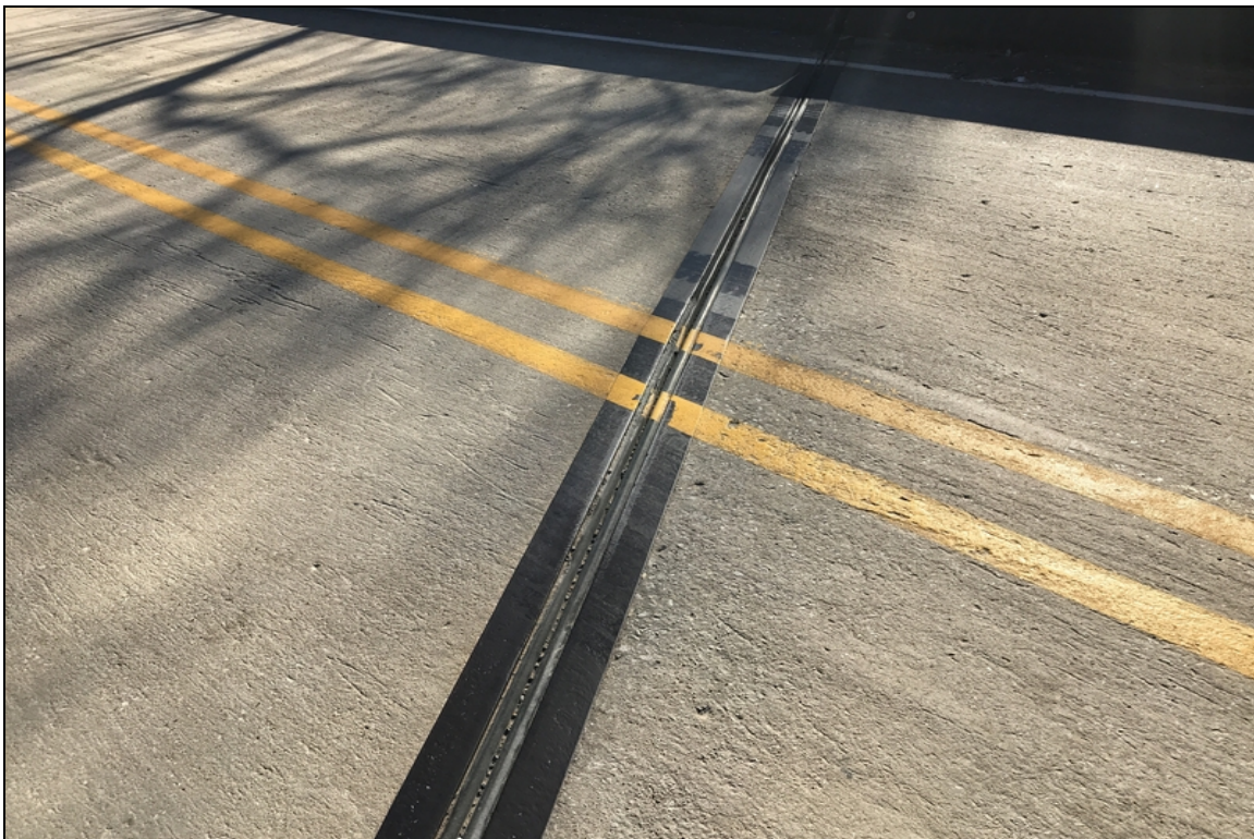
Bent #2 joint material cracking and minor debris impact.
