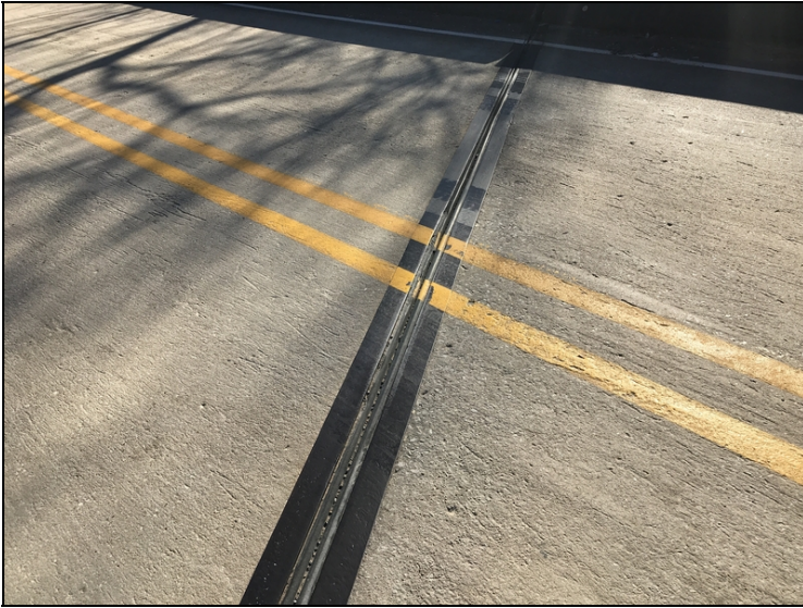
Bent #2 joint material cracking and minor debris impaction.
