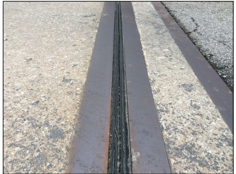
Abutment #1-Deteriorated compression joint seal.
