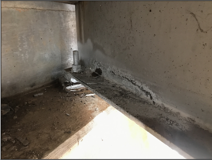
Beam #3 at abutment #2 flaking rust with failed paint repair.
