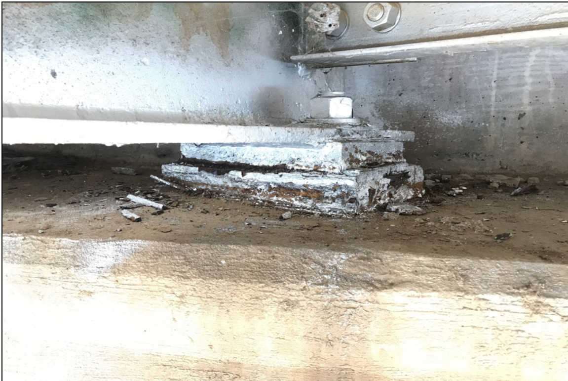
Abutment #2 bearing #3 flaking with a failed paint repair.
