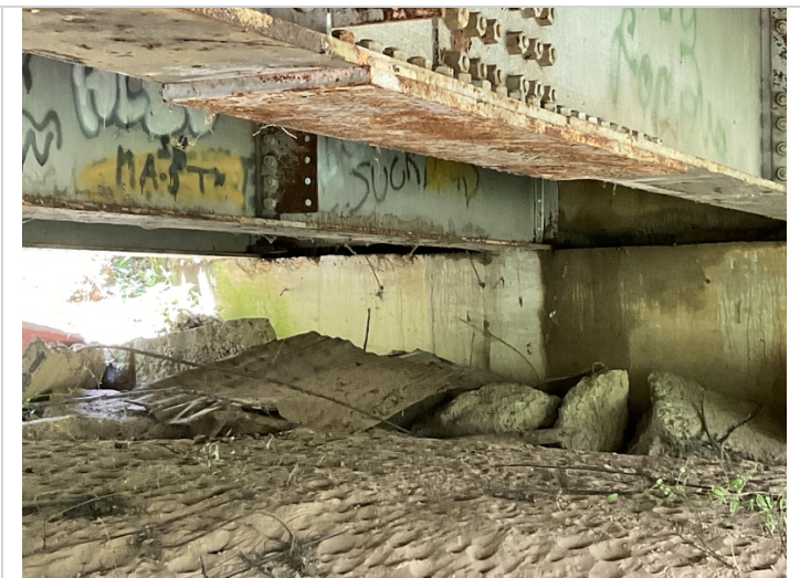
6/22 concrete alignment in good shape. Small spall abutment 2 top edges
