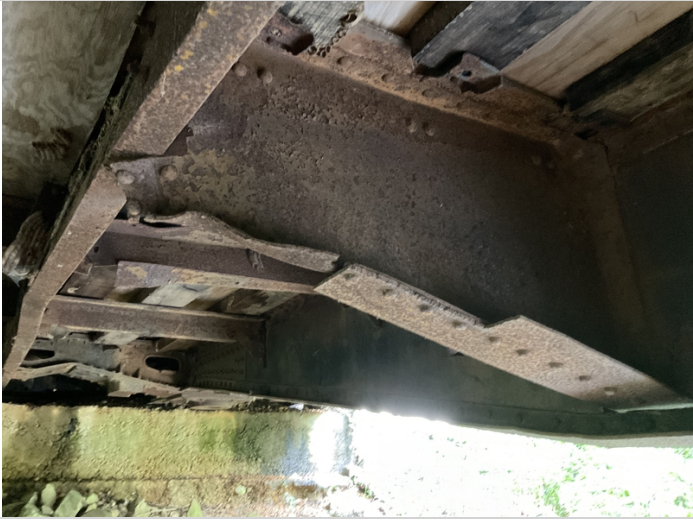
Damage to bracing on inside of beam 1
