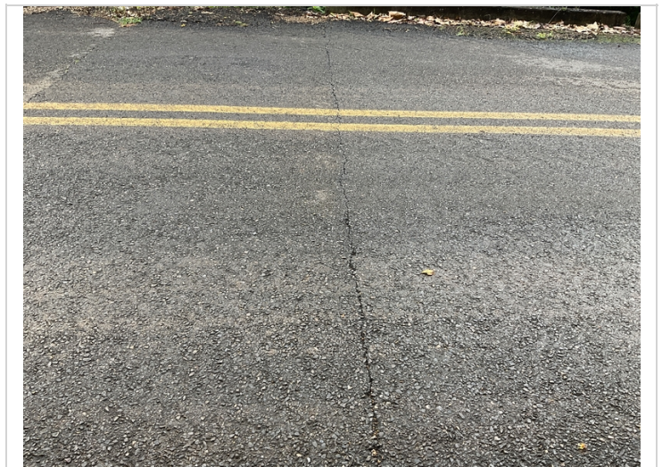
Cracking in wearing surface
