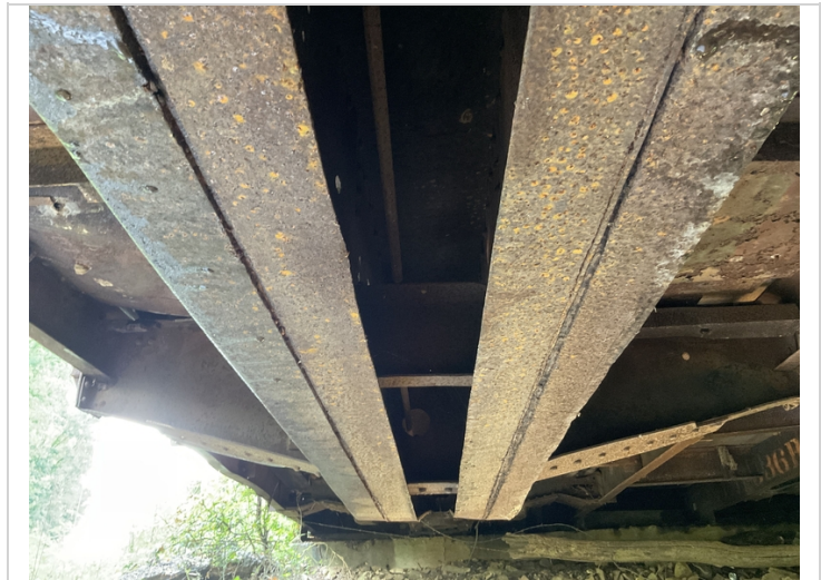
Corrosion on beams
