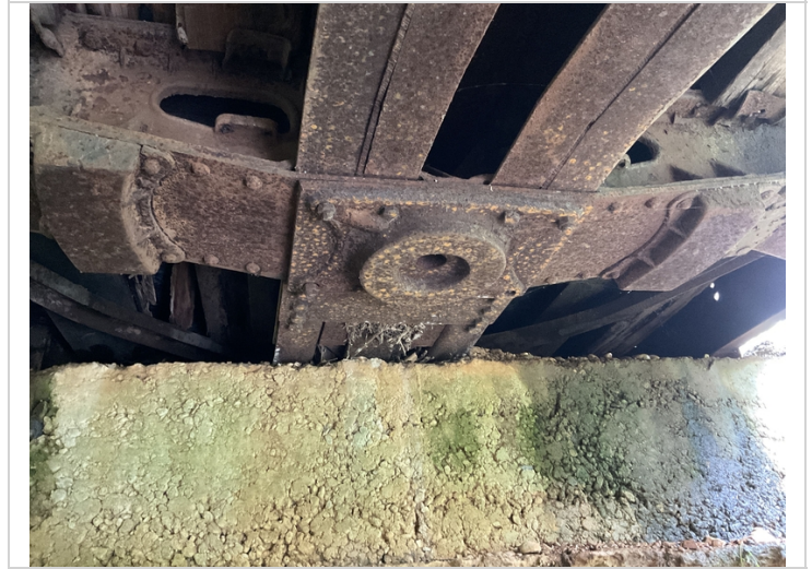
Beam 1 bolster at bent 1
