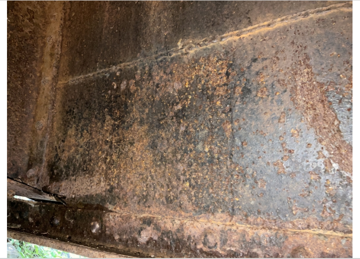
Corrosion on beams
