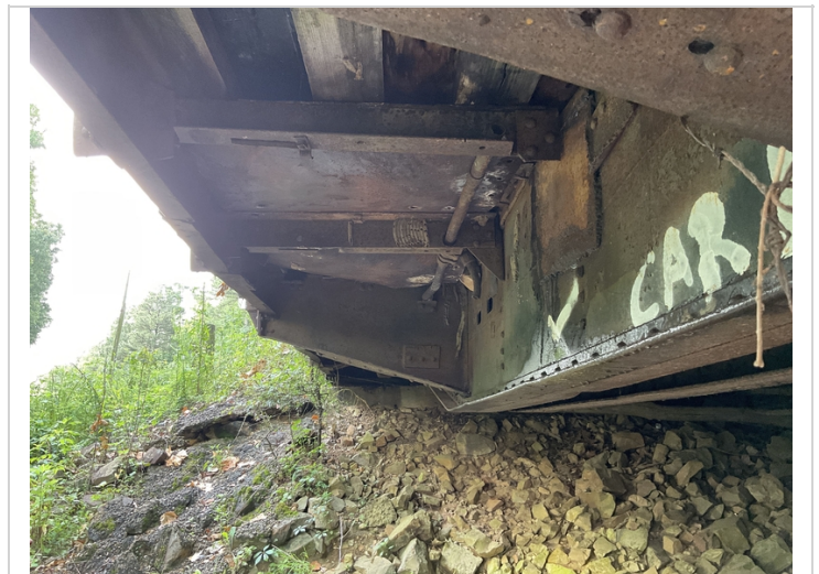
Outside bracing at beam 1
