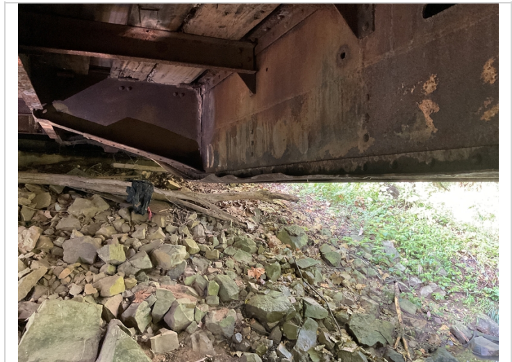
Old damage to beam 2
