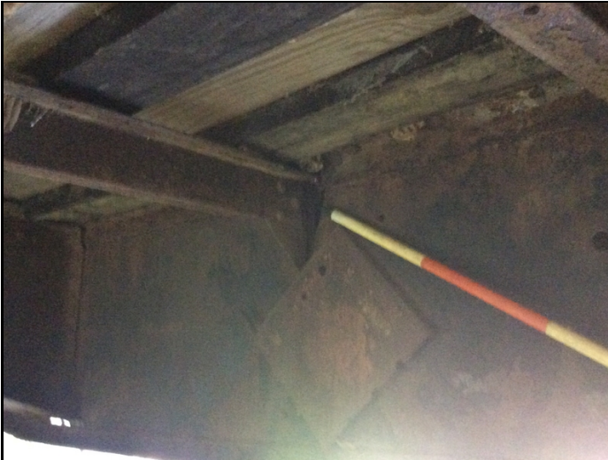
Inside of car plate over crack. Crack still visible at top of sill
