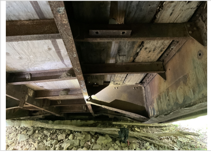
Bracing on inside of beam 2
