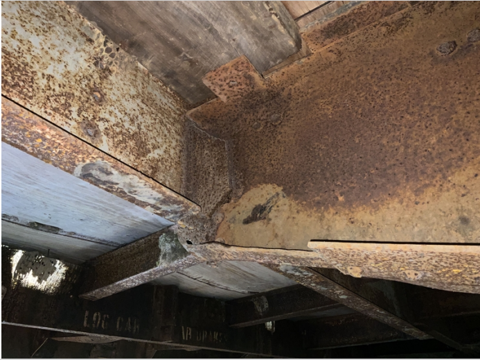
Stringer 2 welded on backside
