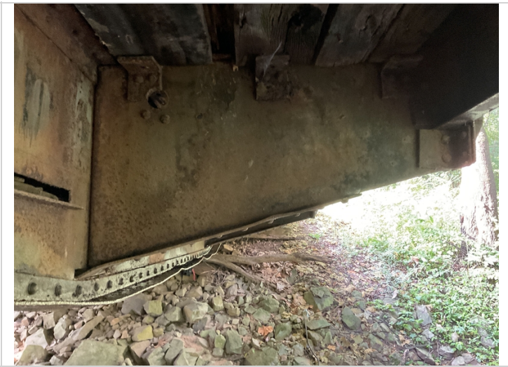
Bracing on outside of beam 2
