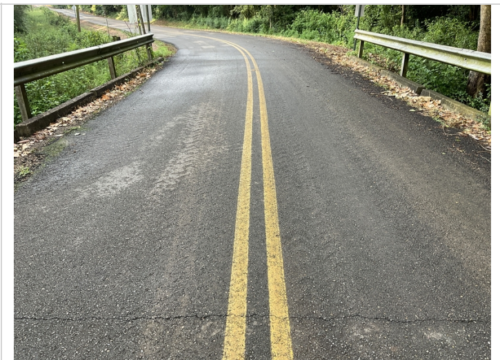
Deck photo. Deck has chip seal overlay
