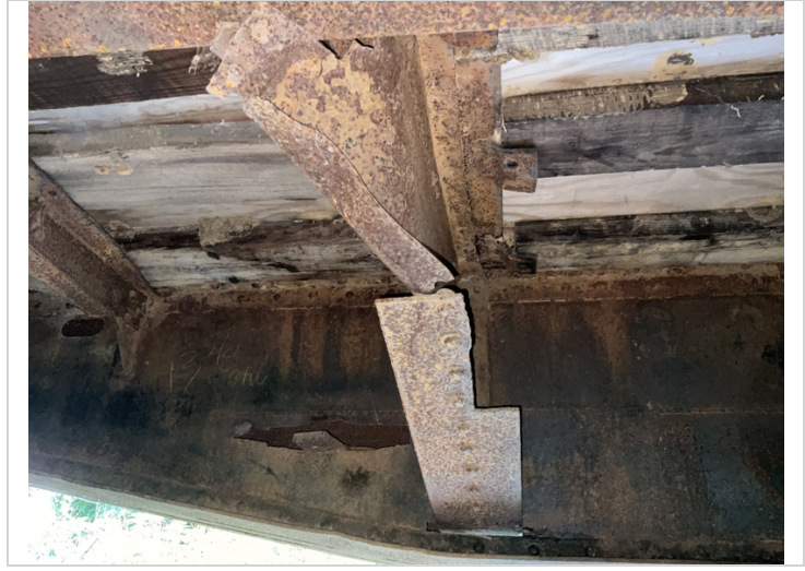
Damage to bracing on inside of beam 1
