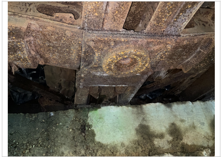
Beam 2 bolster at bent 1
