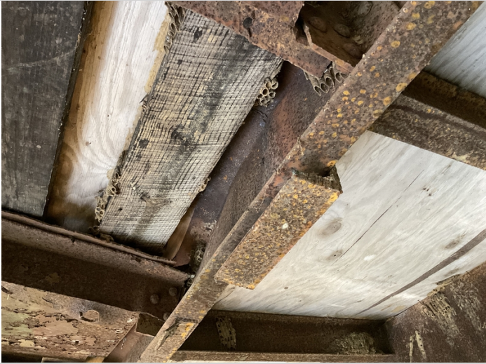
Corrosion on bracing
