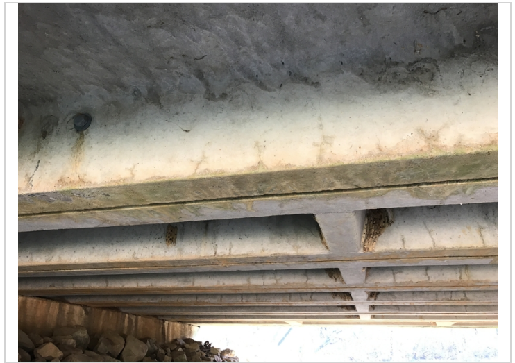
Channel beams
