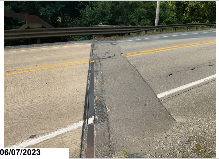
Spalls on top of back wall have been covered with asphalt.
