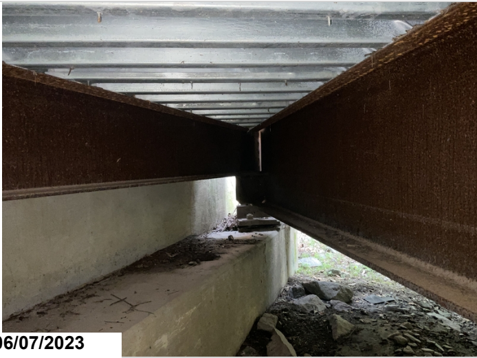
Steel protective coating has heavy granular texture
