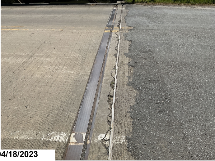
small Spalls in back wall at west end
