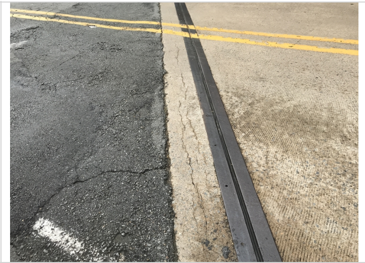
Bent 1 has cracking in backwall
