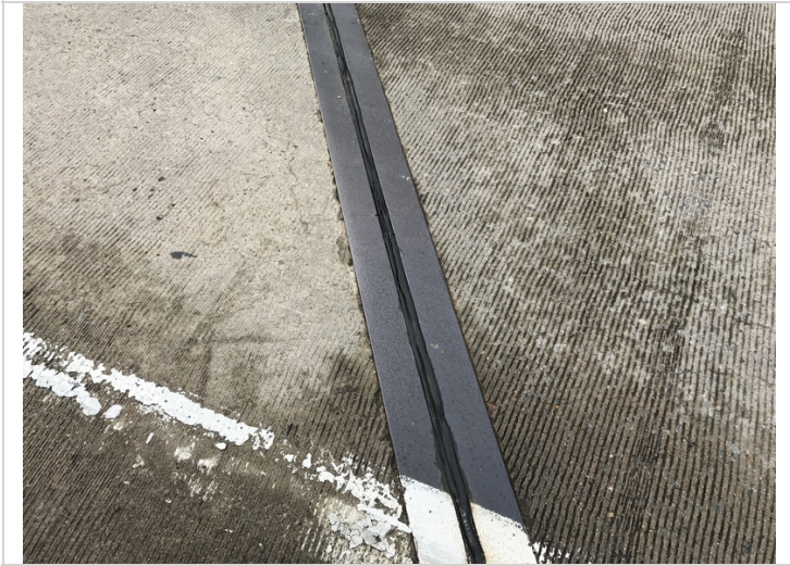
Joints are torn and leaking
