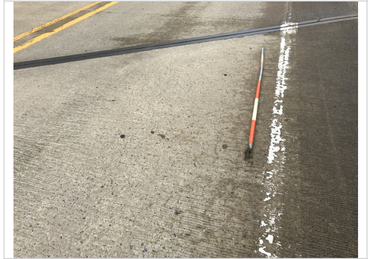
Deck has map cracking
