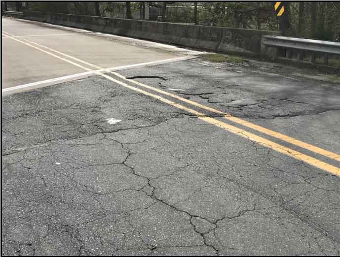
Pothole at bent 4 in the eastbound lane
