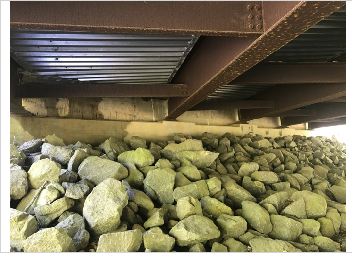
Bent 1 cracks with efflorescence.
