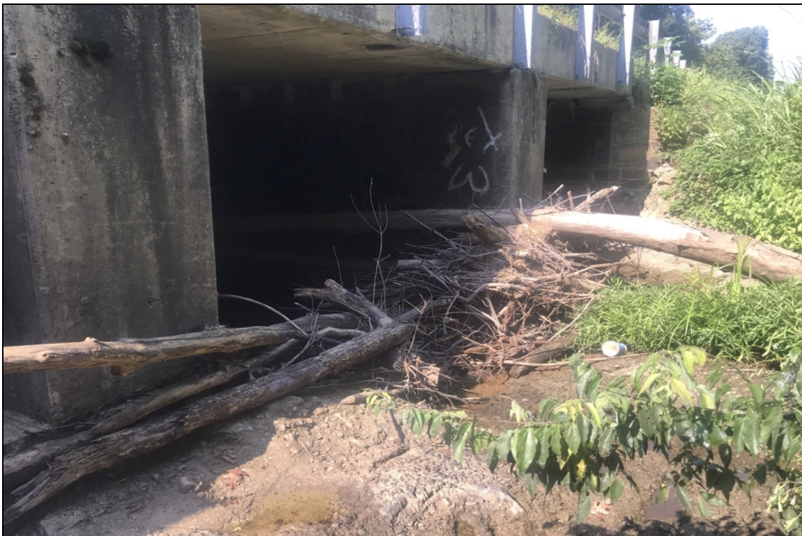
Barrel 2 south side of bridge has logs and debris restricting water flow.
