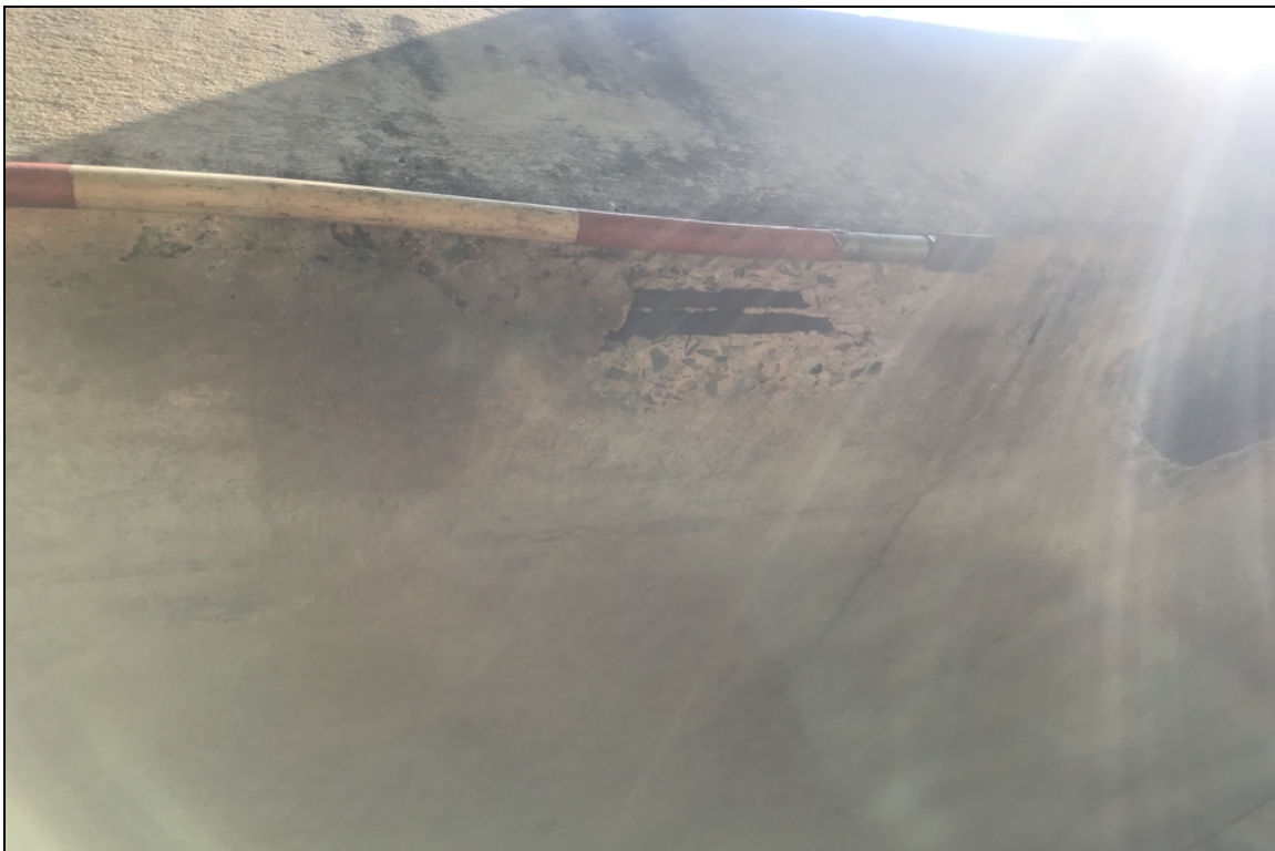
Barrel 2 soffit right side has spall with exposed rebar.
