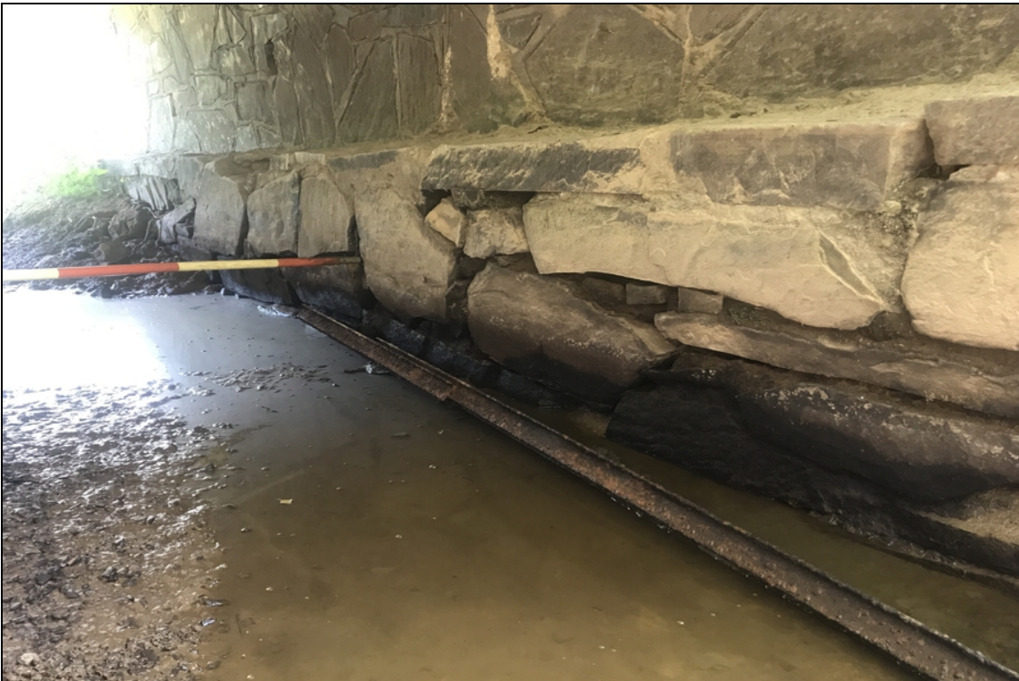
Bent 3 has mortar loss between rocks.
