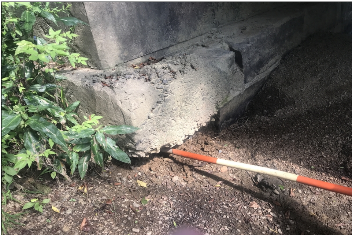
Bent 2 right end scour is partially undermining footing extension.
