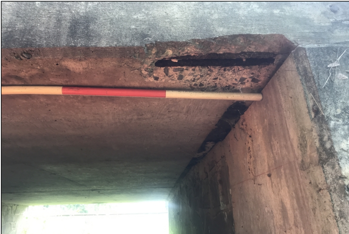
Span 1 soffit near bent 2 has spall with exposed rebar.
