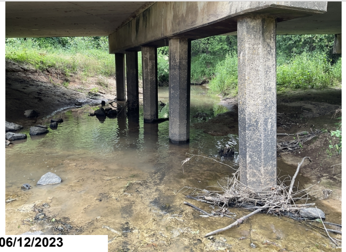
Bent 3 abrasion to piles
