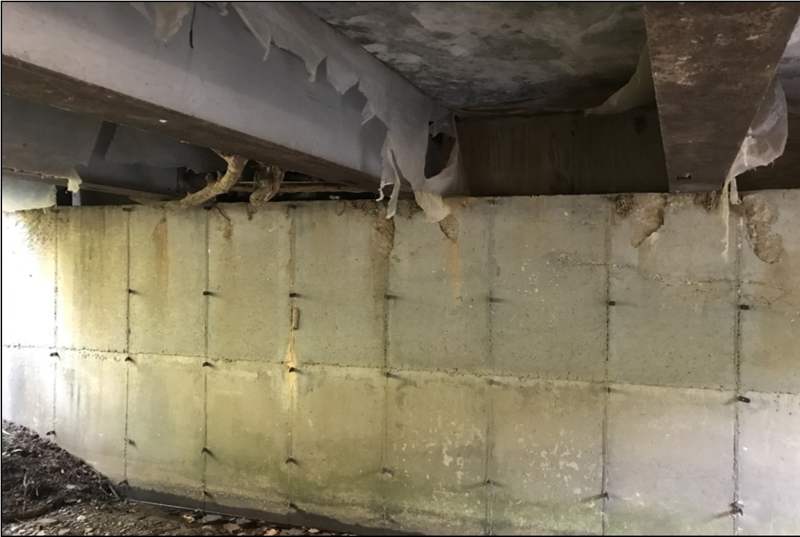
Abutment #1 Typical spalling and delaminated areas under girders.
