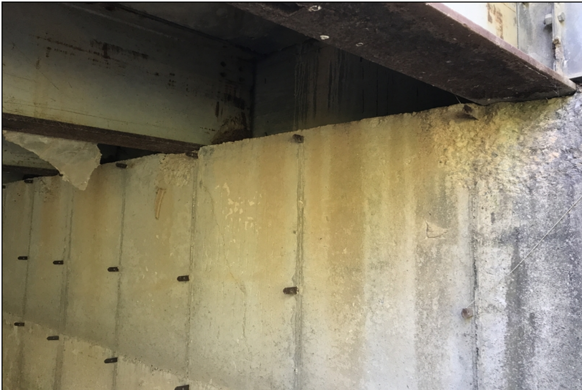
Top of Abutment #2 bearing area under Girders 4 - 6 spalling.
