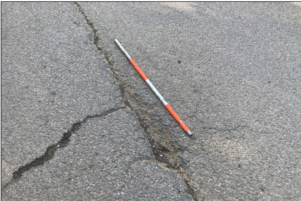
Cracking and spalling of asphalt wearing surface has caused a pothole near centerline of roadway.
