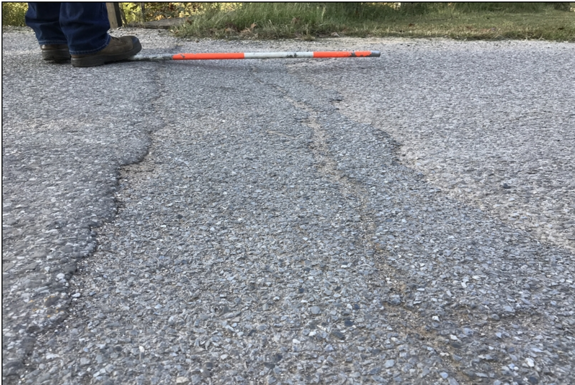
Typical settlement of north approach roadway
