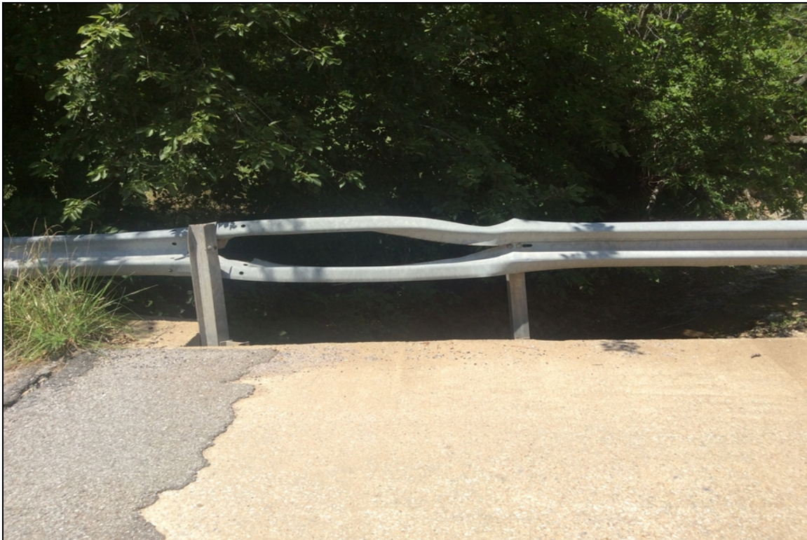
Railing left collision damage adjacent to abutment 1.
