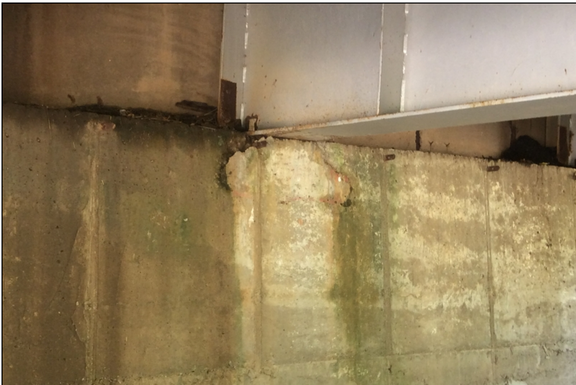
Abutment 1 girder 2 large delaminated area.
