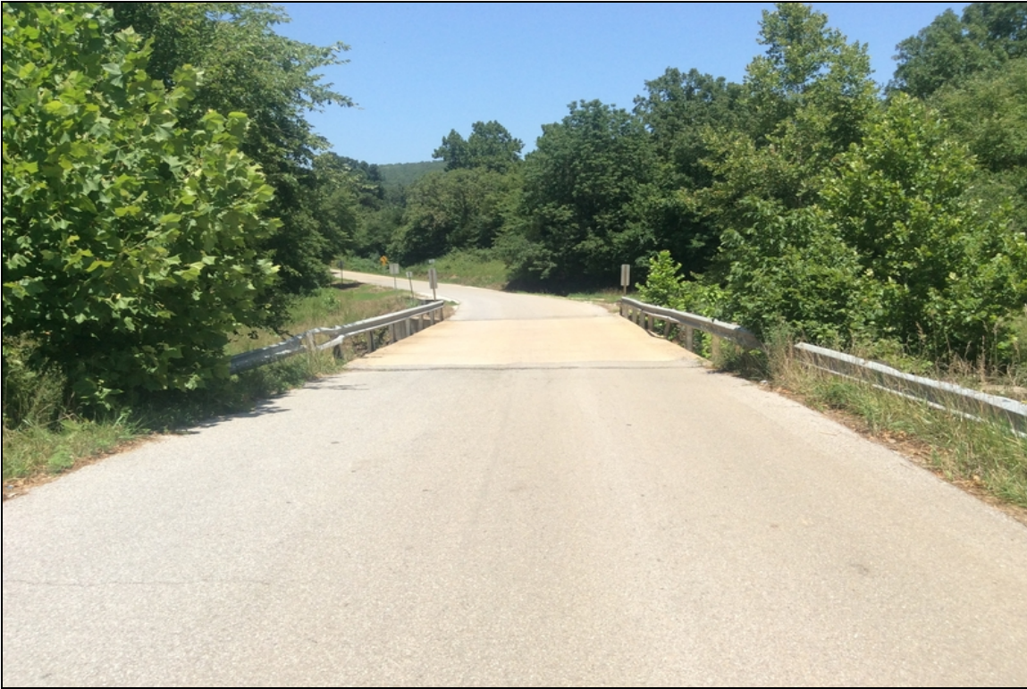
North approach flare boards are missing.
