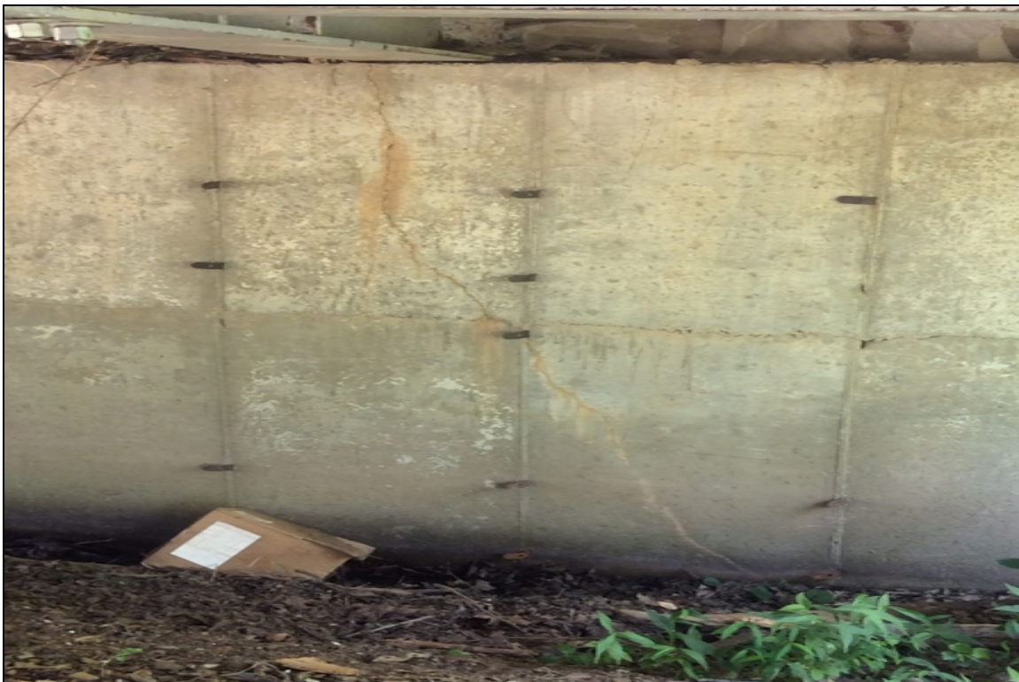
Abutment 2 under girder 3 has a large crack.
