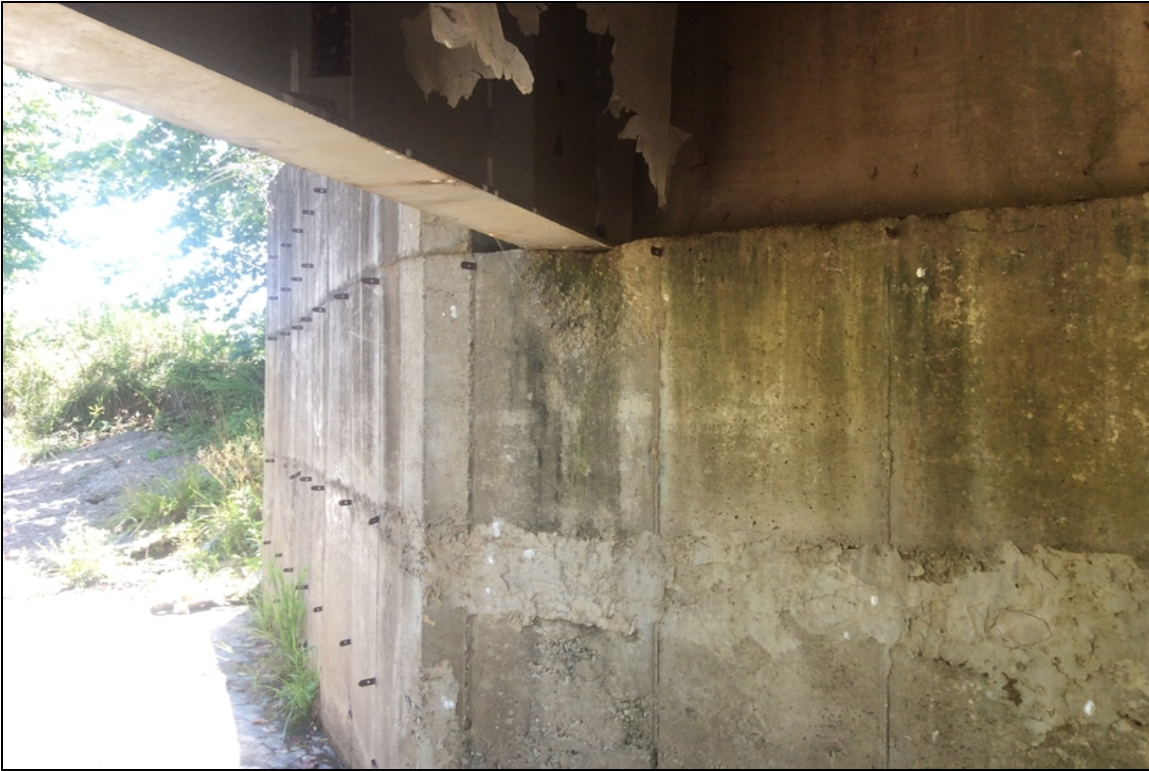
Abutment 1 girder 4 spalling.
