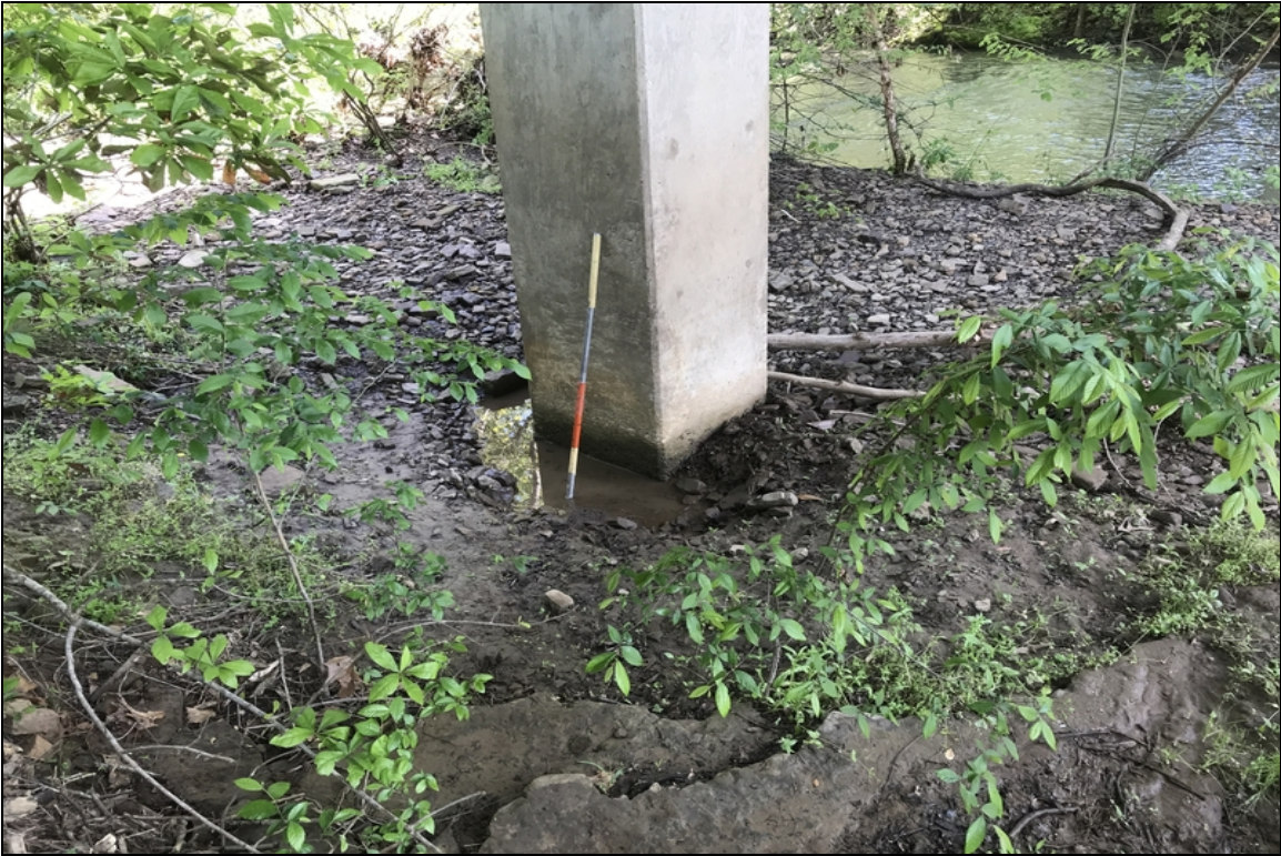
Bent # 2, Column # 1. Top of footing is partially exposed.
