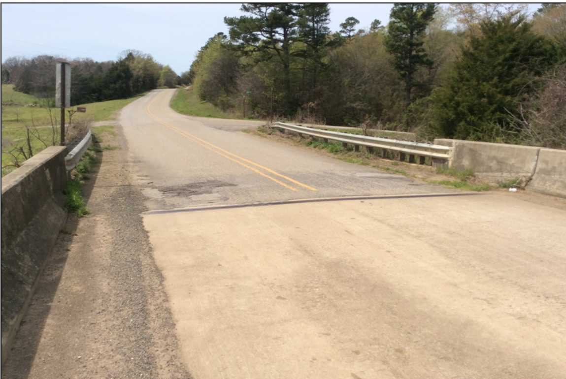
Potholes in the west approach roadway.
