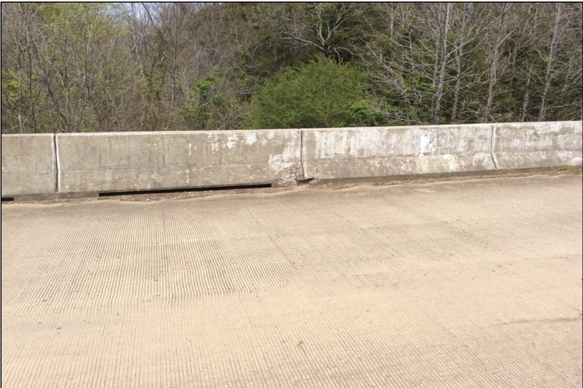
Spalling at the base of the bridge rail in span # 3.
