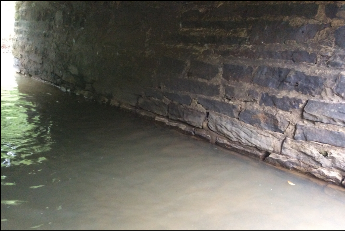
Bent # 2 grout deterioration at the base of the pier wall.
