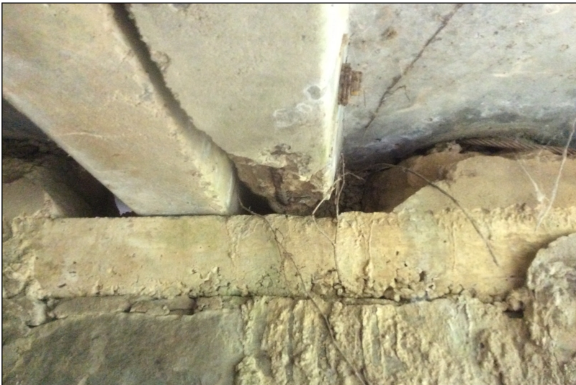
Bent # 2 Span # 1 spalling with exposed reinforcing steel on the RT stem.
