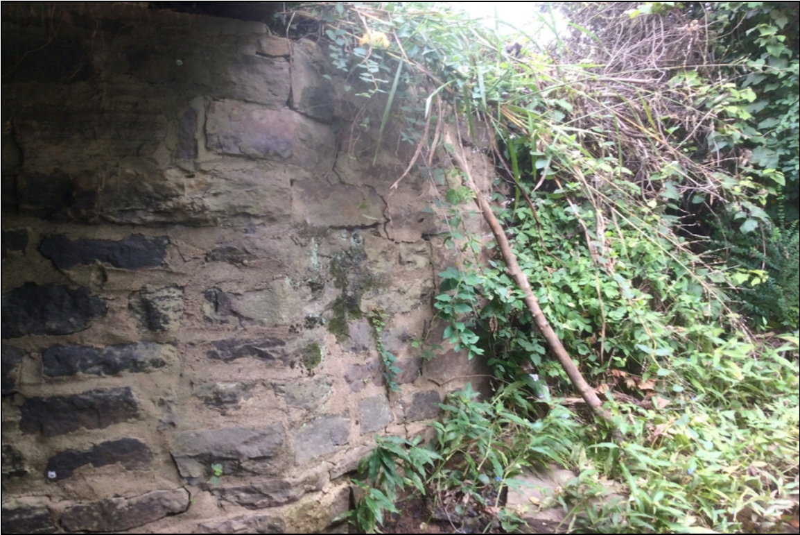
Bent # 1 Lt wing wall cracking with minor rotation towards the channel.
