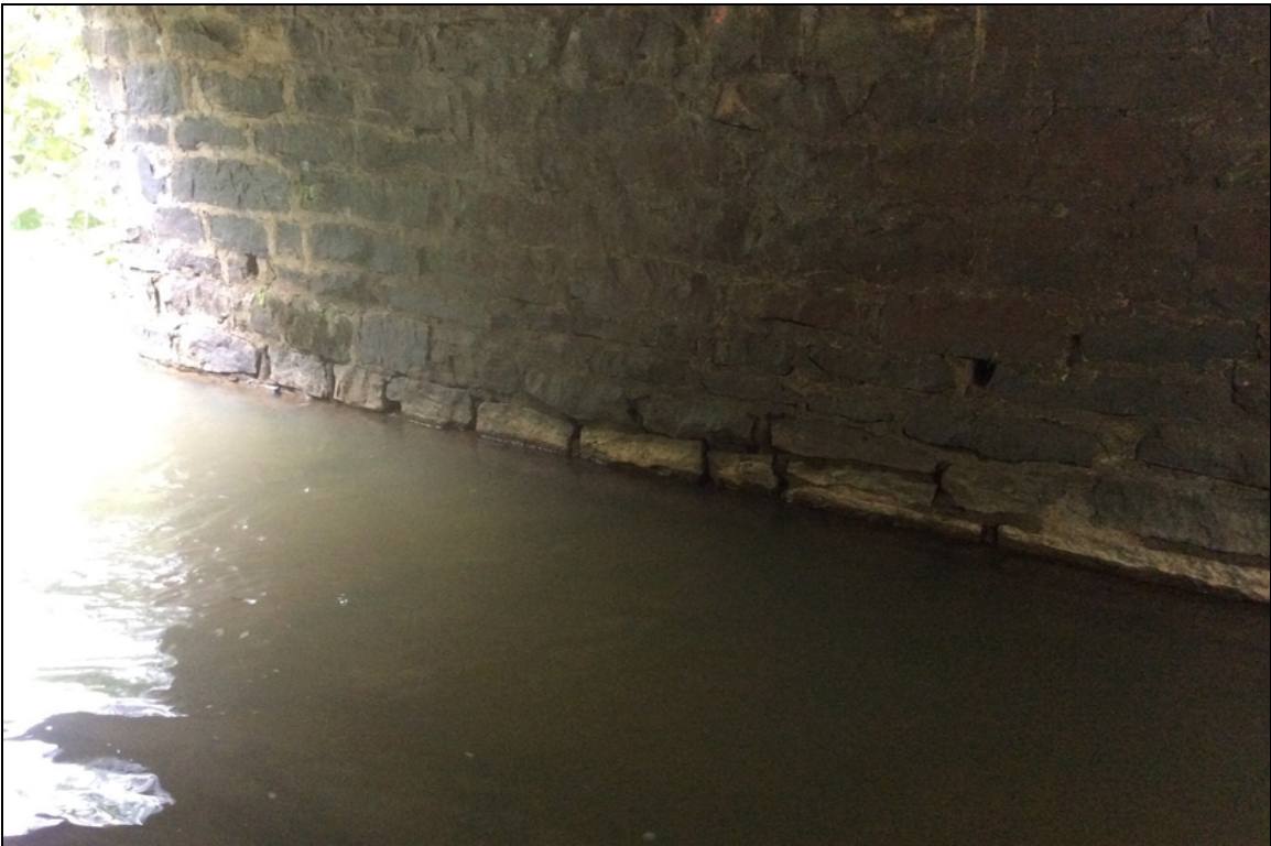
Bent # 1 grout deterioration at the base of the bent.
