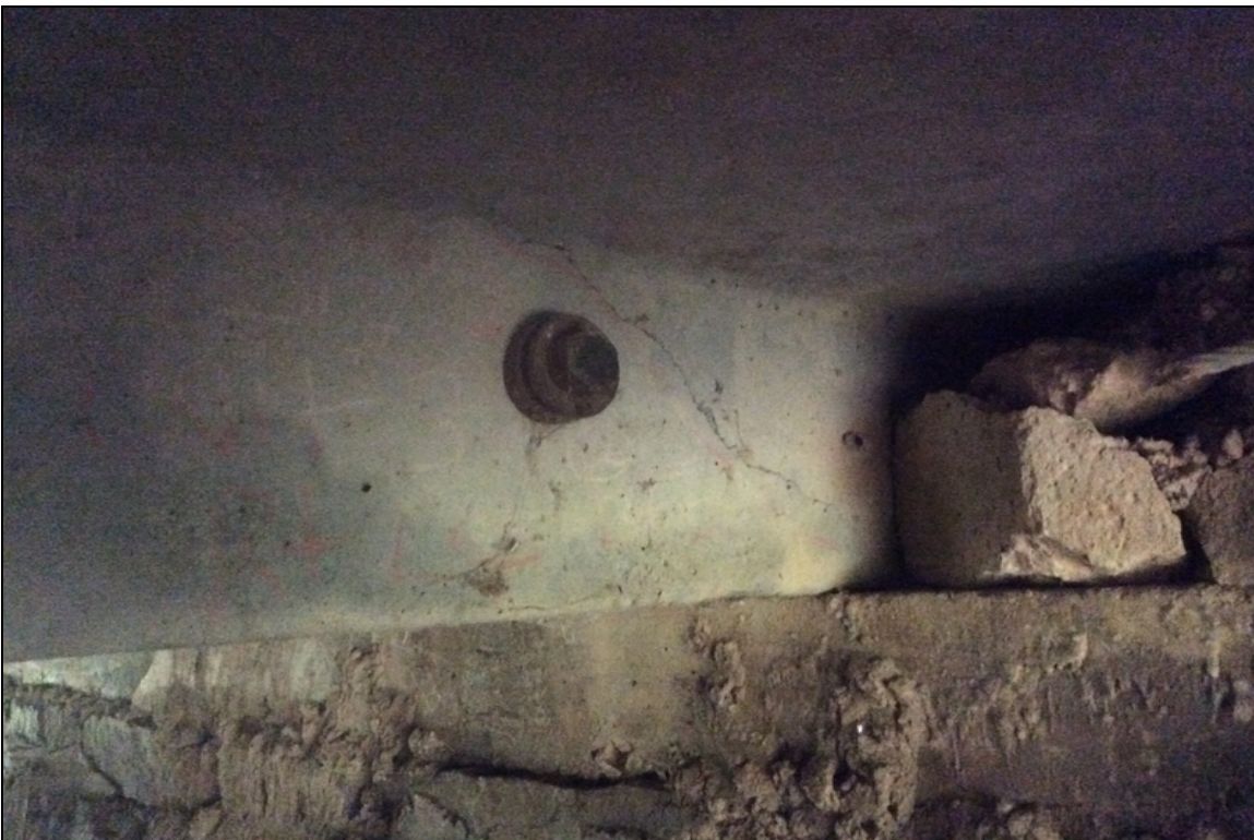
Bent # 2 Span # 2 Unit # 3 Lt & Rt stems have shear cracks.
