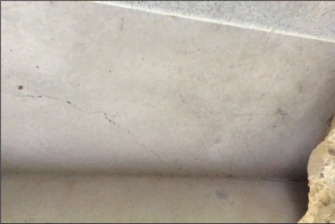
Span # 1 Unit # 2 cracks on the undersurface of the deck.
