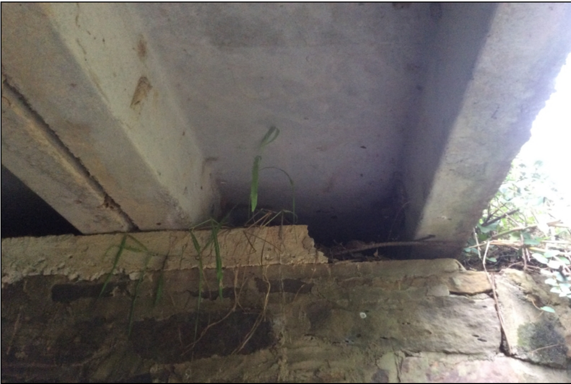
Bent # 1 Unit # 1 missing section of the cap.
