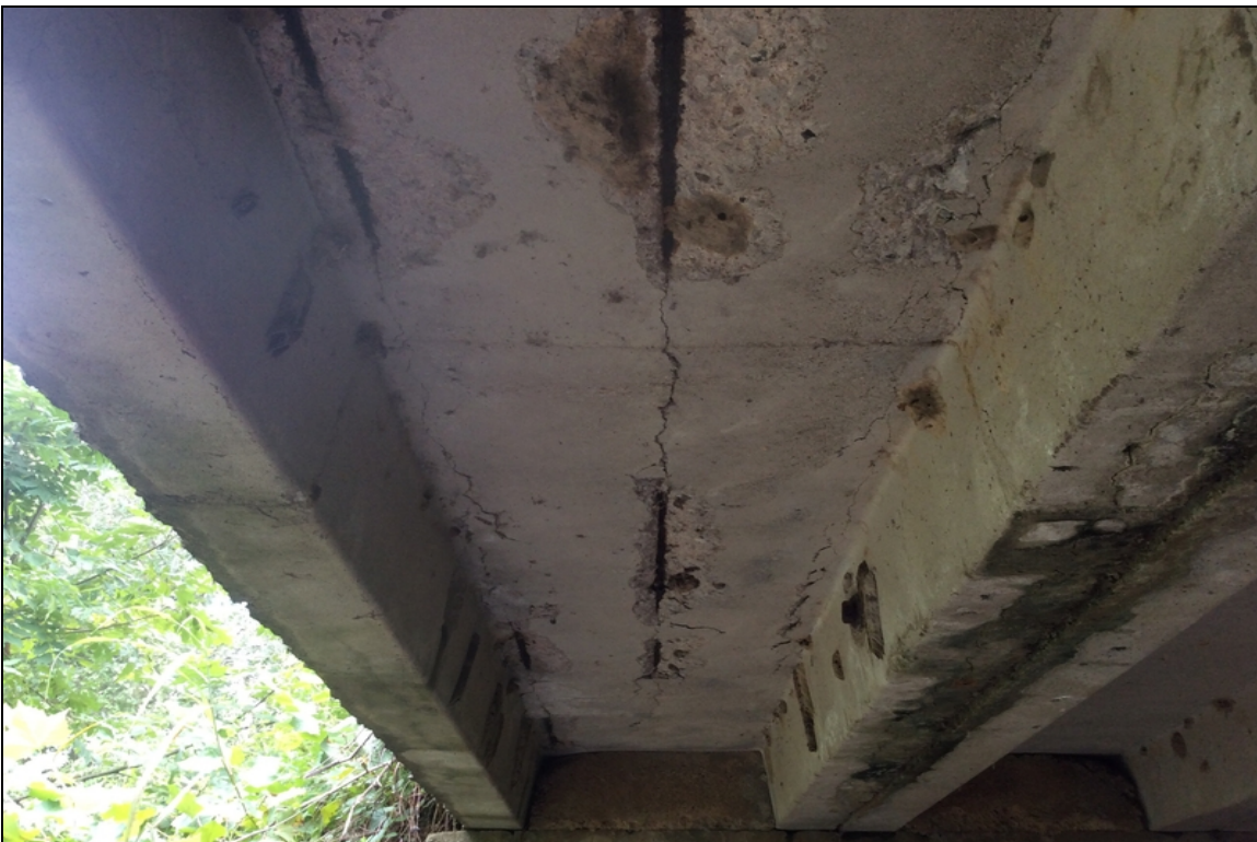
Span # 1 Unit # 8 spalling with exposed reinforcing steel on the undersurface of the deck.
