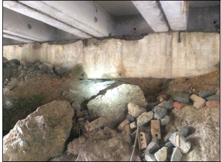
Abutment 1 scour under cap at mid span
