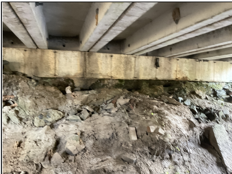
Bent 2 erosion.
