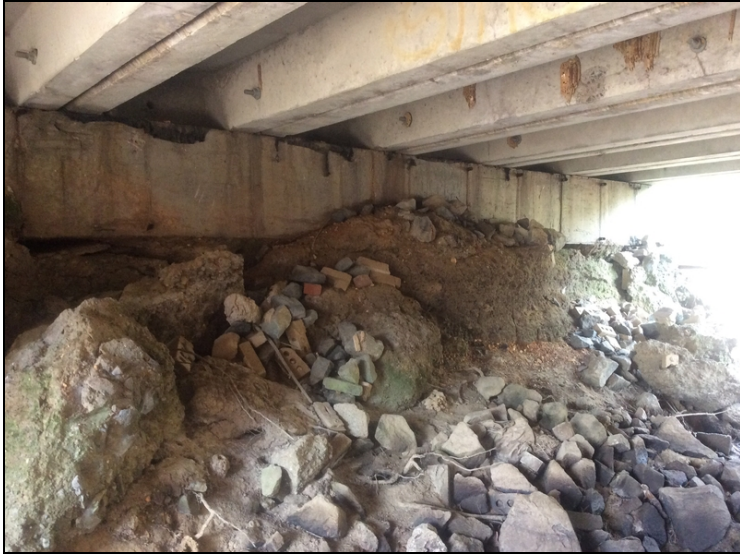
Endslope - Bent 1: Erosion/scouring
