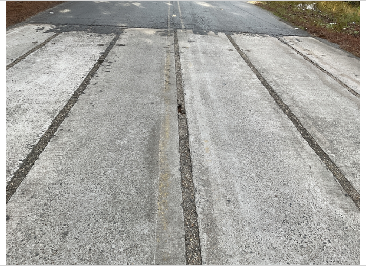
Span 1 girders 4 & 5 grout missing in keyways.
