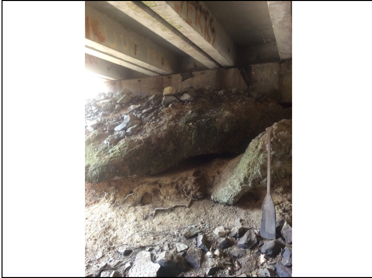
Endslope - Bent 1: Erosion (minimum 8' hole under abutment cap)
