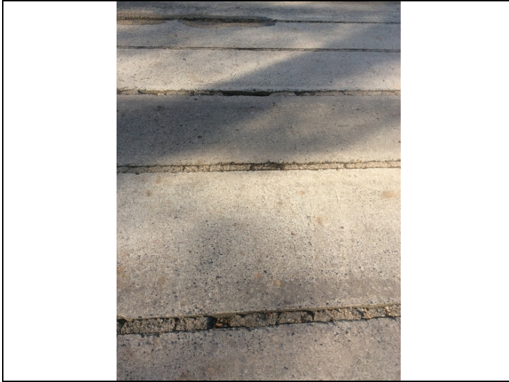
Deck - Span 2 Units 2-7: Grout deterioration
