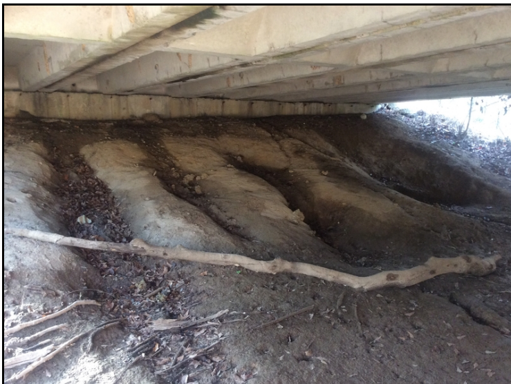
Endslope - Bent 3: Erosion
