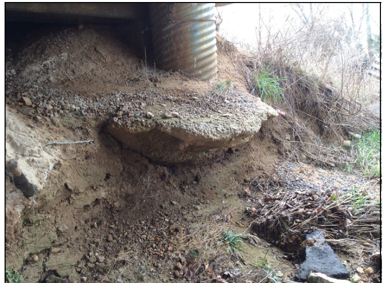
Scour and undermining at footings at Column 3 @ Bent 2.
