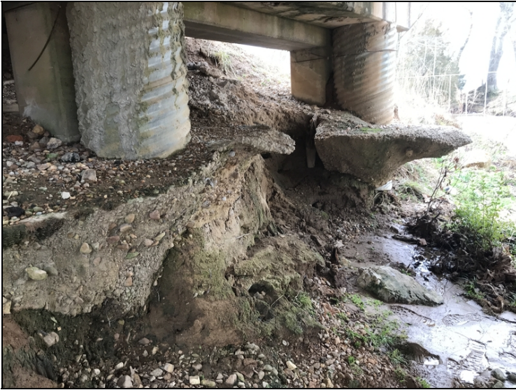
Scour at Columns 2 & 3 footing at Bent 2. Footing is undermined.
