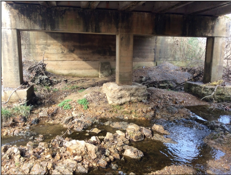
Scour 1.5' to 2' below top of footings at Bent 1.
