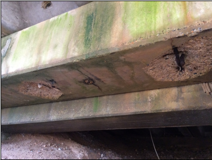
Cracks / spalls with rebar exposed to cap @ Bent 2.
