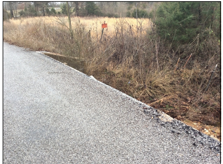
Bridge rail is missing on Right side.
