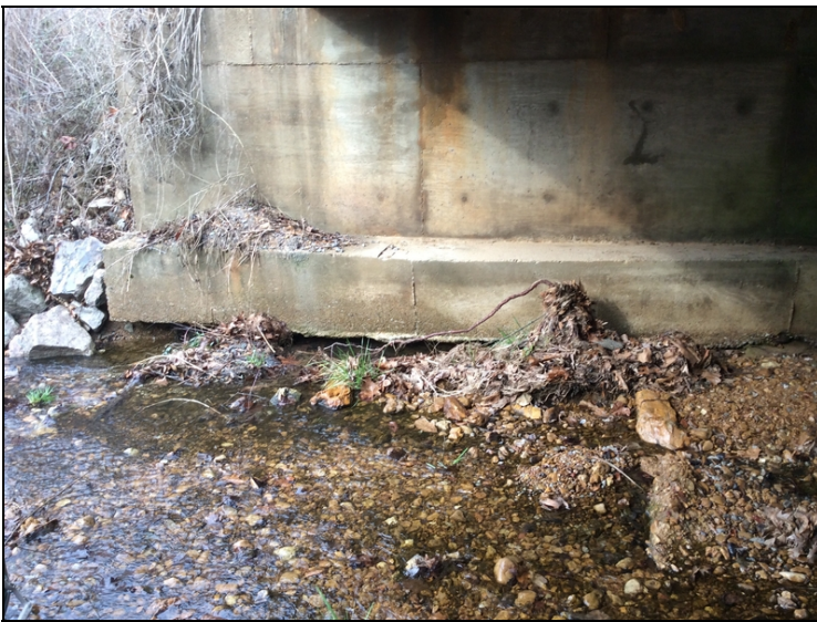
Scoured 1' below bottom of footing & 2' back under @ Abutment 1.
