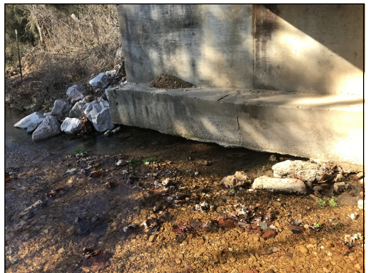
Abutment 1 Scoured 1' below bottom of footing & 2' back under.
