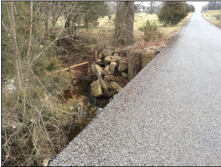
Bridge rail is missing on Left side.
