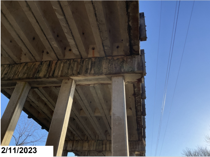
Delam on left side of bent 9, span 10 side.
