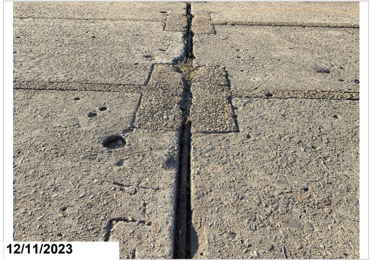
Loss of joint material
