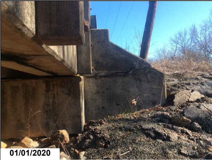
Abutment wing wall crack left side of beginning of bridge
