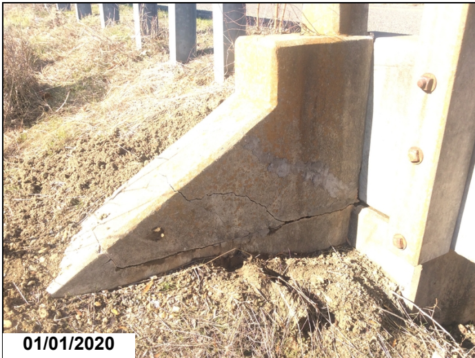
Abutment wing wall left side cracks
