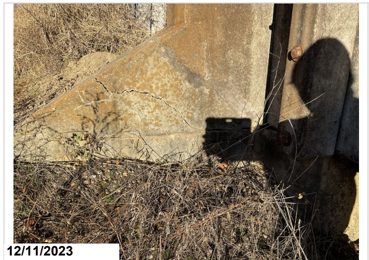
End of bridge left side cracking on abutment wing
