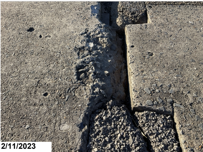
Spalls on edges of precast units
