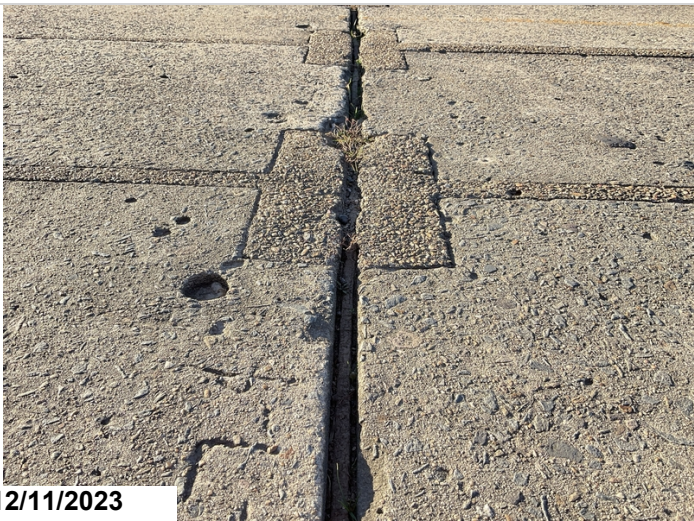
Loss of joint material
