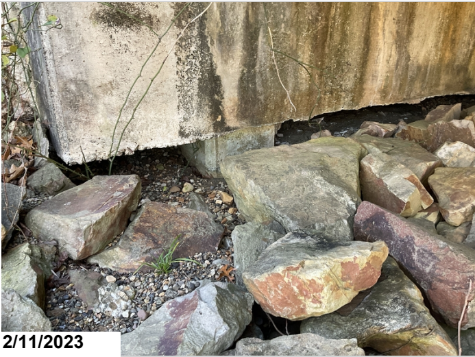
Pile exposed right side of abutment 1
