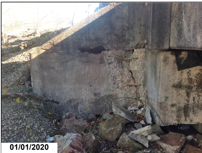
Abutment wing wall cracked and exposed rebar right side beginning of bridge
