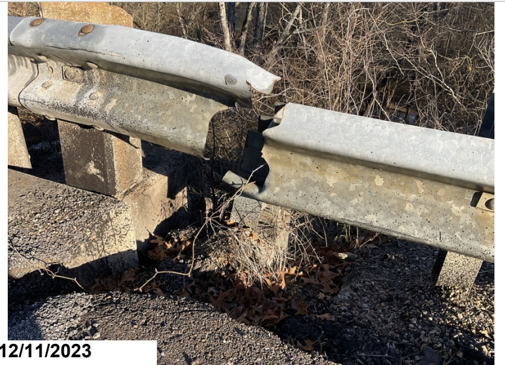
Beginning of bridge right side damage
