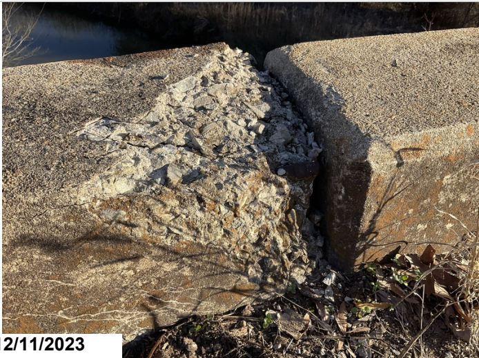
Spall with rebar exposed on right side of concrete bridge railing in span 7
