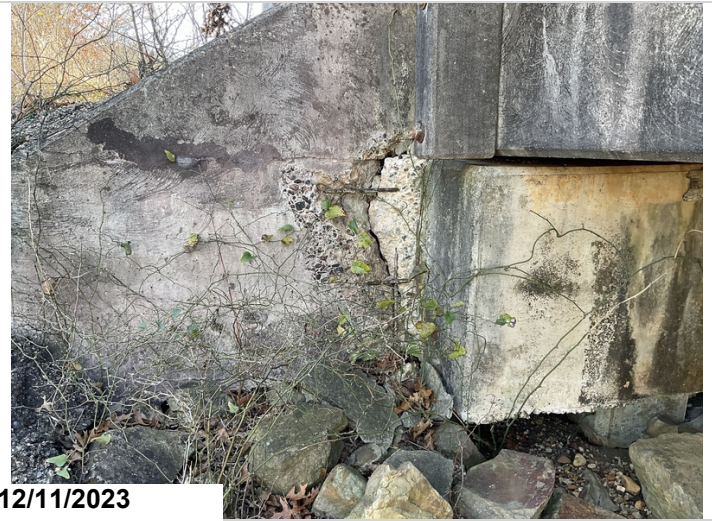
Spalling with rebar exposed to right side of bent 1 abutment wing
