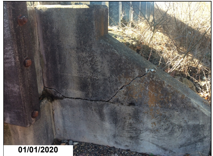
Right side end of bridge abutment wing wall cracks
