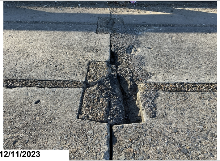
Spalls on edges of precast units
