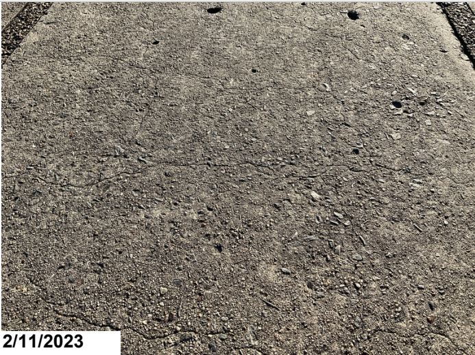
Cracking in units
