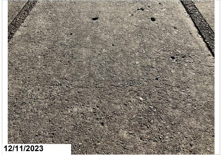
Sealable deck cracking in all spans
