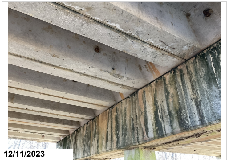
Minor spalling on various precast units
