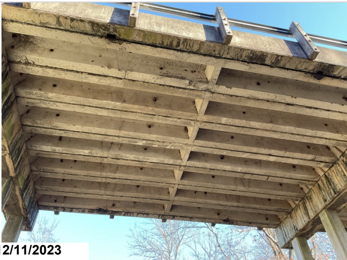
Minor spalling on various precast units. Span 3
