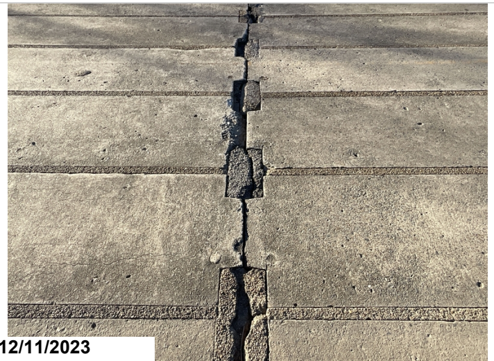
Spalls on edges of precast units
