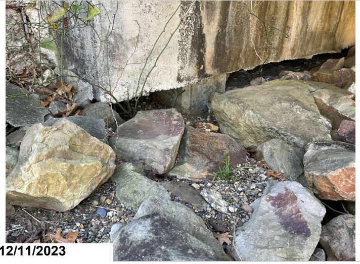
Pile exposed right side of abutment 1
