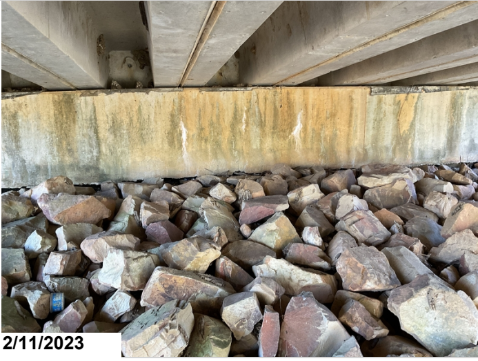
Cracking with Efflorescence in abutment 1
