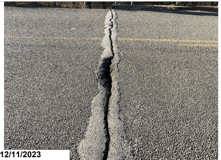
Large cracking in asphalt at beginning of bridge
