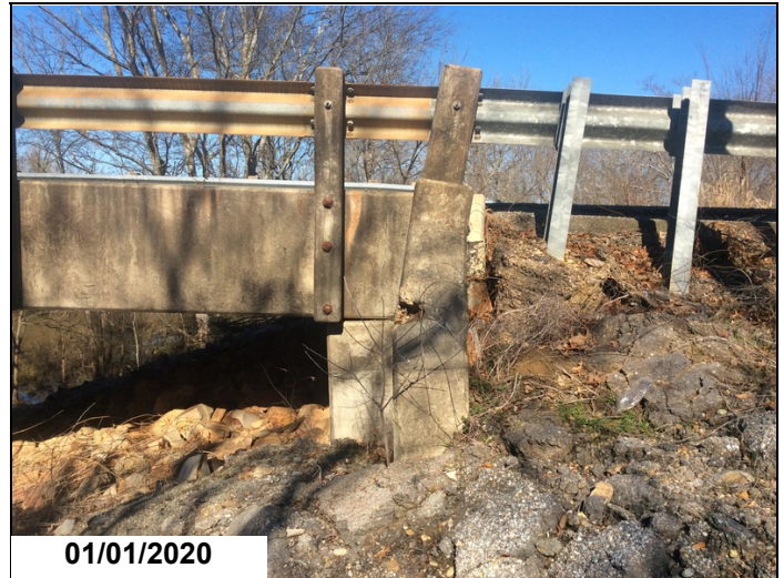
Left side beginning of bridge wing leaning also cap leaning in opposite direction
