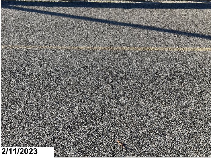
Cracking in asphalt wearing surface in span 1
