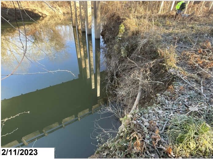
Scour to bank around bent 6
