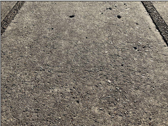
Sealable deck cracking in all spans
