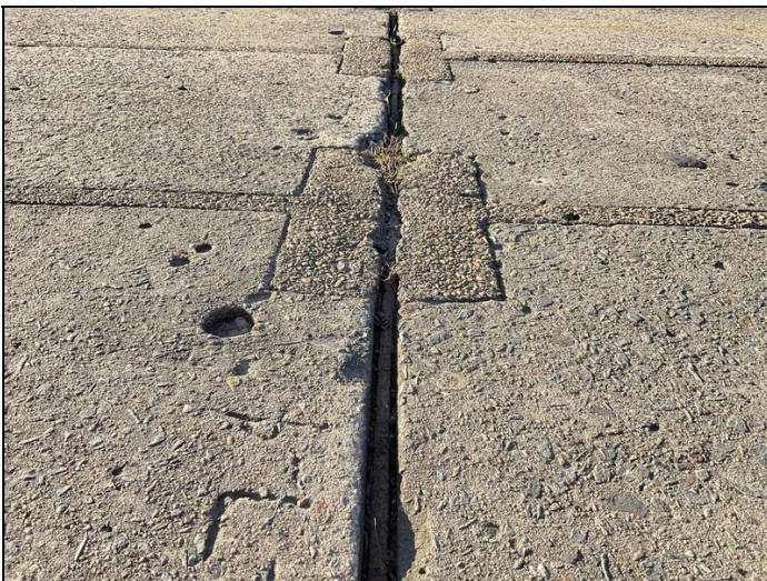
Loss of joint material
