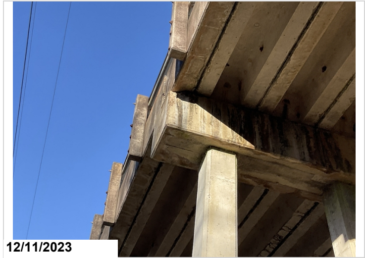
Spall on left side of bent 5 cap
