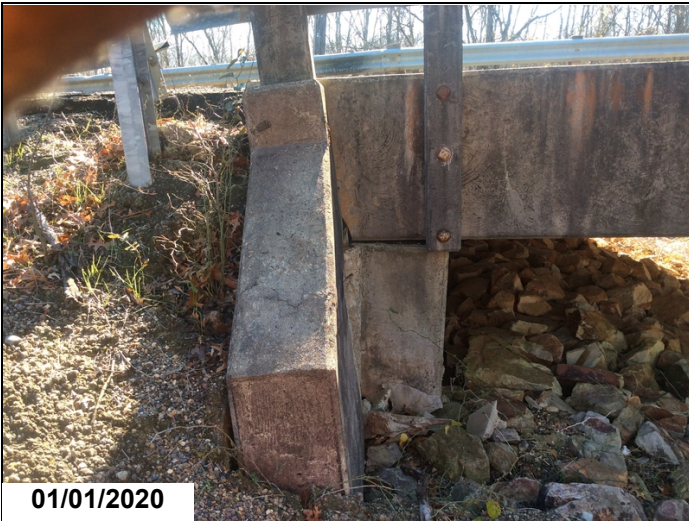
Right side beginning of bridge wing wall leaning and cap leaning opposite direction
