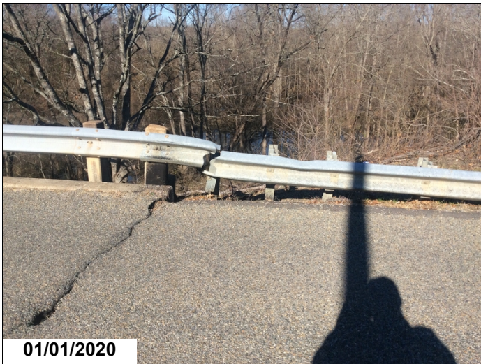
Guard rail busted right side beginning of bridge
