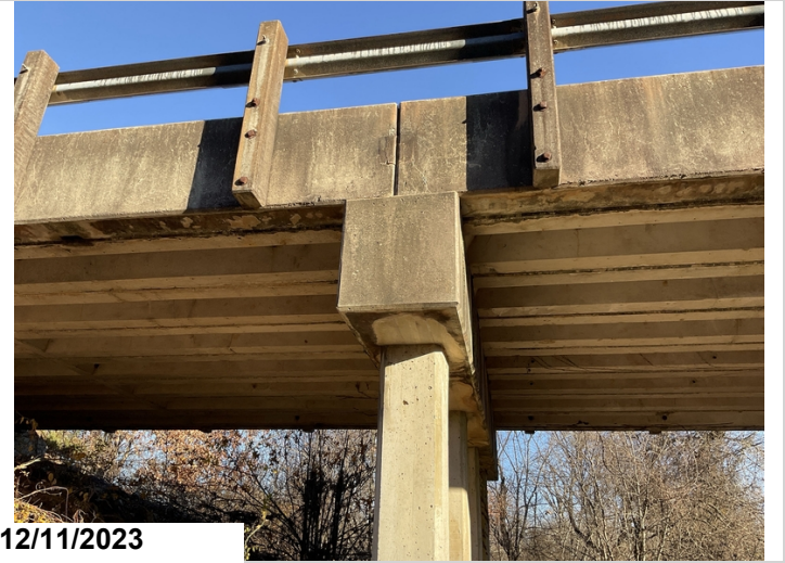
Delam and cracking with efflorescence above bent 11. Both sides have cracking with efflorescence
