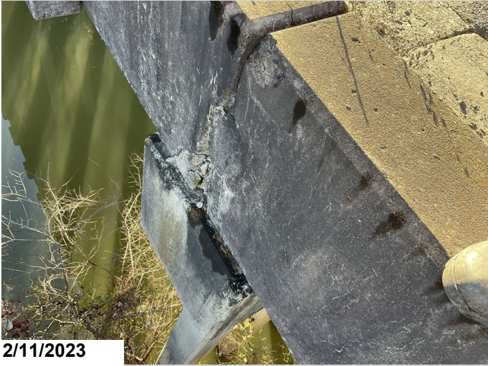
Spalling on right and left sides of bent 6
