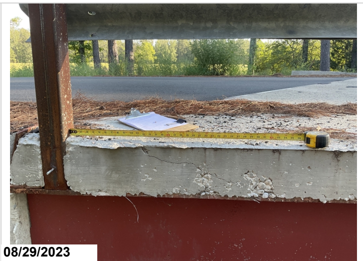
Deck at bent 2: delam to the deck.
