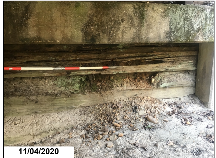
Bent 1 timber cribbing has severe decay allowing embankment to spill through.
