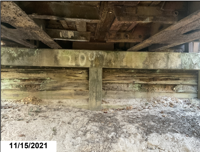
Bent 1, the timber cribbing has severe decay. Embankment is beginning to spill through the decayed cribbing.
