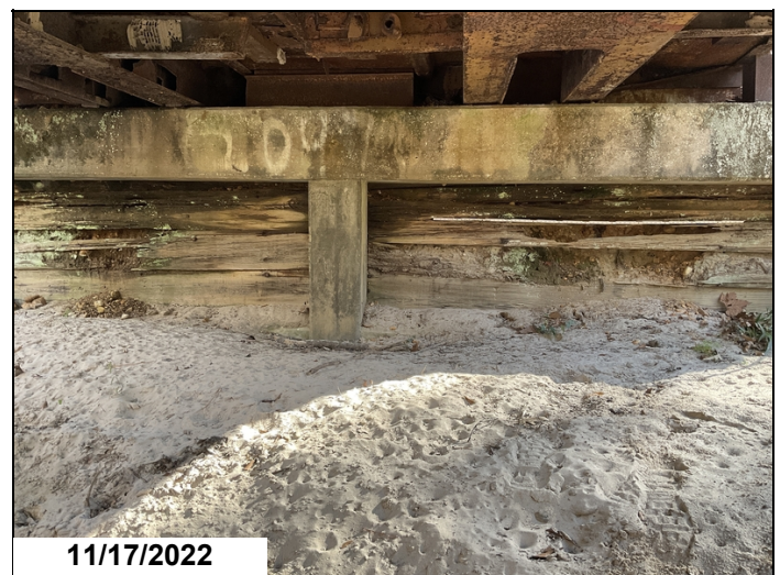
Bent 1: timber cribbing has rotted to where backfill is spilling through 2022
