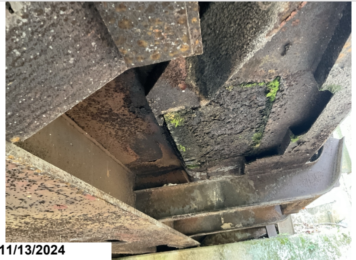
Left car 10' away from bent 1, active corrosion with section loss.
