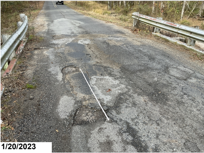
Multiple pot holes in the asphalt overlay
