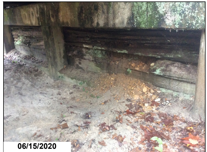
Bent 1 timber cribbing, severe decay allowing embankment to spill through.
