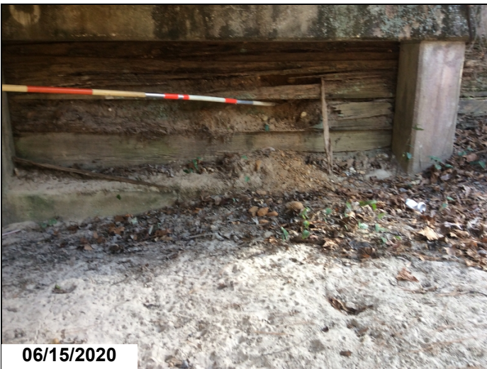
Bent 1 timber cribbing has severe decay.
