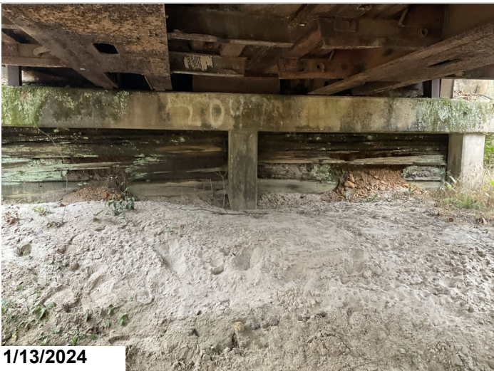
Bent 1, timber cribbing: severe decay allowing embankment to spill through. 2024
