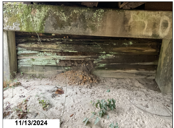
Bent 1: timber cribbing has rotted to where backfill is spilling through 2024
