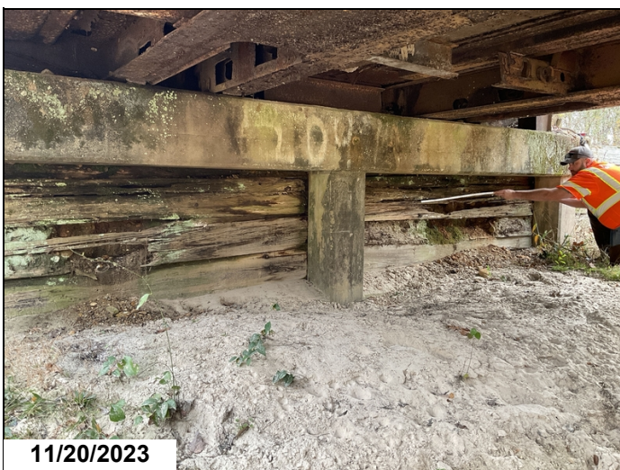
Bent 2, timber cribbing: severe decay allowing embankment to spill through. 2023
