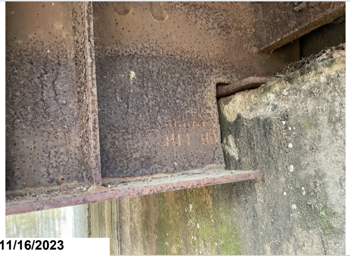
Bent 1, left car: both left and right car center sills are notched to fit the abutment. Special attention was these coped areas.
