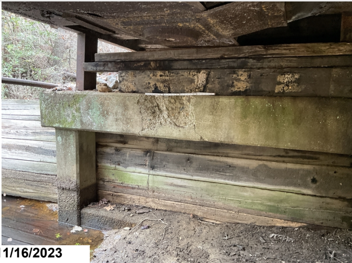
Bent 6: spall in cap under the left car. 2023
