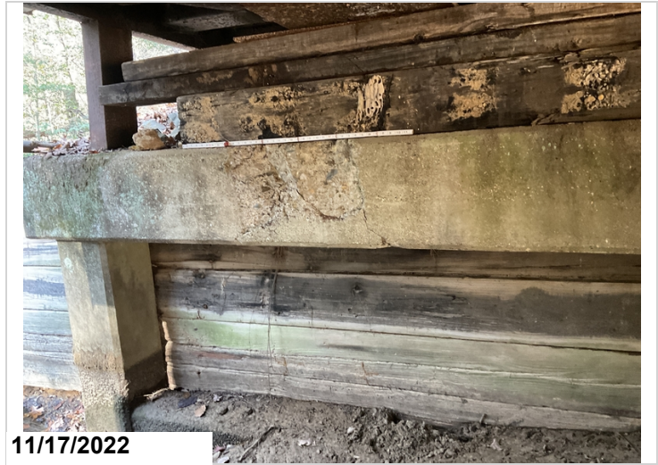
Bent 6: Spall to face of cap between columns 1&2.
