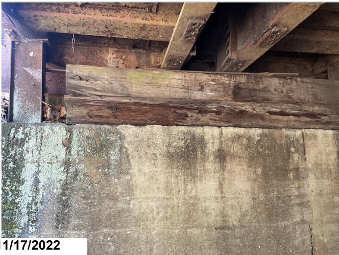
Bent 1: Timber cribbing beginning to have some rot on the end
