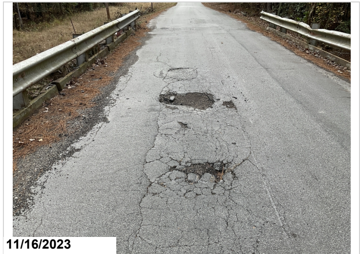
Pot holes in the asphalt wearing surface on the east side
