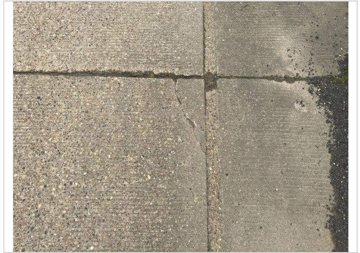
Span 1 unit 6 has crack in the ahead right corner common span 2.
