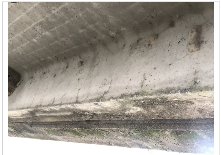
Span 2 unit 1 left leg has flexure cracks.
