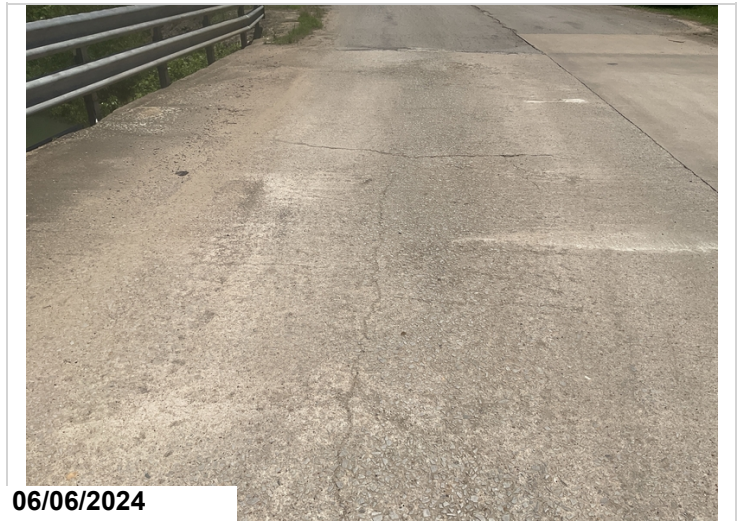
Full depth transverse and longitudinal cracks in the original portion of the deck (right side). CS2
