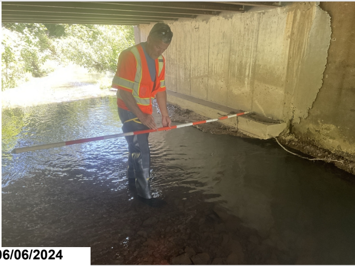
Bent # 2, back: the footing has an area of full depth undermining to the new portion of pier wall left of centerline that extends approximately 6' in length at this inspection.
