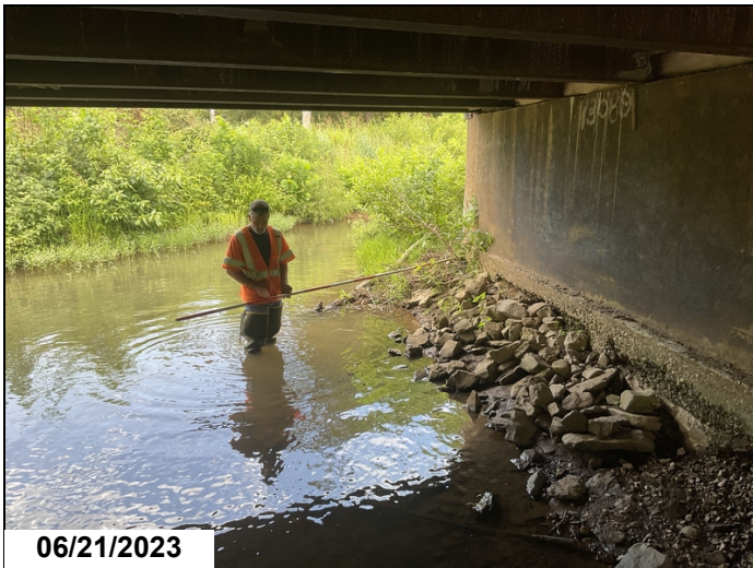
Abutment # 1 Rt undermine scale.
