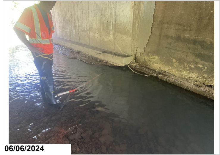
Bent # 2, back: the footing has an area of full depth undermining to the new portion of pier wall left of centerline that extends approximately 6' in length at this inspection.
