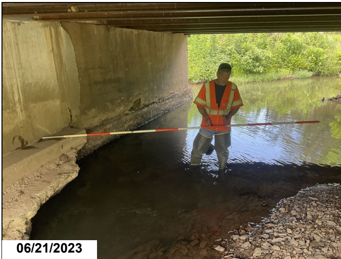
Bent # 2 backface undermine scale.
