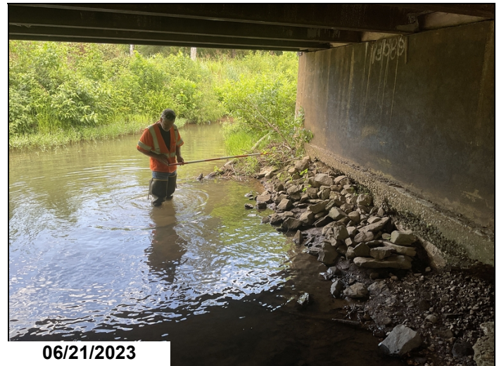
Abutment # 1 Rt wing wall undermining.
