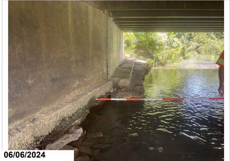
Abutment # 1, right: The Rt footing has concrete deterioration with a 6" void adjacent to the centerline construction joint.
