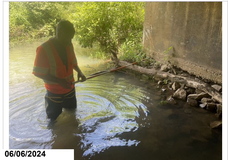
Abutment # 1, right: The Rt footing has concrete deterioration with a 3' void adjacent to the right wing wall.
