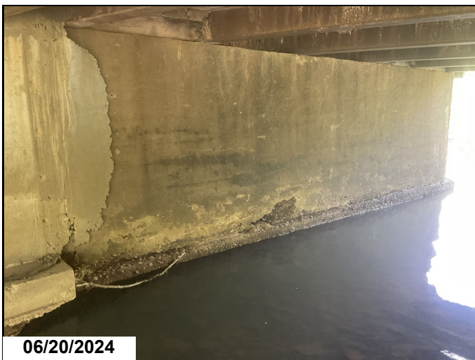
Bent # 2 backface has a 24" area concrete deterioration with approximately 4" of concrete section loss located approximately 8' Rt of centerline.
