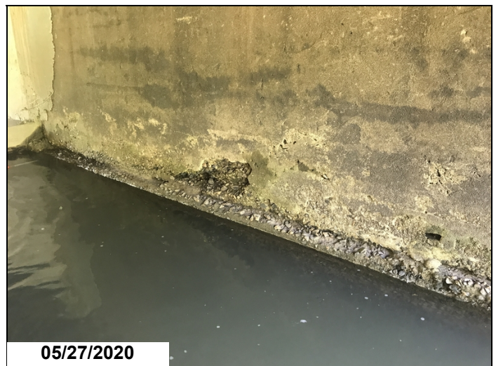
The bases of the bent walls and the footings in the original portion of structure (Right side) have soft deteriorated concrete with concrete section loss. The substructure appears to be founded on creek gravel and soil with voids that penetrate under the footings.
