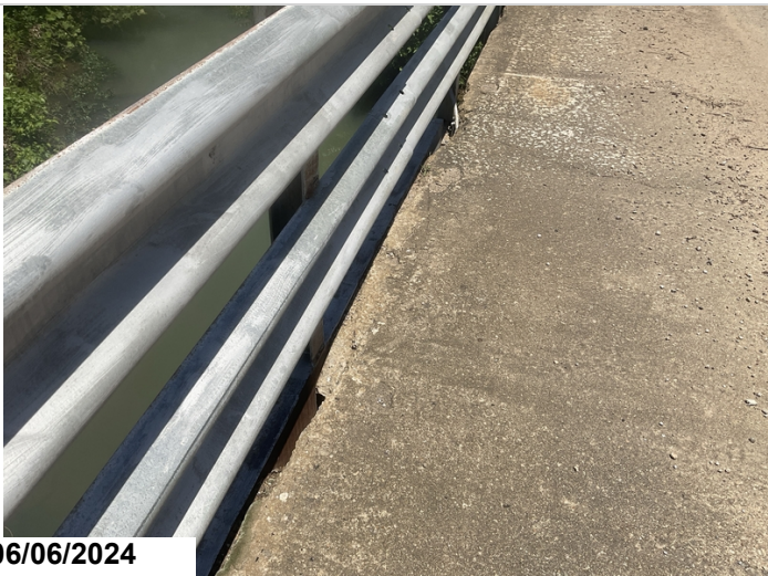
Span # 2, right: the edge of the deck in span # 2 has several spalls that are partially concealed by a steel channel where the bridge rail posts are attached to the deck.
