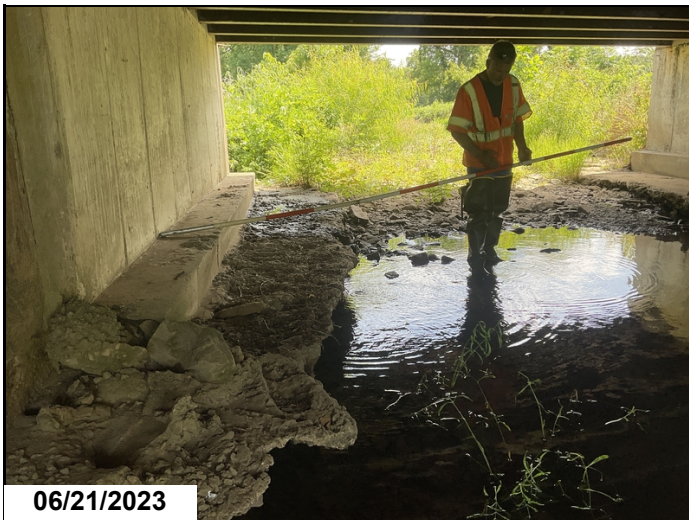
Bent # 2 aheadface undermine scale.
