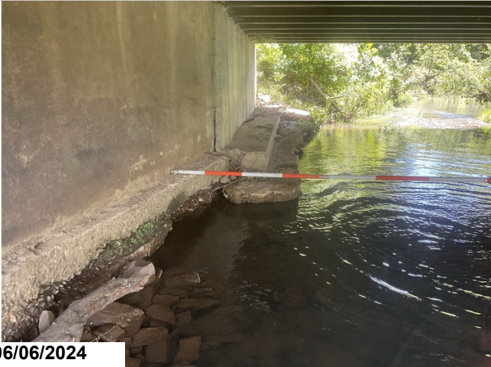
Abutment # 1, right: The Rt footing has concrete deterioration with a 6" void adjacent to the centerline construction joint.
