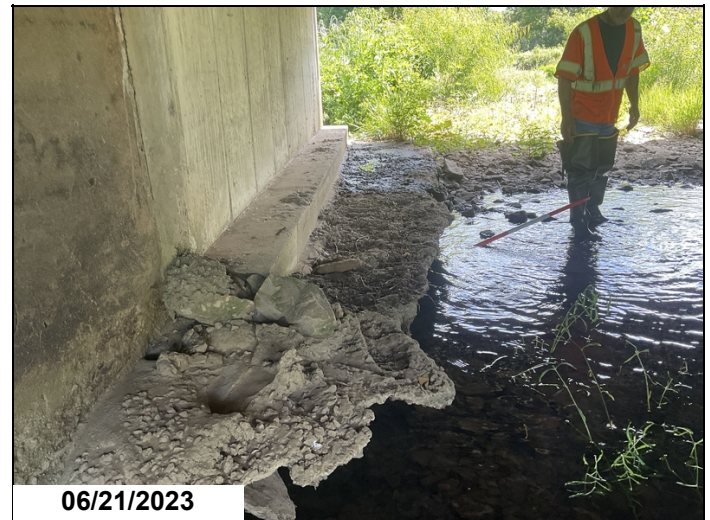
Bent # 2 aheadface undermine.
