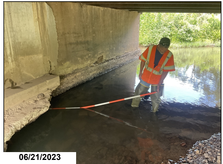
Bent # 2 backface undermine.
