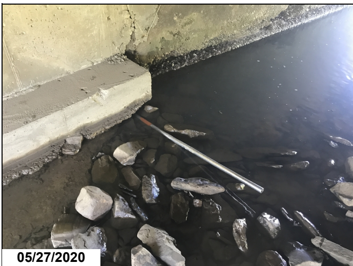
Bent 2 footing, span 1-Void under footing.
