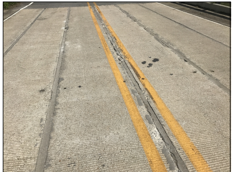
Typical grout missing at beam 3 - 5 joints.
