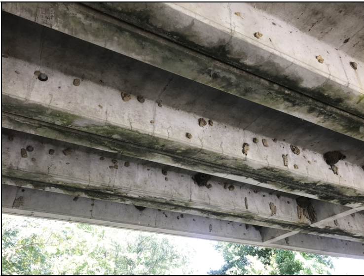
Typical cracking in legs of beams.
