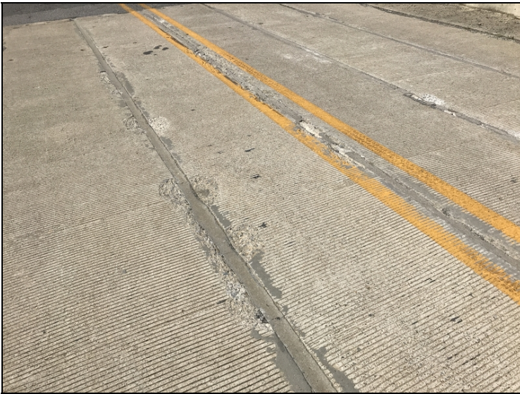
Typical spalling at beam joints.
