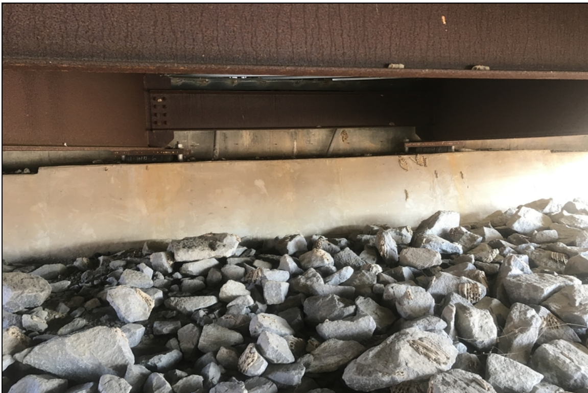
Bent 1 has cracks with efflorescence.
