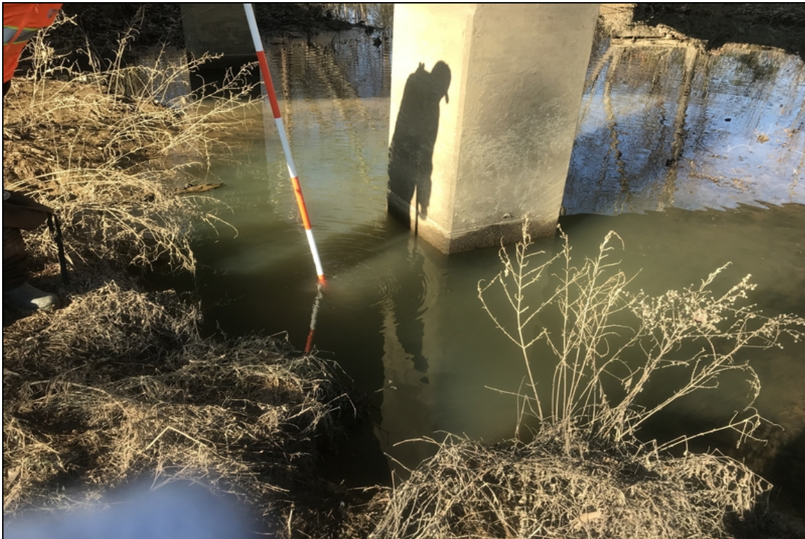
Bent 3 both columns have minor local scour.
