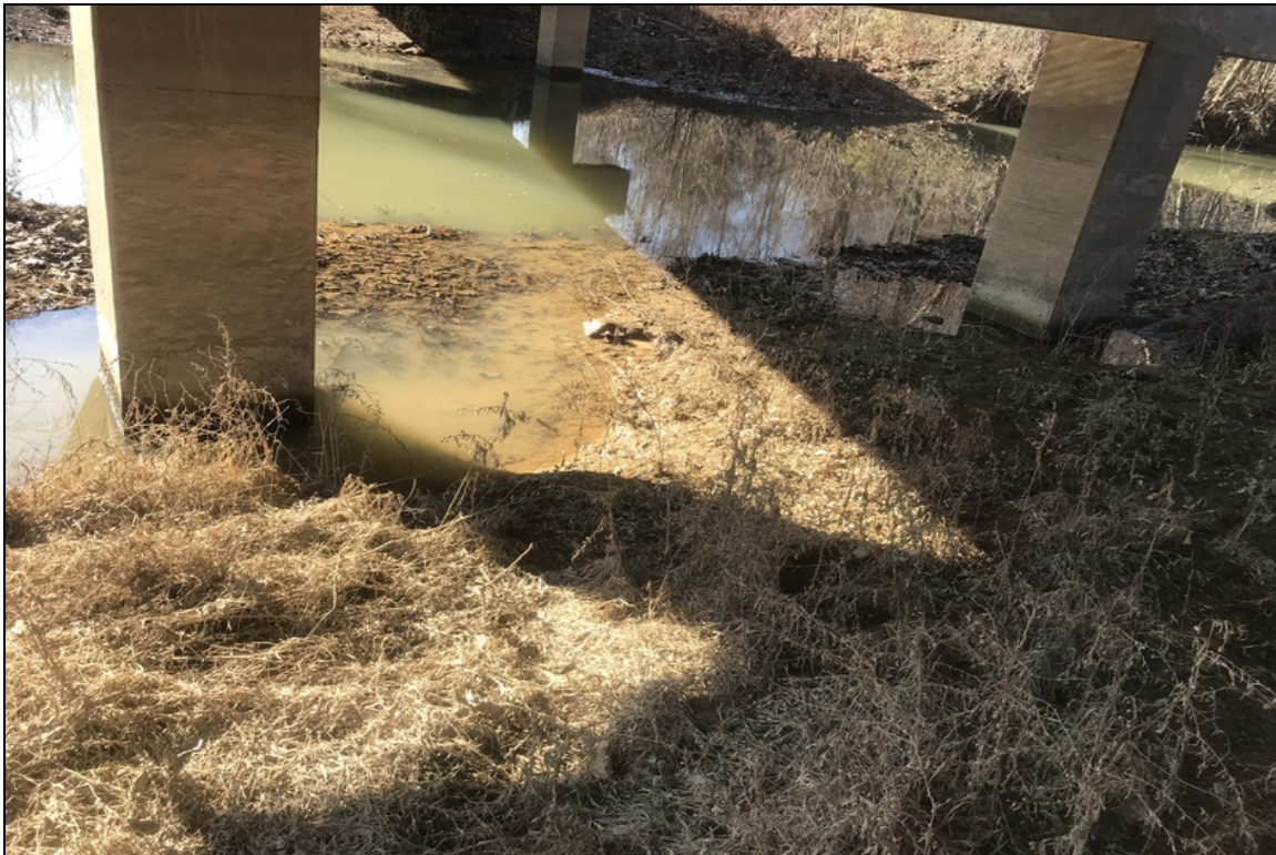
Bent 2 both columns have minor scour.
