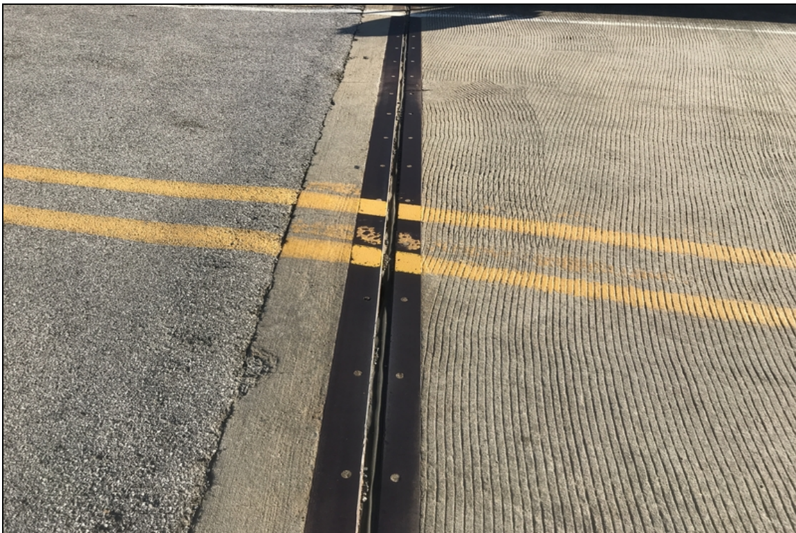
Bent 1 pourable joint has 6' of holes.
