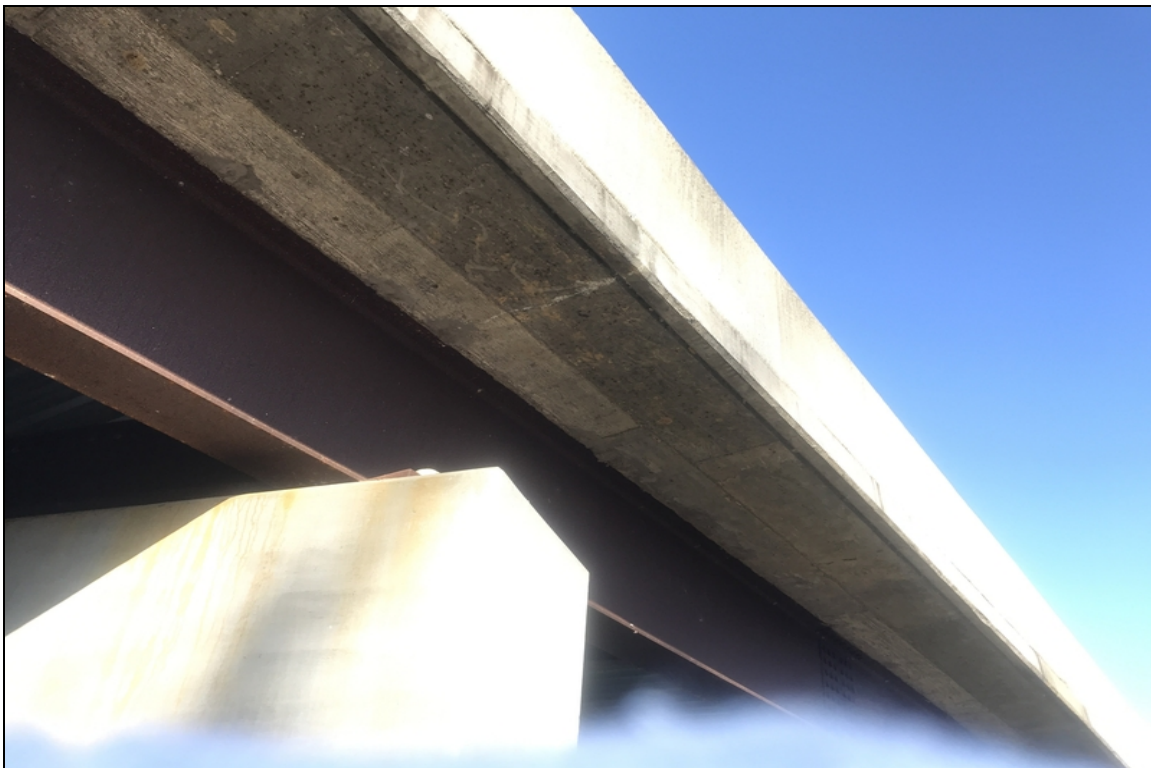
Overhangs have cracks with efflorescence.
