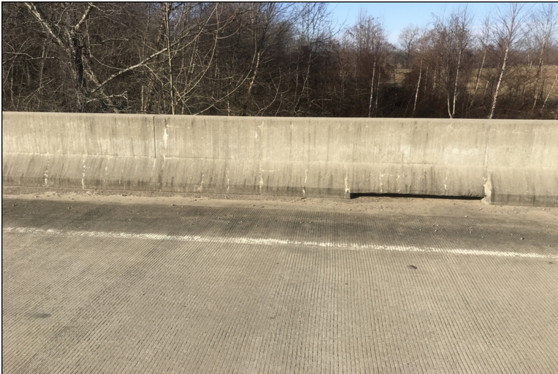
Concrete bridge rail has vertical cracks scattered throughout.
