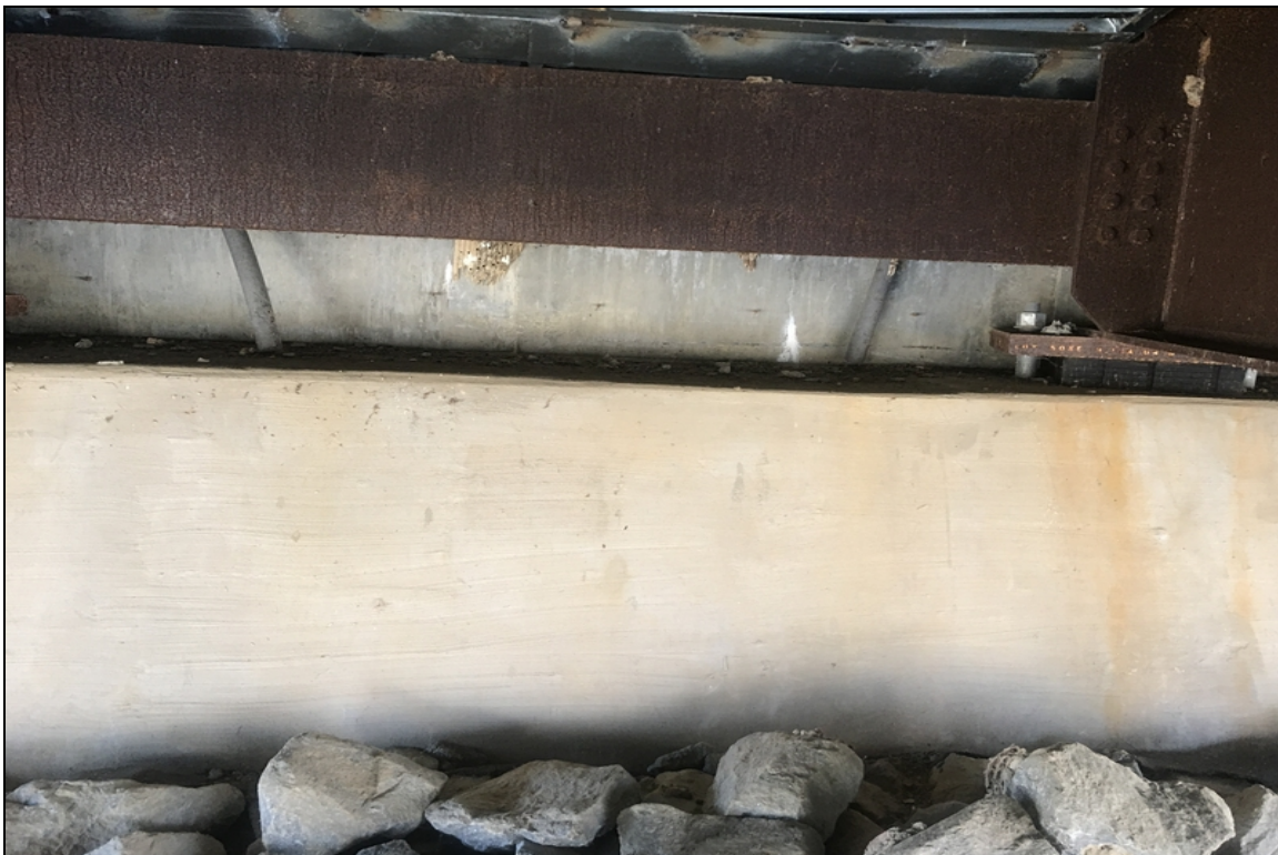
Bent 4 has cracks with efflorescence.
