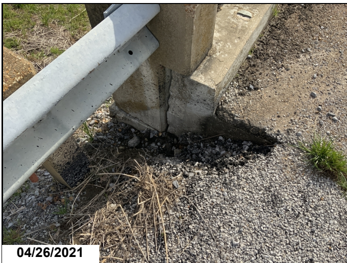
Abutment #1 left approach shoulder eroded.
