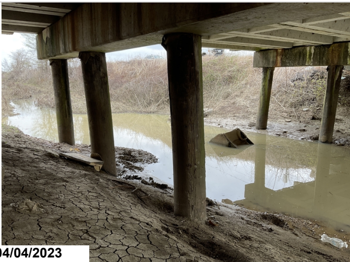
Bent #2 piles #1,3 are split by drift pin, and pile #3 is also sounds moderately hollow.
