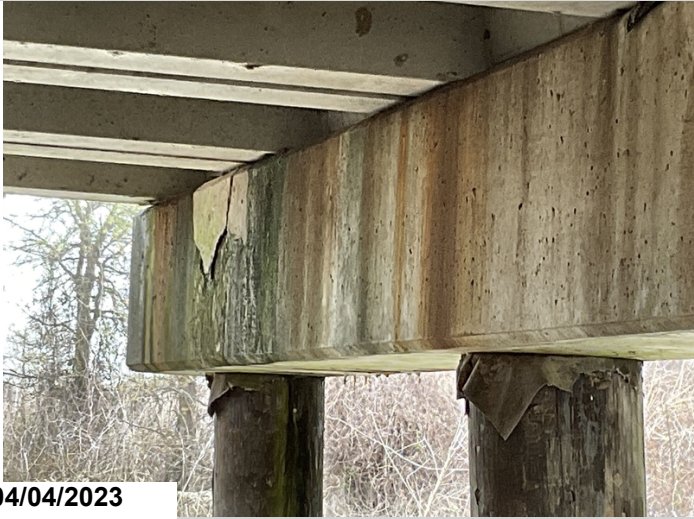
Bent #2 cap back face has a 2' delamination under unit #1 right leg.
