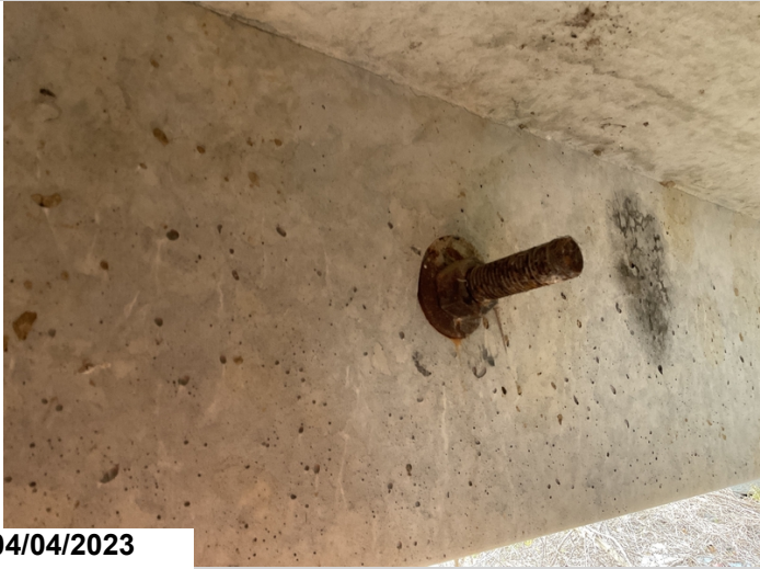
Typical corroded connection bolt
