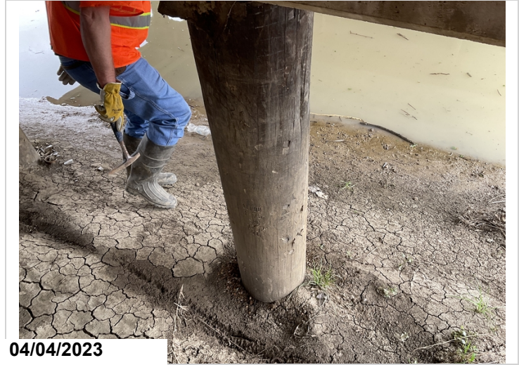
All piles are weathered and have minor vertical cracks.
