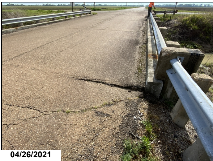
Abutment #1 roadway settlement, right side.
