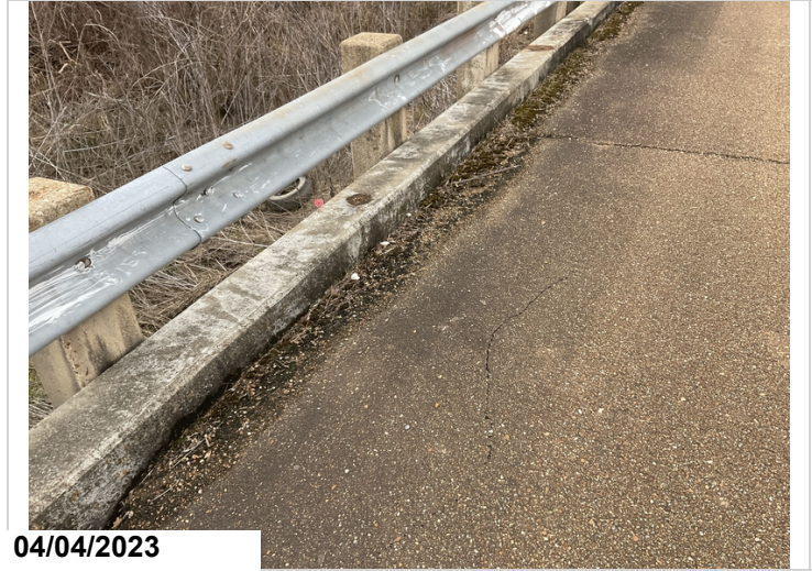
Typical debris in gutters
