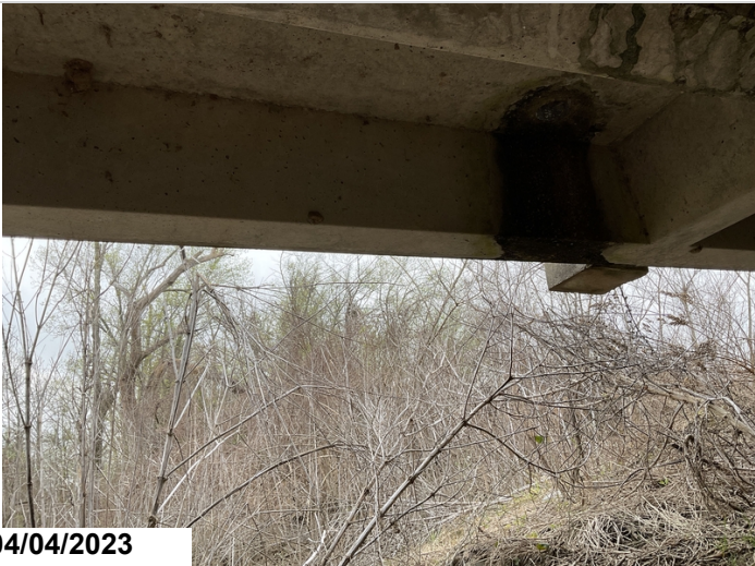
All units at drains have light to moderate abrasion for 1'.
