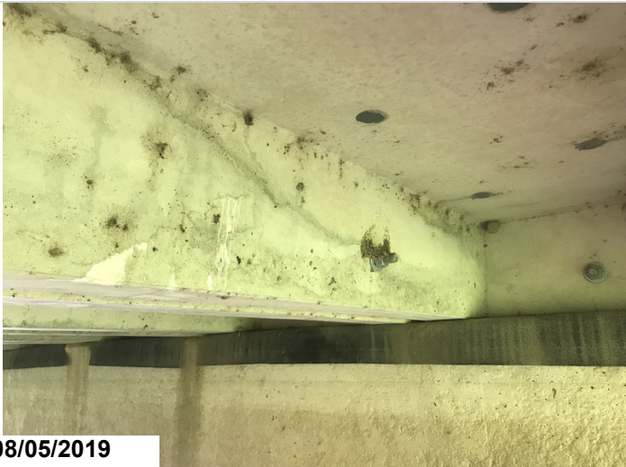
Typical diagonal cracks
