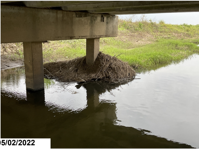
Bent 2 has minor drift buildup.
