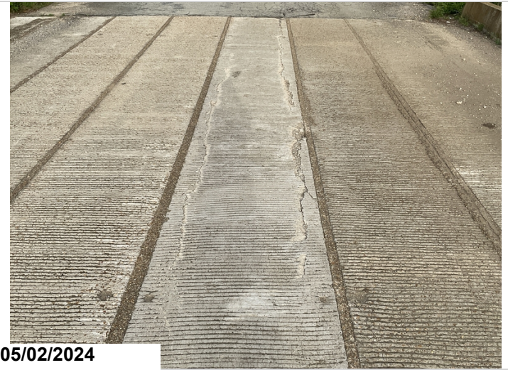
Span 2 unit 5 top flange delaminated areas
