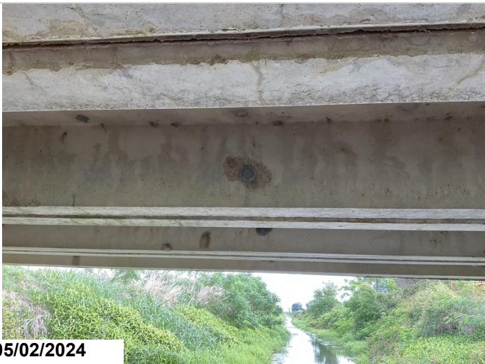
Span 2 unit 6 spall at transverse bolt connection (typical).
