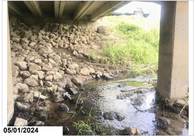
Span 2 right side has some embankment erosion and rip rap displacement
