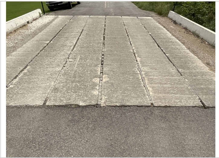
Shear key grout
