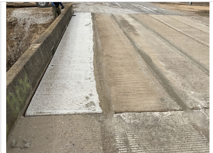
Span 2 unit 1 NEW Span 2 unit 2 was moved from unit 1 position
