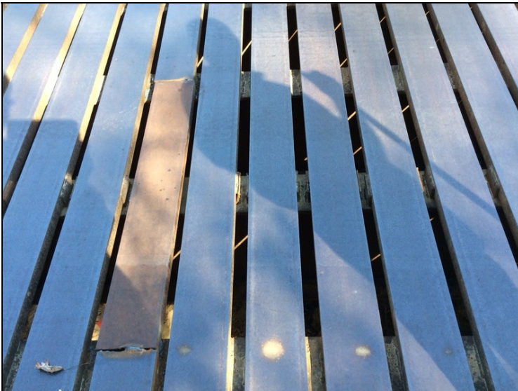
Several cracked welds at steel deck channels
