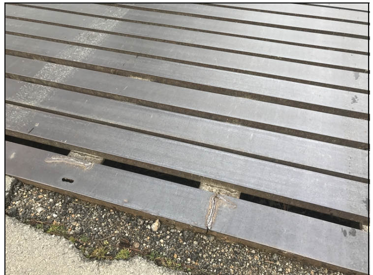
Cracked channels
