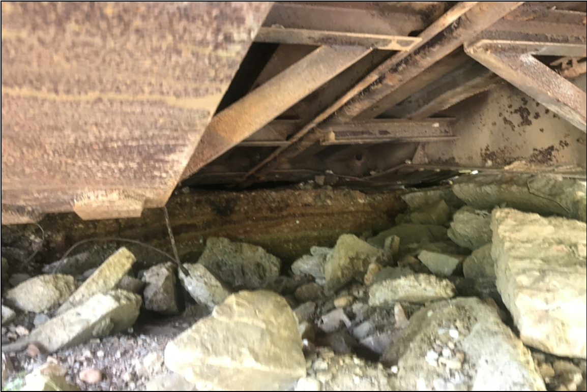
Scour at abutment 2 approx. 10' from end of bridge
