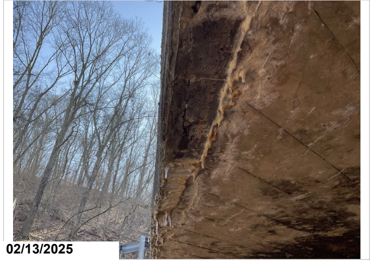
Barrel 2, Right: Cracking with efflorescence with build up.
