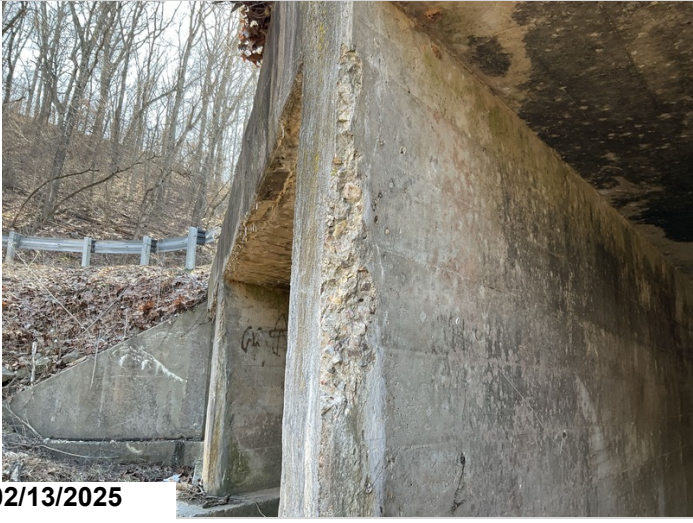
Barrel 2 & 3, Intermediate Wall: Spalling.
