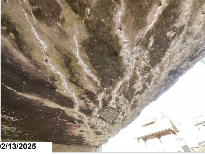
Barrel 1, Right: Cracking with efflorescence with build up.
