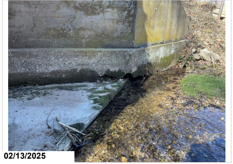
Barrel 3, Back Wall, Footing: Spalling.
