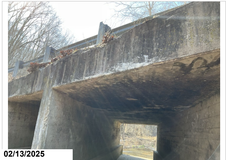
Barrel 3, Right: Cracking with efflorescence.
