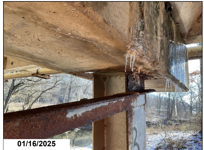
Bent 2, Pile 4: Active corrosion with flaking rust.
