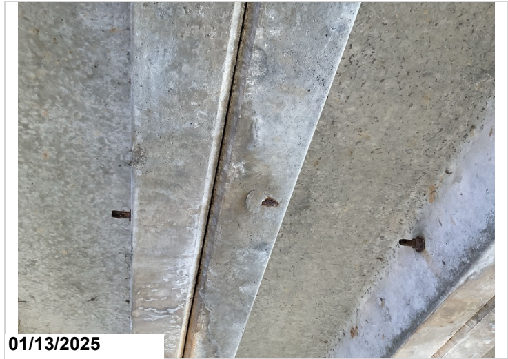
Span 2, Channel 4, Left Leg: Spalling with exposed reinforcing steel with section loss.
