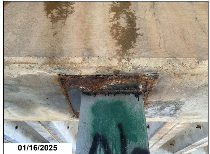
Bent 1, Pile 2 & 4: Minor active corrosion.
