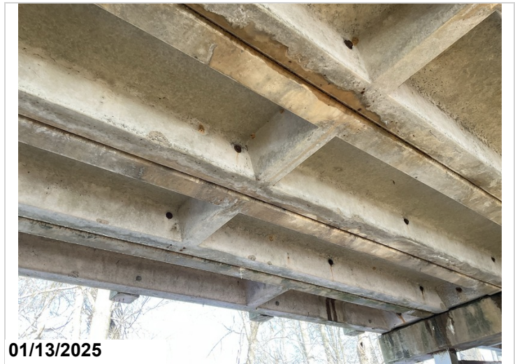
Span 8, Channels 1, 3, 5, 6 & 7: Minor spalling.
