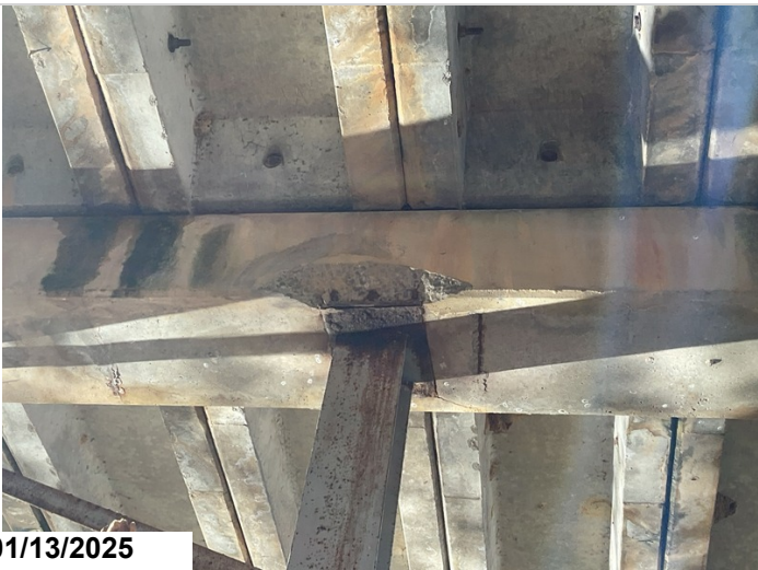
Bent 4, Pile 3, Ahead: Spalling with exposed reinforcing steel with section loss.
