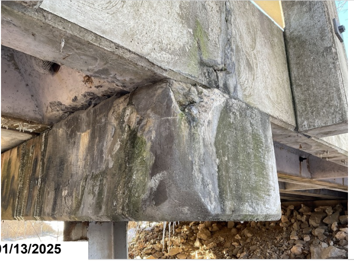
Bent 1, Left: Spalling.
