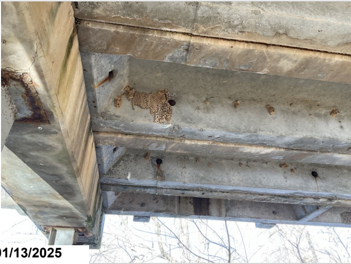
Span 6, Channels 1 - 6: Spalling.
