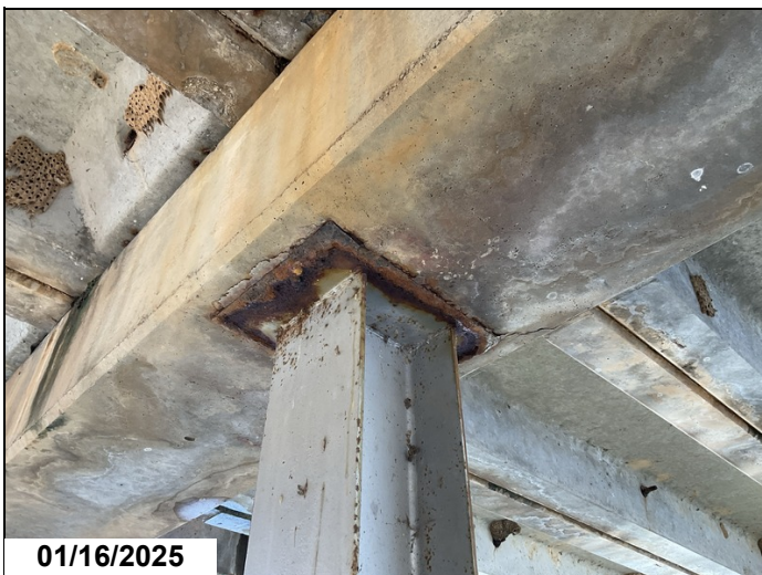
Bent 5, Piles 1 - 4: Active corrosion with flaking rust.
