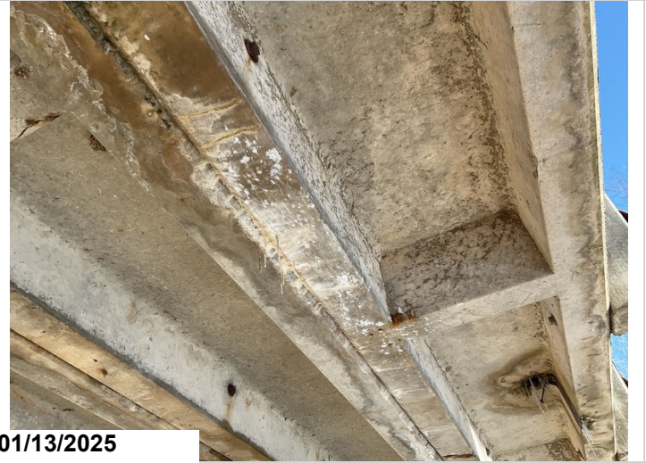
Span 3, Channel 8, Left Leg: Longitudinal cracking with efflorescence with build up.
