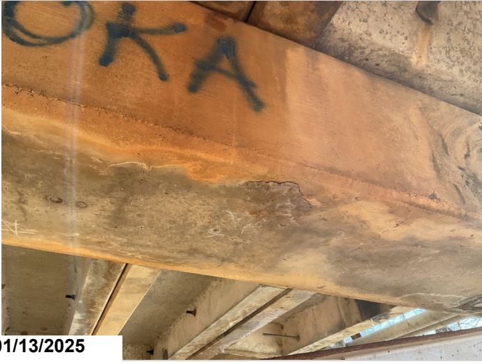
Bent 1, Right: Delam.
