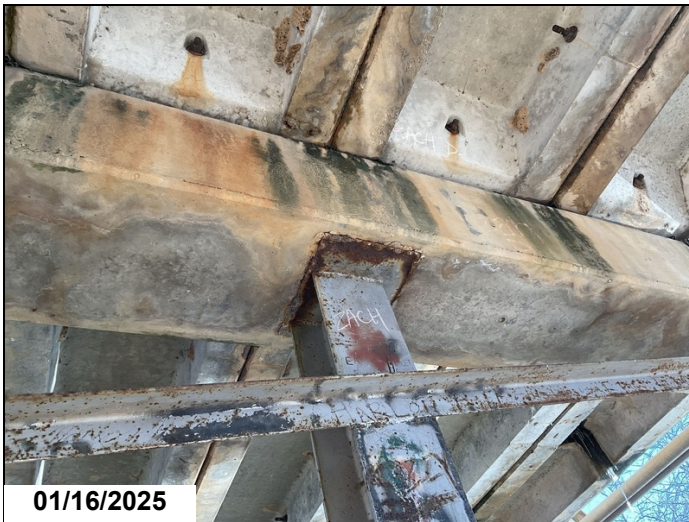
Bent 3, Piles 1 - 4: Minor active corrosion.
