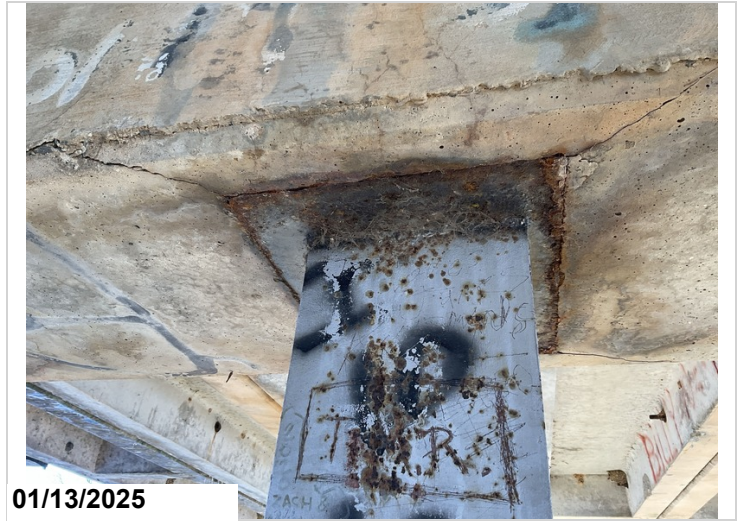
Bent 2, Piles 1 - 3: Minor active corrosion.
