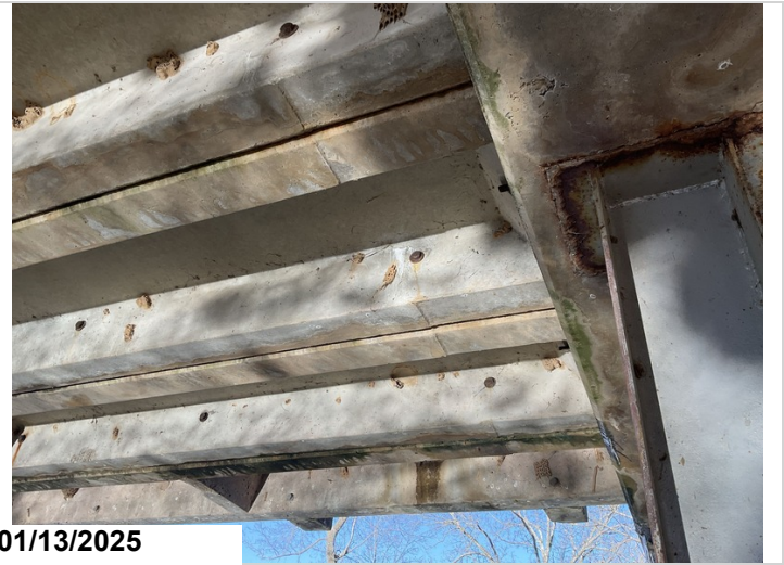
Span 5, Channel 2: Cracking with efflorescence with build up.
