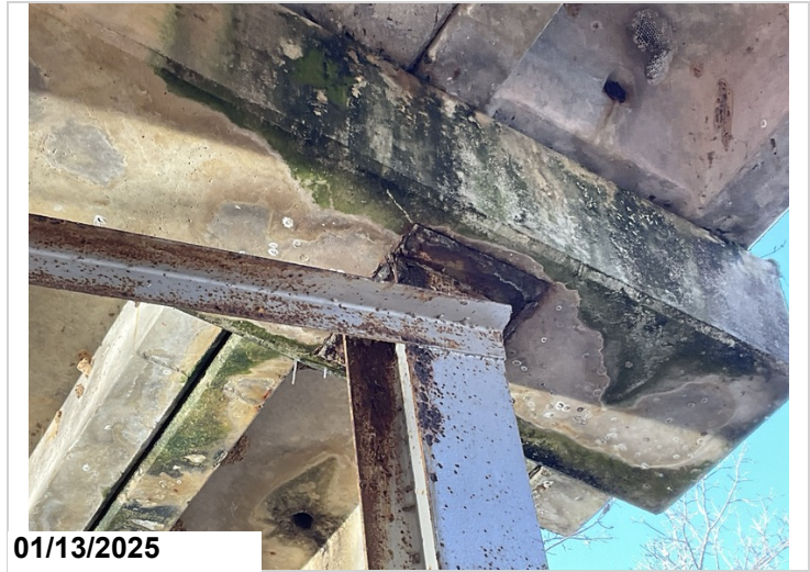
Bent 4, Piles 1 - 4: Active corrosion with flaking rust.
