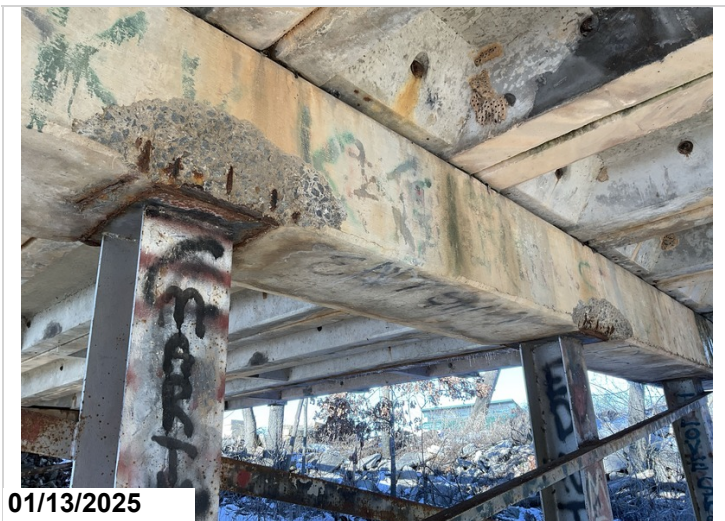
Bent 2, Piles 2 & 3, Ahead: Spalling with exposed reinforcing steel with section loss.
