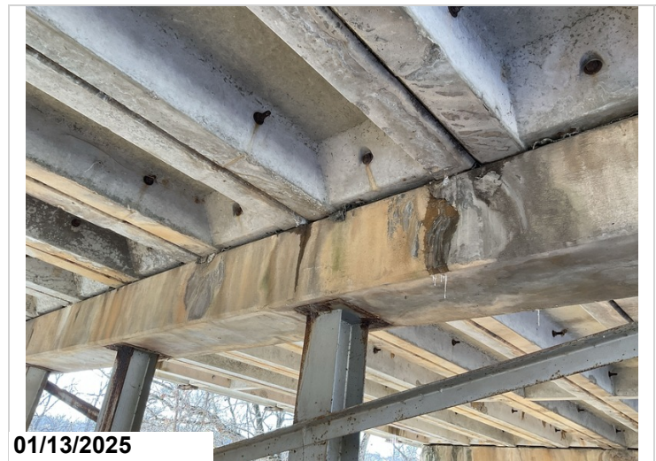
Bent 7, Channels 2 & 3, 4 & 5: Bearing Area: Spalling.
