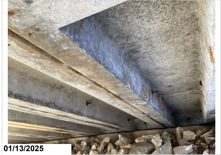
Span 1, Channel 2 & 6, Right Leg: Spalling.
