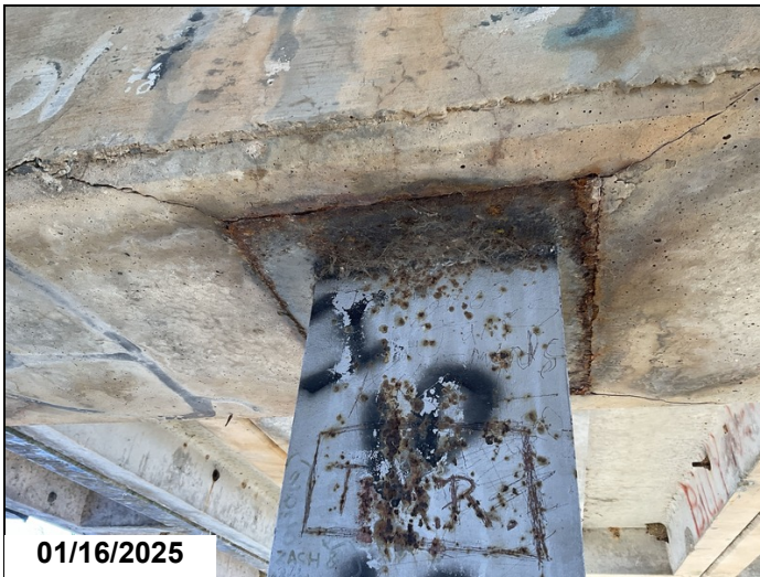
Bent 2, Piles 1 - 3: Minor active corrosion.
