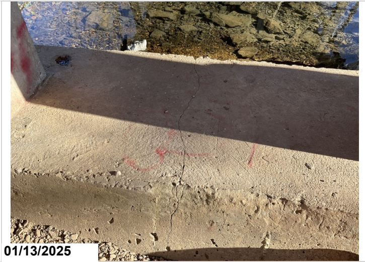
Bent 3, Between Piles 2 & 3, 3 & 4: Cracking.
