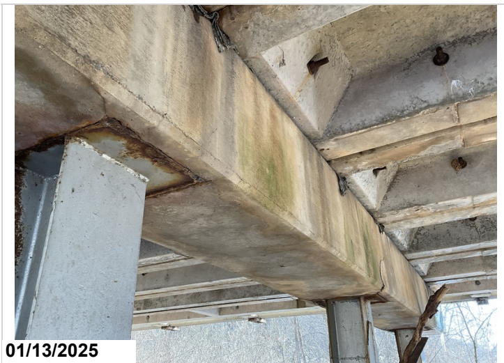
Bent 8, Piles 2 & 3, Ahead & Back: Delam.
