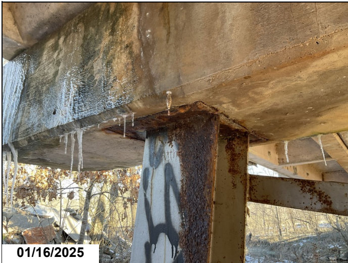
Bent 1, Pile 1: Active corrosion with flaking rust.
