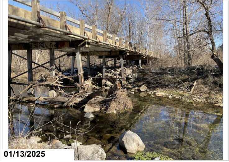
Large boulders added to channel.
