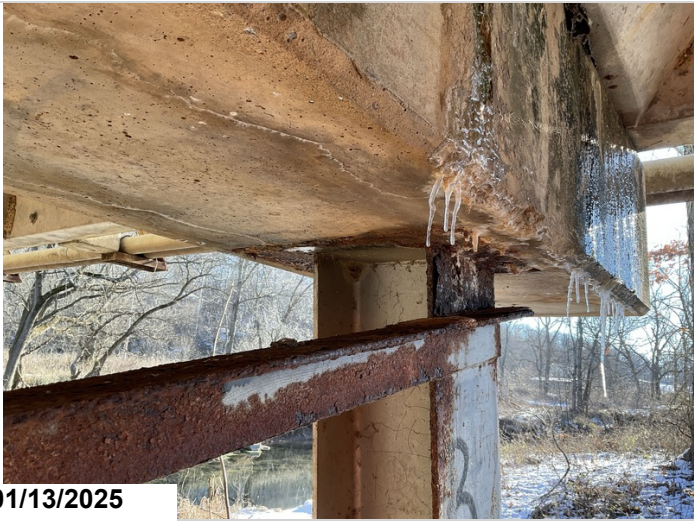
Bent 2, Pile 4: Active corrosion with flaking rust.
