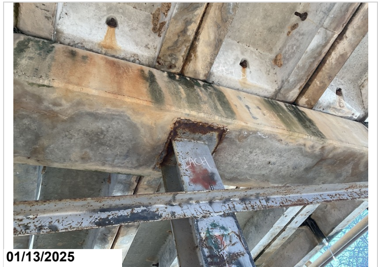
Bent 3, Piles 1 - 4: Minor active corrosion.
