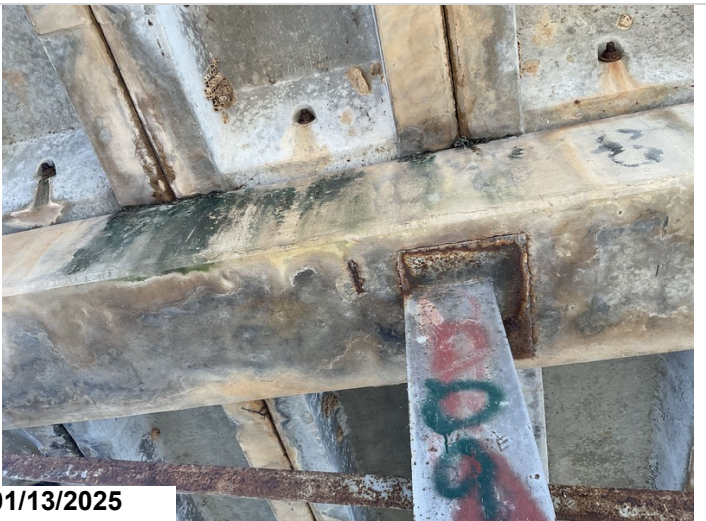
Bent 3, Adjacent to Pile 2: Spalling with exposed reinforcing steel with section loss.
