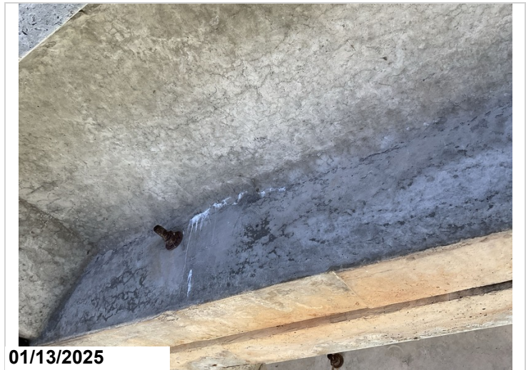
Span 1, Channel 2, 4 & 6: Longitudinal cracking with efflorescence.
