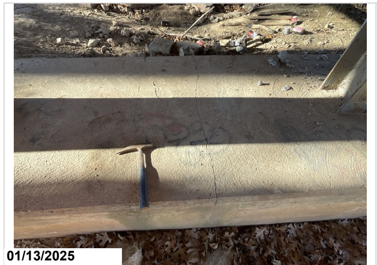
Bent 2, Footing: Cracking.
