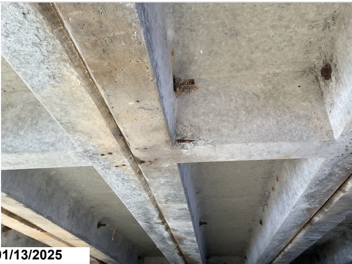
Span 1, Channel 3, Diaphragm: Spalling with exposed reinforcing steel with section loss.
