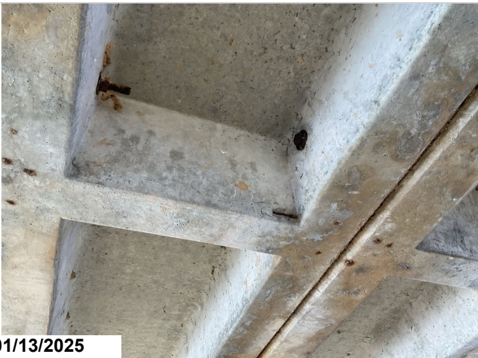
Span 2, Channel 4, Diaphragm: Spalling with exposed reinforcing steel with section loss.
