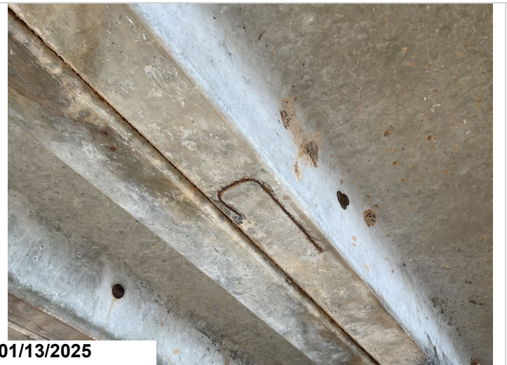
Span 2, Channel 6: Spalling with exposed reinforcing steel with section loss.
