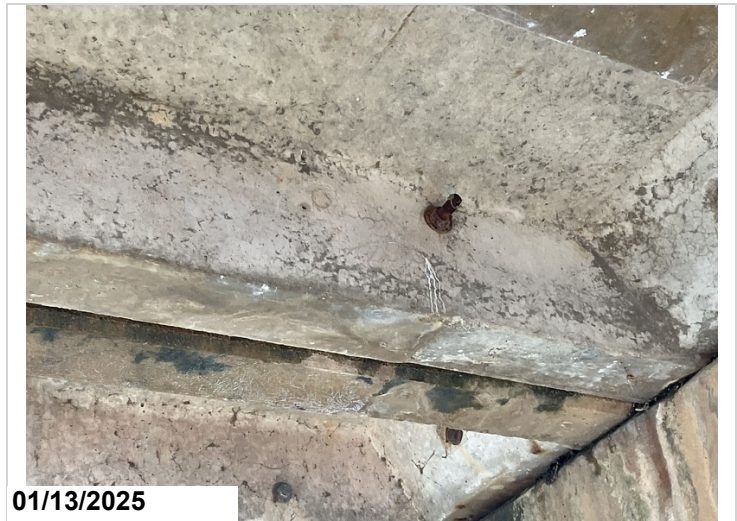
Span 6, Channels 2 - 7, Near Bolts: Cracking with efflorescence.
