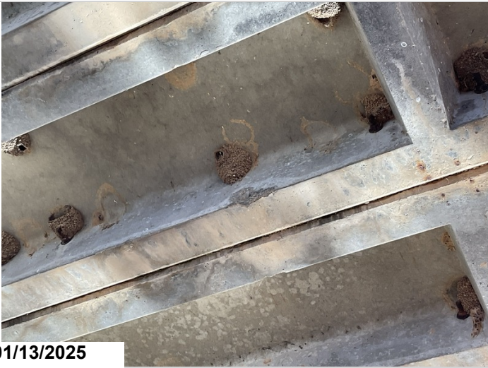
Span 4, Channels 3 & 5: Minor spalling.
