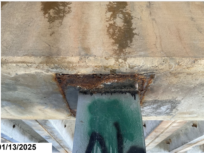
Bent 1, Pile 2 & 4: Minor active corrosion.
