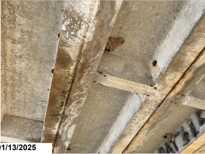
Span 3, Channel 7, Diaphragm: Delam.
