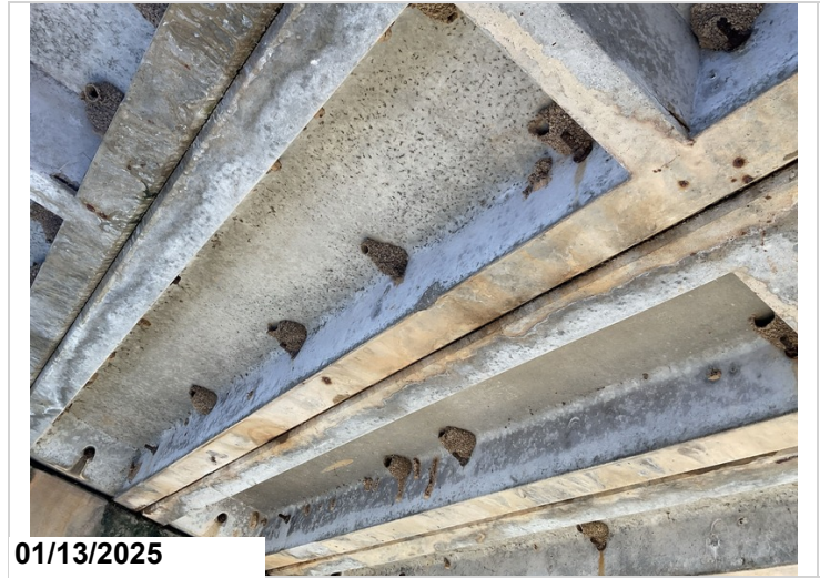
Span 3, Channels 2 - 5: Minor spalling.
