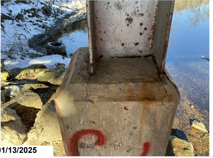
Bent 3, Piles 1 - 4, Concrete Encasement: Cracking.
