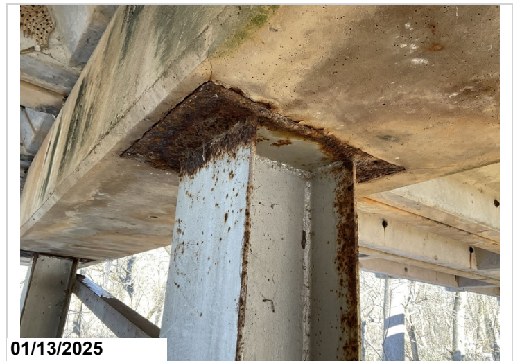
Bent 6, Piles 1 - 4: Active corrosion with flaking rust.
