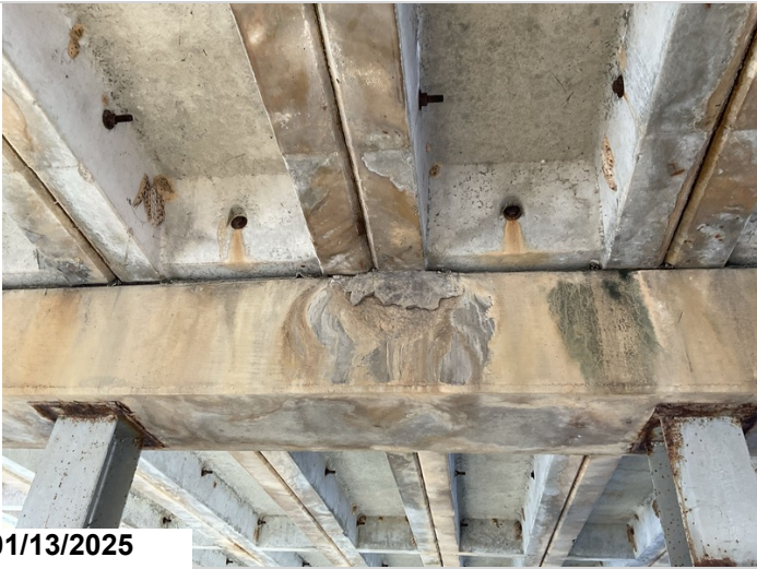
Bent 7, Channels 4 & 5, Bearing Area: Spalling.
