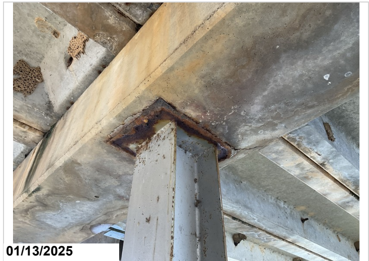
Bent 5, Piles 1 - 4: Active corrosion with flaking rust.
