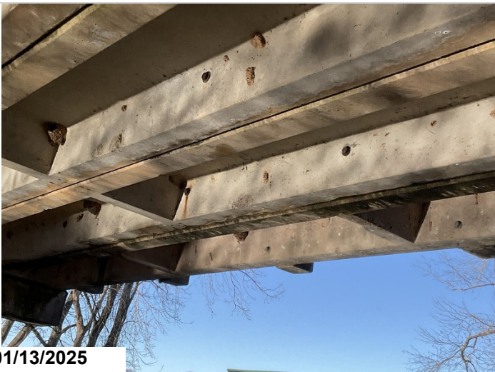
Span 5, Channels 2, 3, 6 & 8: Minor spalling.
