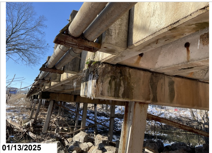
Bent 6, Right: Spalling.
