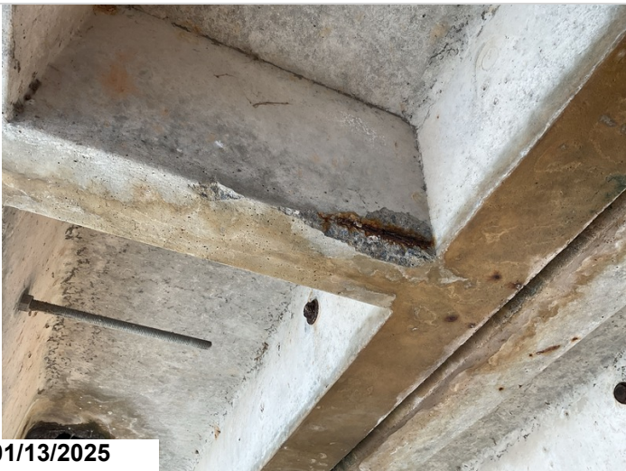
Span 2, Channel 8, Diaphragm: Spalling with exposed reinforcing steel with section loss.
