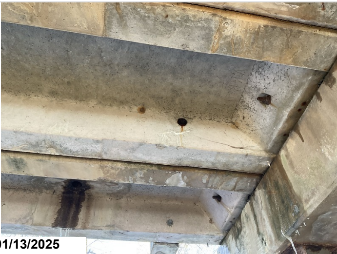
Span 7, Channels 2, 4 & 5: Cracking with efflorescence.
