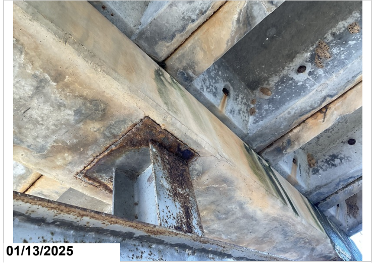
Bent 3, Pile 2, Ahead: Delam.
