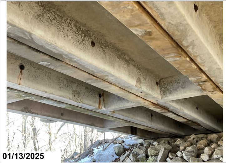
Span 9, Channels 1 - 8: Minor spalling.
