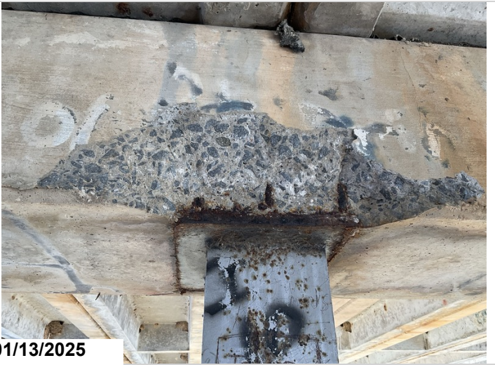
Bent 2, Pile 3, Back: Spalling with exposed reinforcing steel with section loss.
