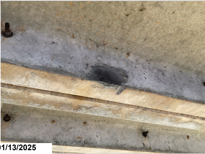
Span 2, Channel 3: Failing repair.
