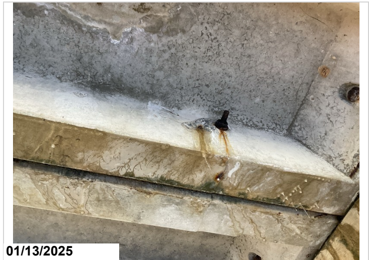
Span 7, Channel 1: Spalling with exposed reinforcing steel with section loss.
