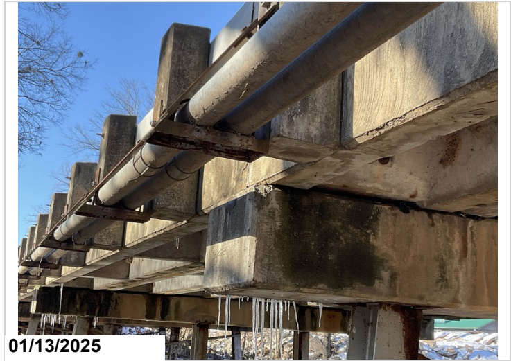
Bent 5, Right: Spalling.
