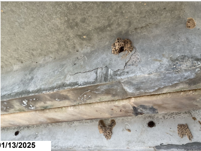
Span 6, Channel 5, Left Leg: Delam.
