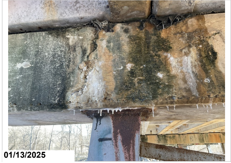
Bent 2, Back, Left & Right: Cracking with efflorescence with build up.
