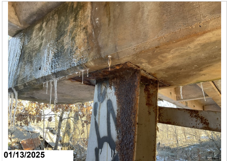
Bent 1, Pile 1: Active corrosion with flaking rust.
