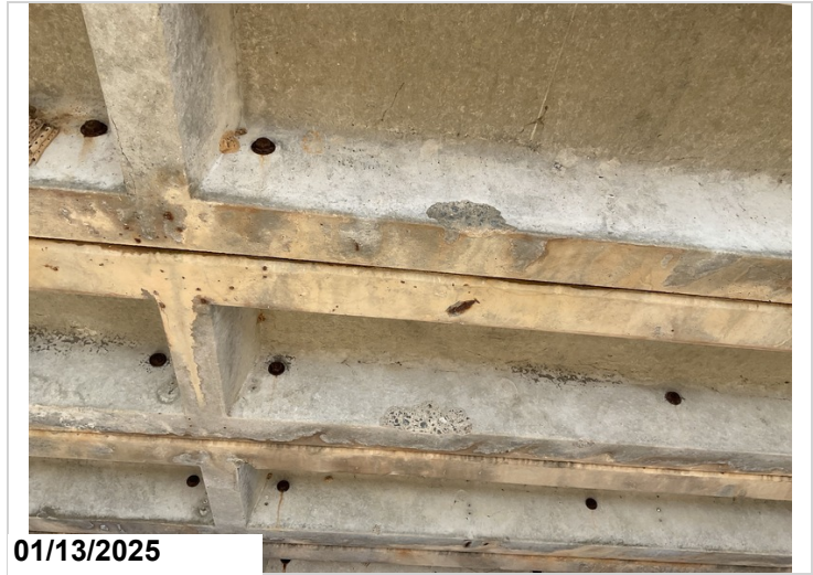
Span 7, Channels 1 & 3 - 8: Minor spalling.
