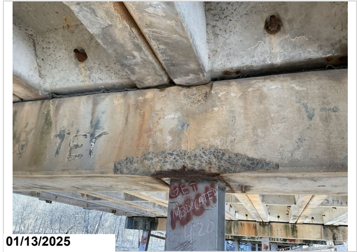
Bent 2, Pile 3, Back: Spalling.
