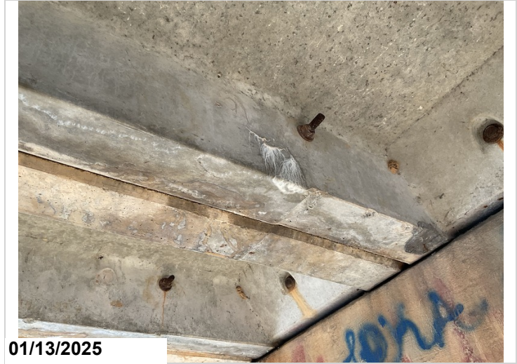
Span 2, Channel 5: Cracking with efflorescence with build up.
