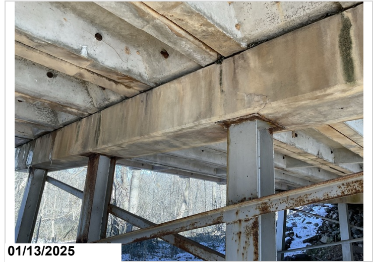
Bent 7, Piles 2 & 3: Delam.
