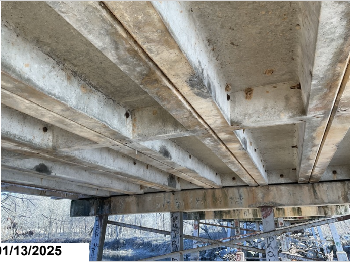
Span 2, Channels 4 - 8: Failing repairs.
