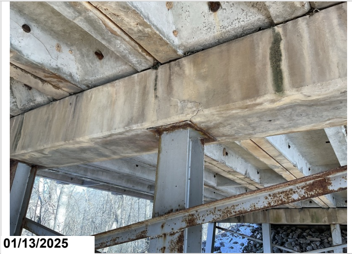
Bent 7, Piles 1 - 4: Active corrosion with flaking rust.
