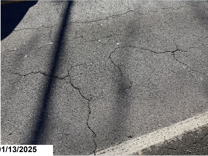
Spans 1 - 8, Wearing Surface: Moderate cracking.
