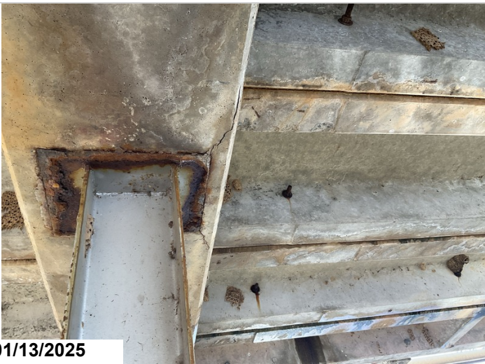
Bent 5, Pile 2, Ahead: Delam.
