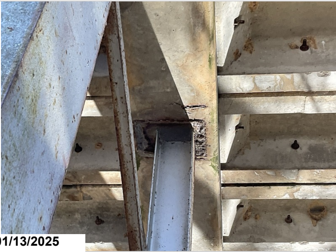
Bent 2: Spalling with exposed reinforcing steel with section loss.
