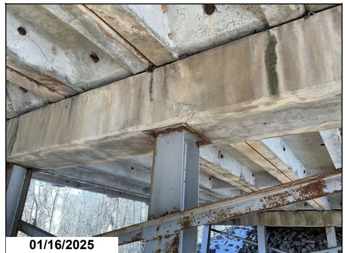
Bent 7, Piles 1 - 4: Active corrosion with flaking rust.
