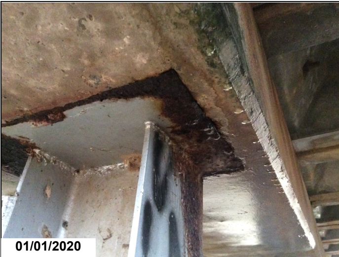
Bent #1, pile #1-Corrosion to top plate and piling.
