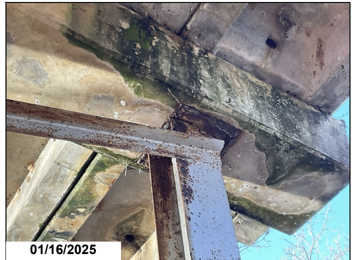
Bent 4, Piles 1 - 4: Active corrosion with flaking rust.
