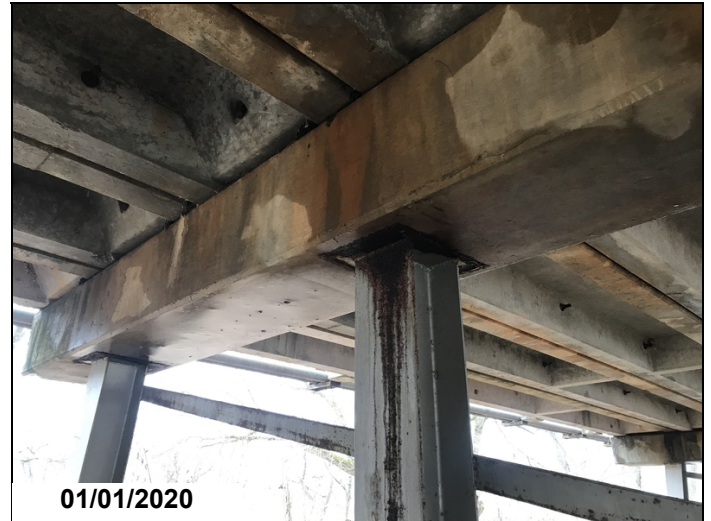
Typical failing paint system of steel piling.
