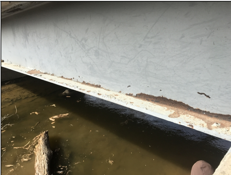
Paint system failure.
