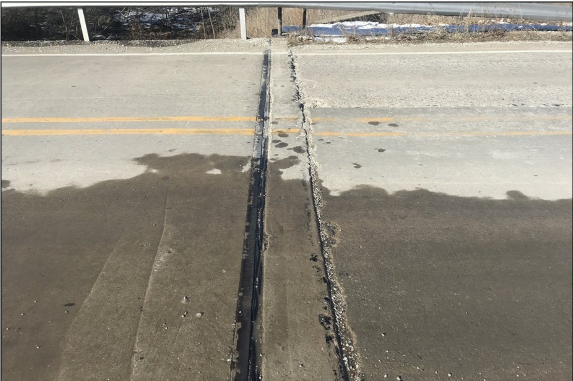
Abutment #2 top of the backwall spalling along the approach slab.
