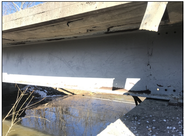
Beam 4-Failing paint with rust forming.
