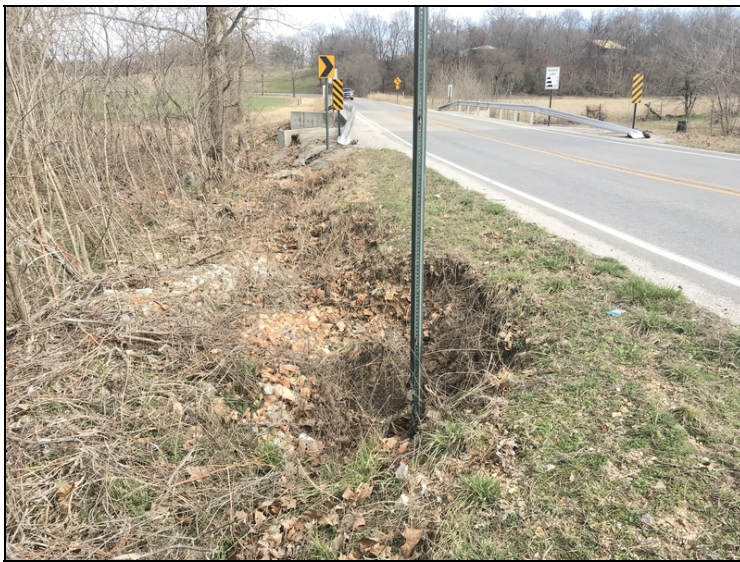
The North embankment of the West approach roadway has erosion that is nearing the approach roadway.
