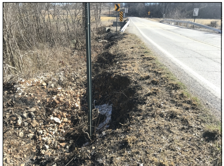
The North embankment of the West approach roadway has erosion that is nearing the edge of approach roadway.
