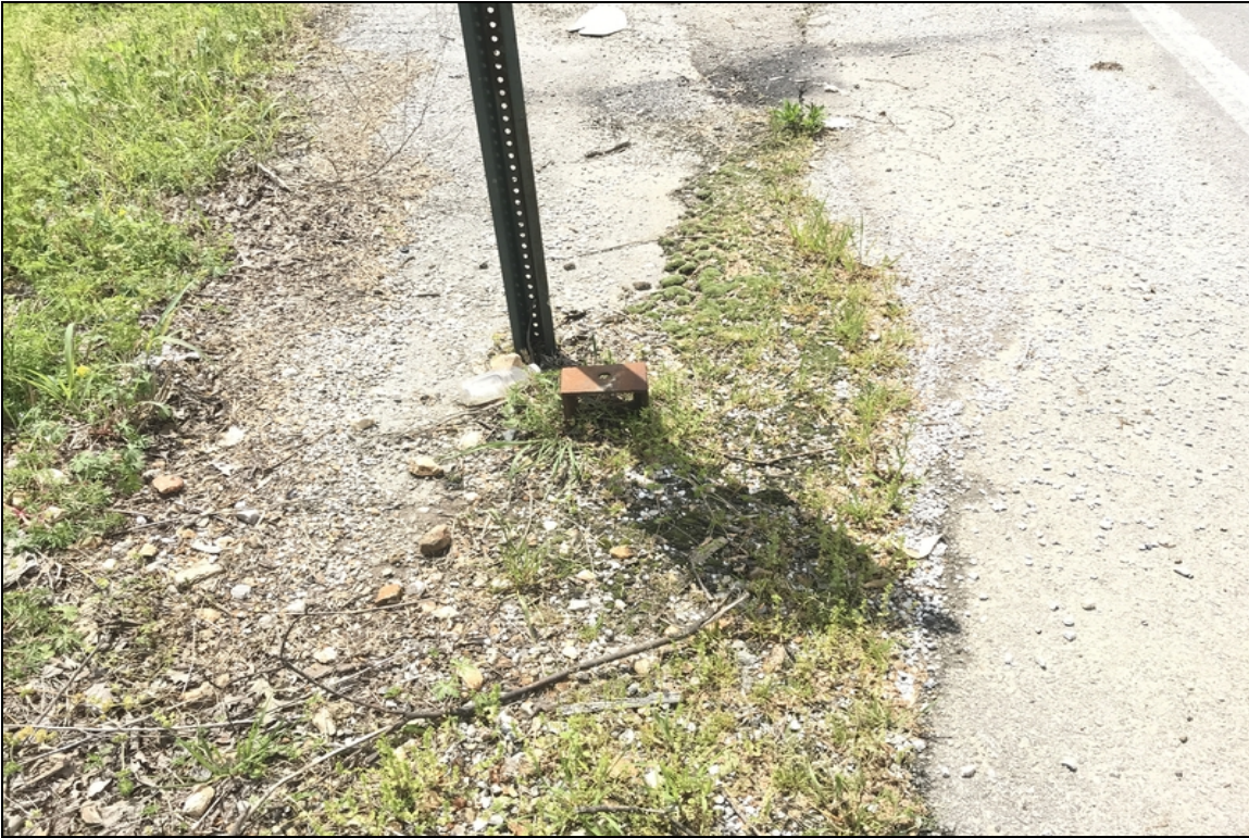
Ground Anchorage for Southeast approach railing.
