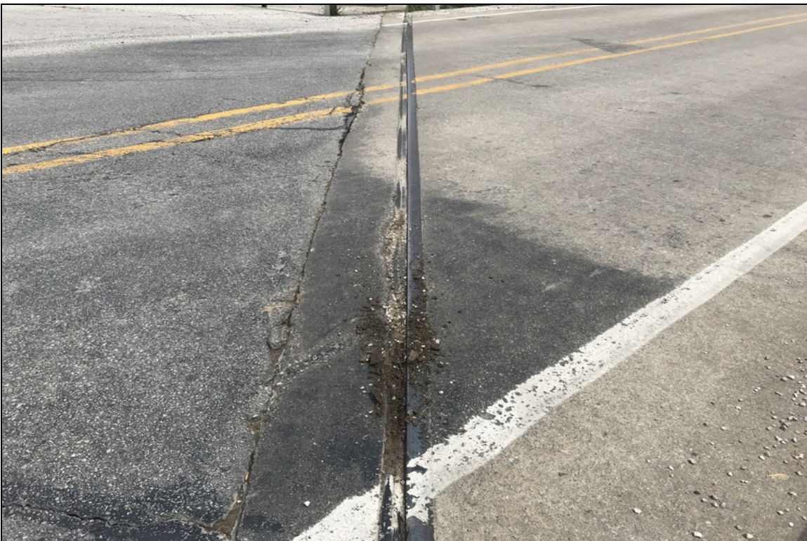
Abutment 1 compression joint seal.
