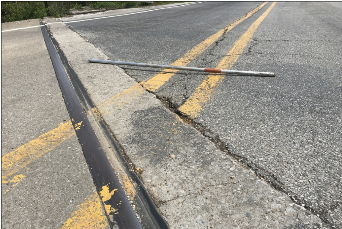
Settlement in East approach roadway at centerline.
