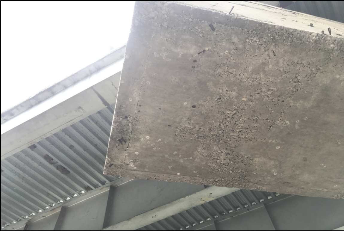
Bent 2 cap, right undersurface-Honeycombing with exposed secondary steel.
