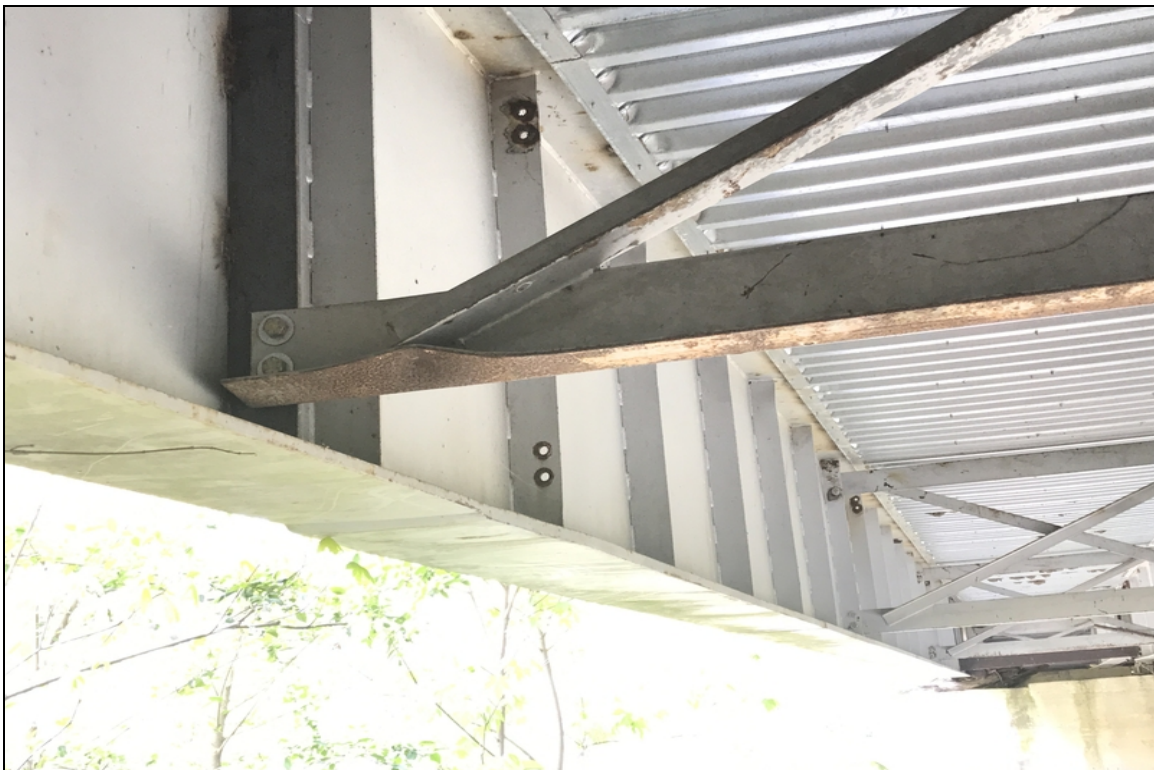
Cross frames have minor out of plane bending to the bottom angles in some locations.
