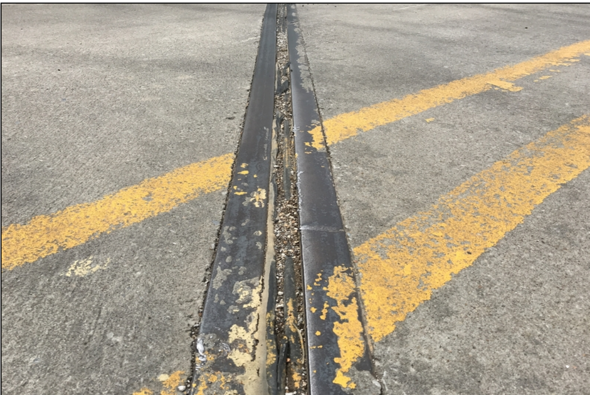
Bent 2 expansion joint has areas of rips, tears and adhesion failure.
