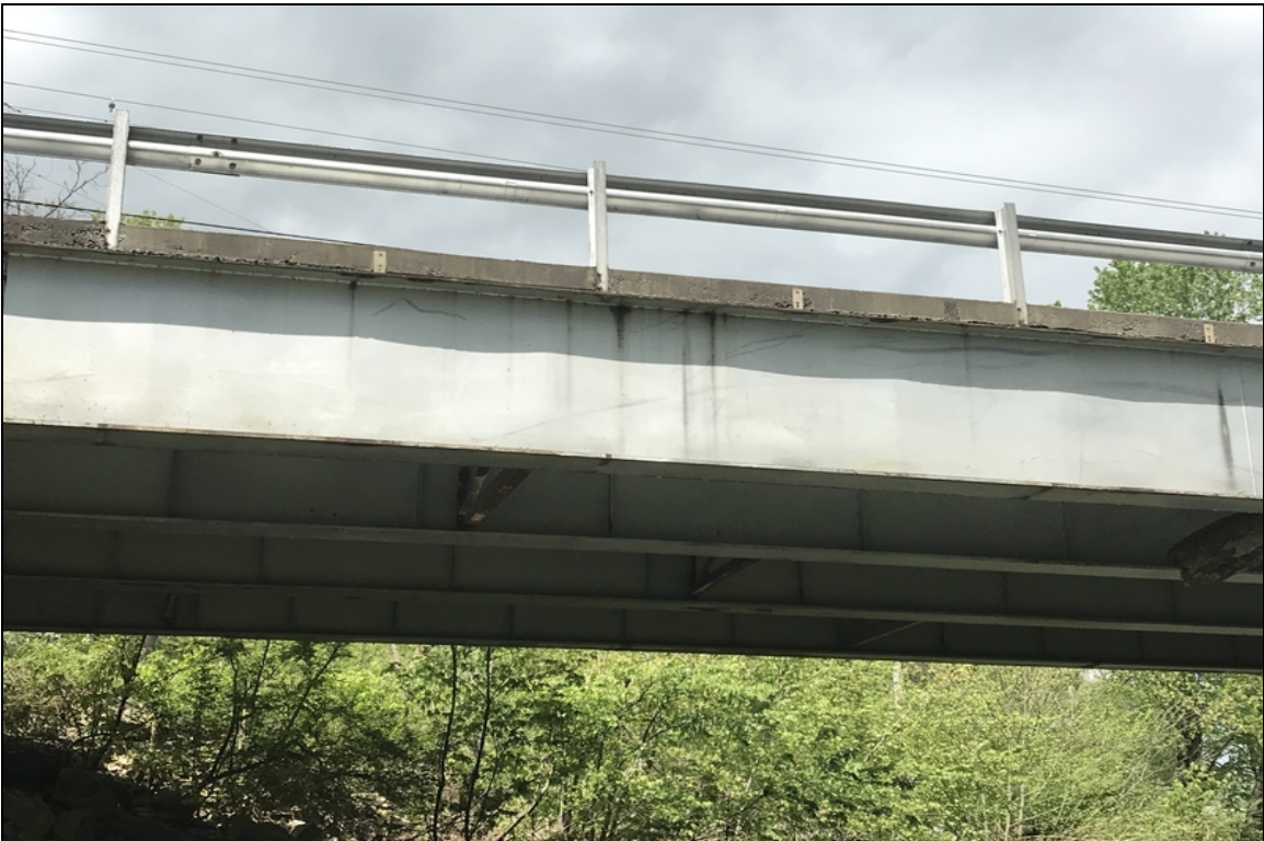
Beam 4 of span 1-Scuff marks from drift impacts.
