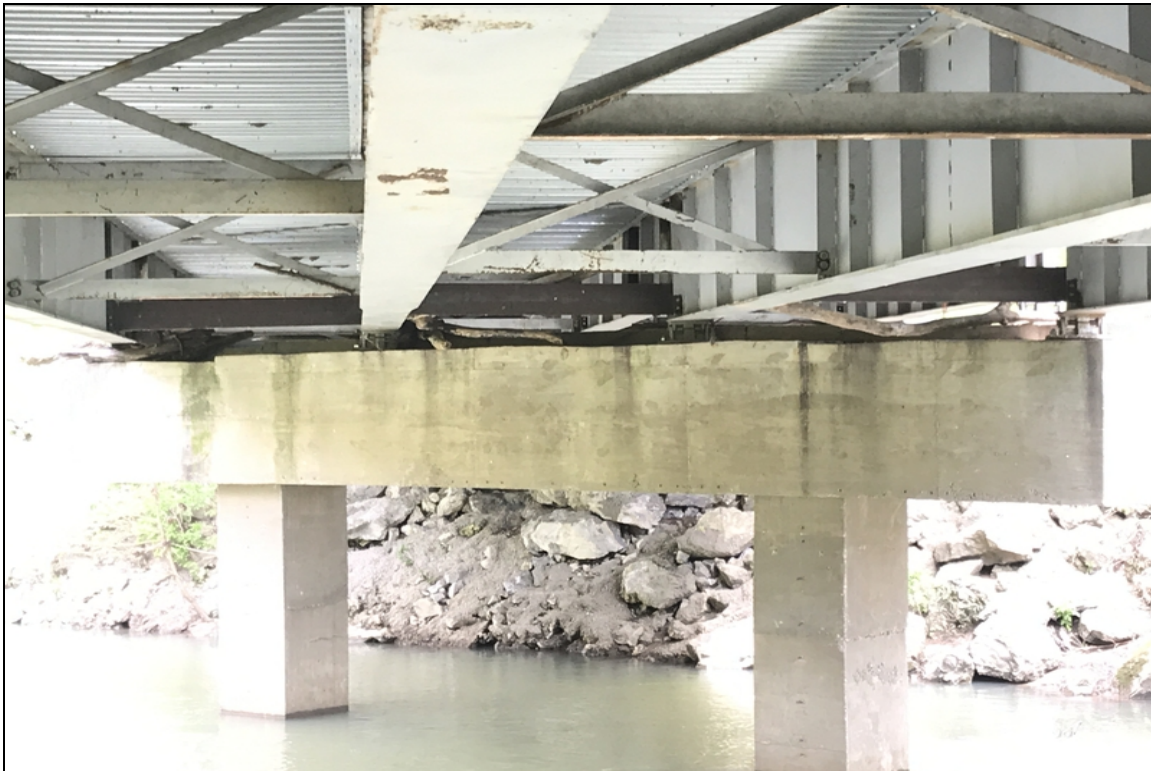
Drift accumulation on bent 2 cap.
