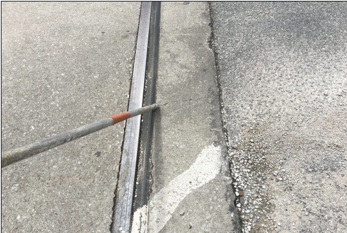
Abutment 1-Transverse cracking in top of backwall.
