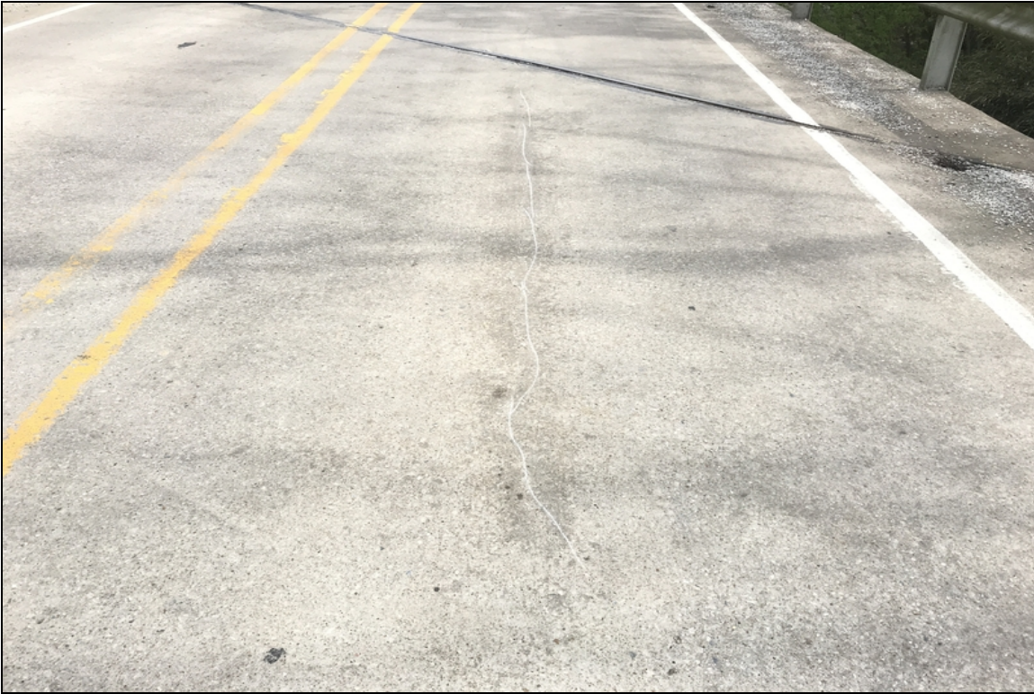
Span 1, right lane-Longitudinal cracking.
