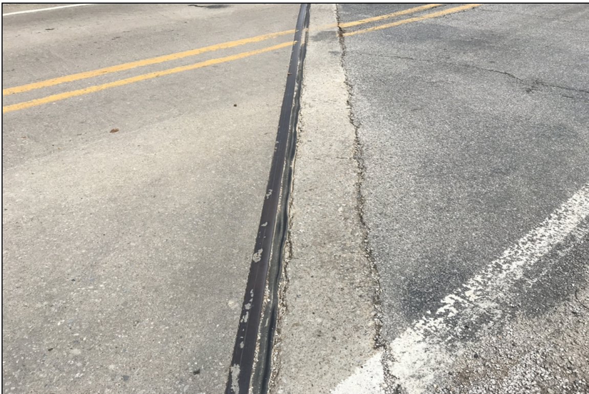
Abutment 2-Transverse cracks.
