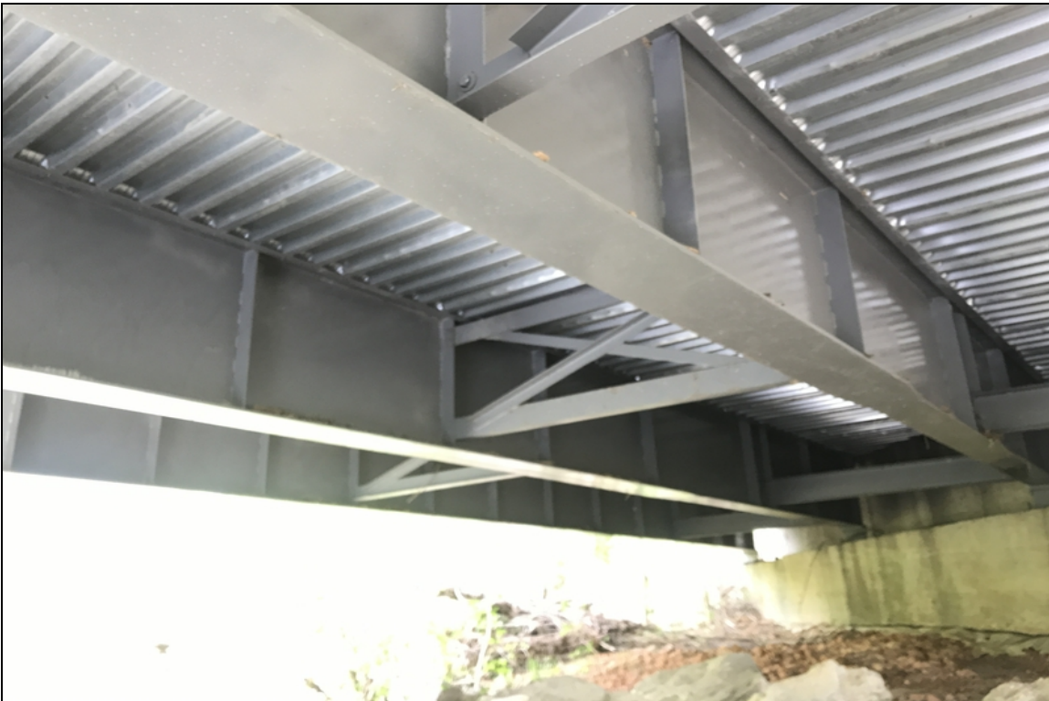
The beams in span 2 have been painted from mid-span to abutment 2.
