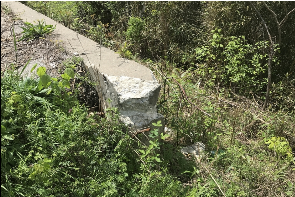
Spall to end of Northeast wing wall.
