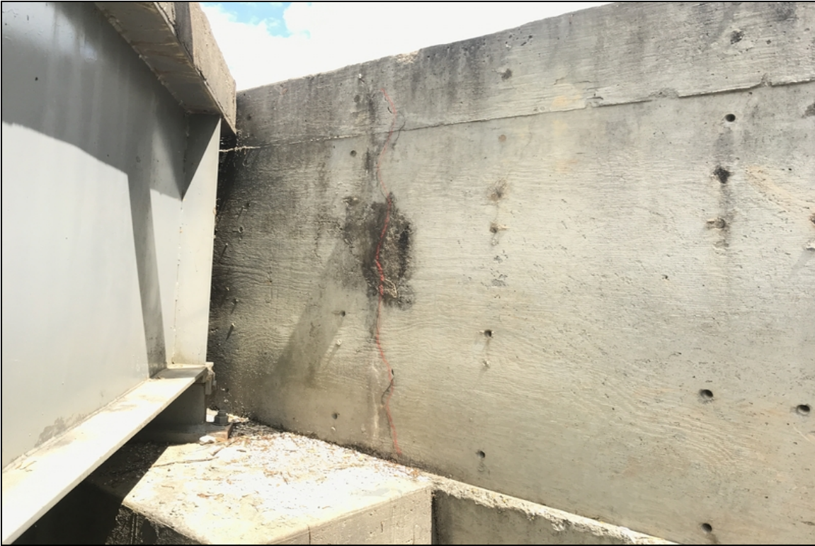
The right exterior side of abutment 2 backwall has a vertical and diagonal crack.
