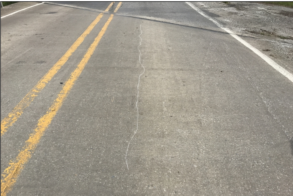
Span 2, right lane-Longitudinal cracking.
