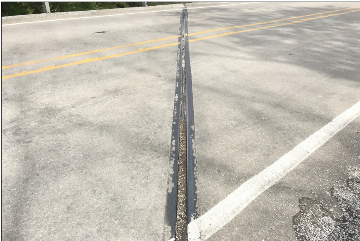
Bent 2 expansion joint.
