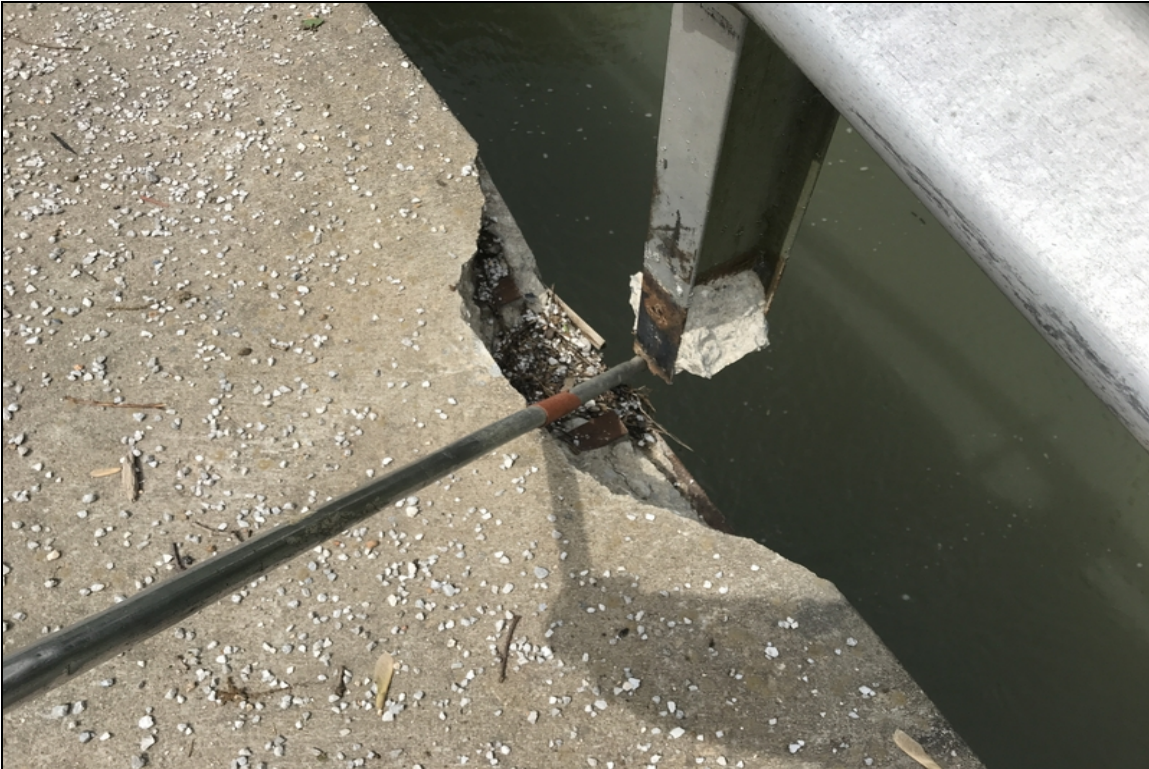
Left bridge railing in span # 1 has collision damage over bent # 2 that has created a locket in the railing and has fractured / spalled a 2' long area of the edge of the deck where one of the railing post was incorporated into the deck.
