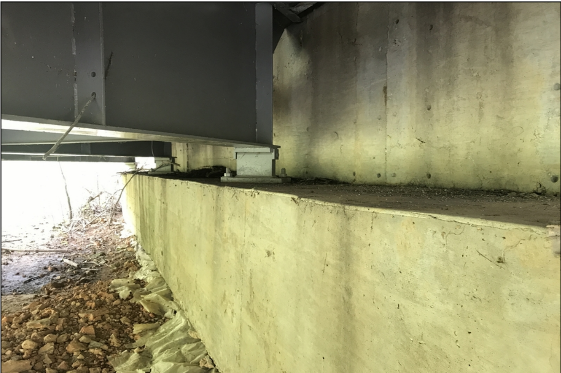
Abutment 2 bearing area.
