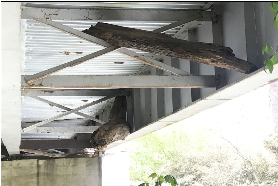
Span 1-Drift in superstructure.
