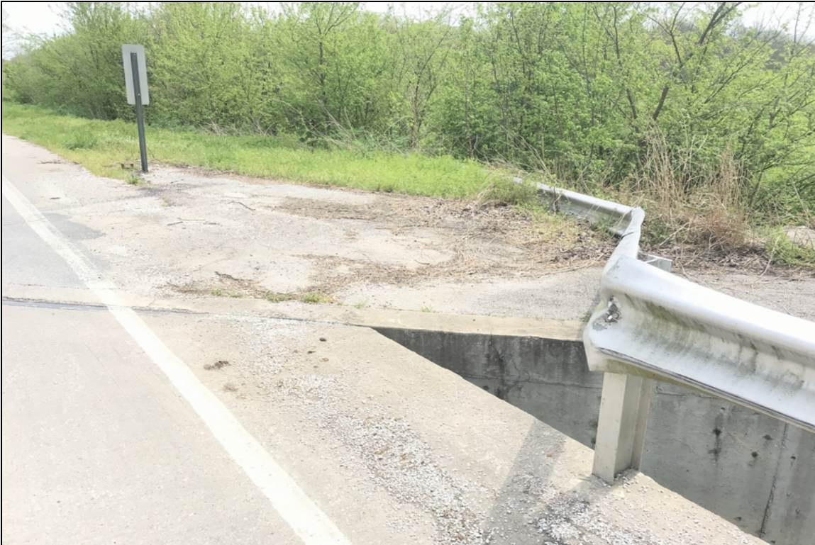
The Southeast approach railing has collision damage that has broken the railing loose from the ground anchorage and destroyed the turndown section of railing.
