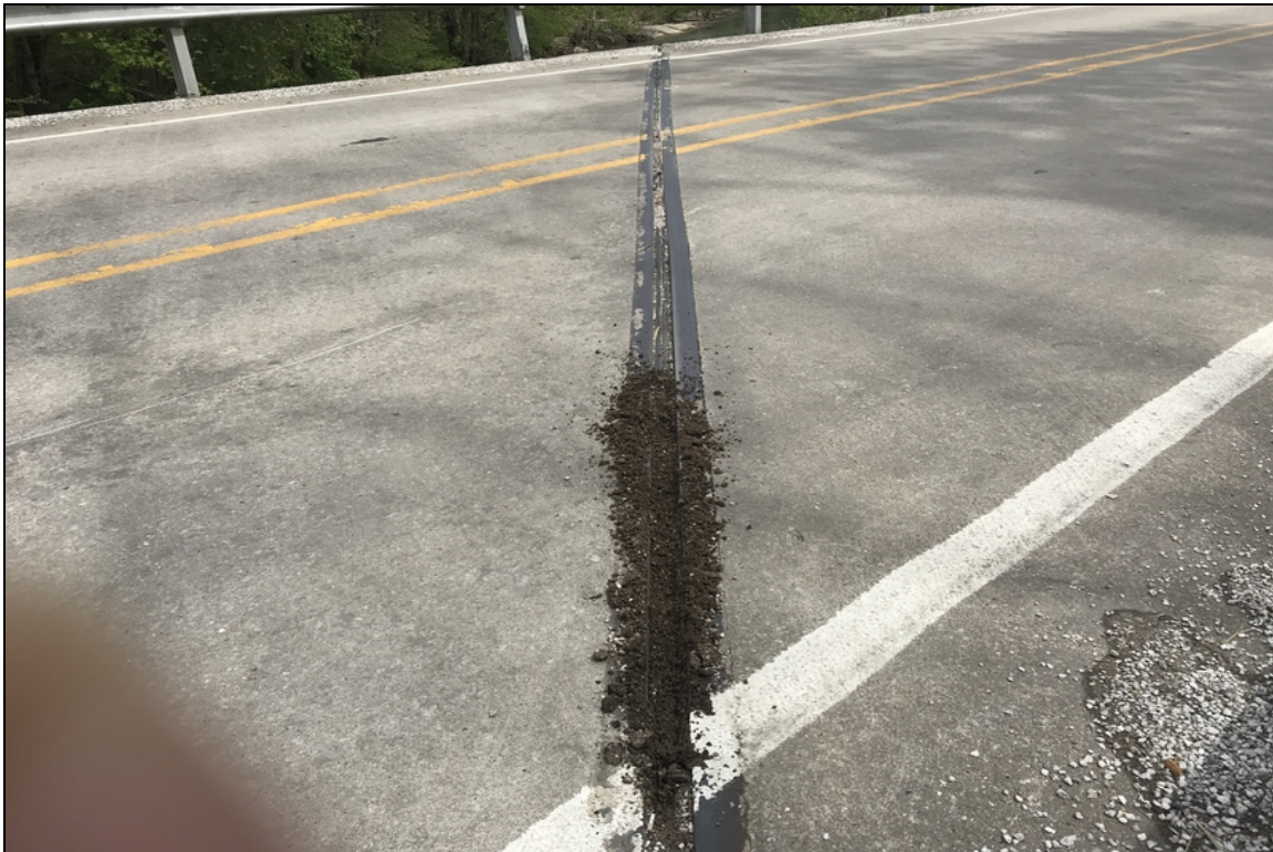
Bent 2 expansion joint sagging in locations.
