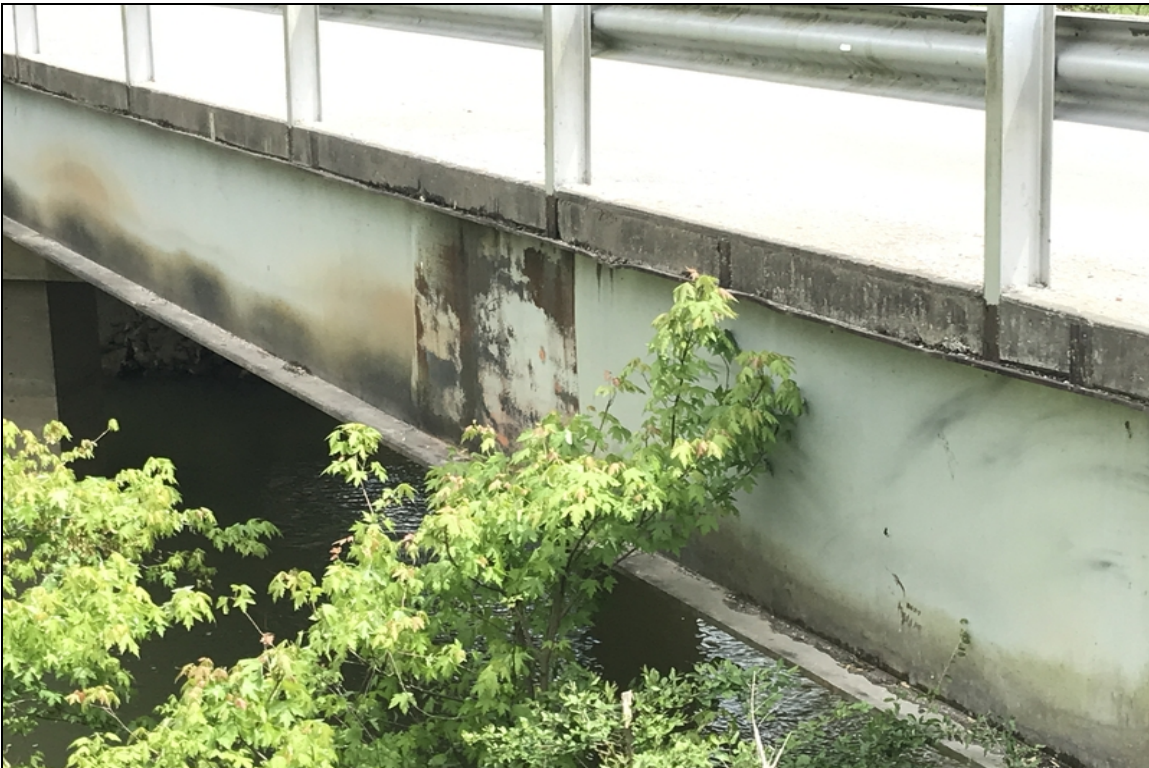
Span 1, beam 1-Rust forming.
