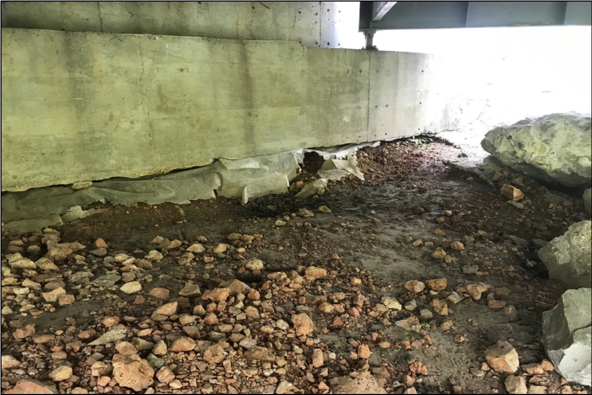
The East embankment at the base of abutment # 2 has minor earth settlement / erosion.
