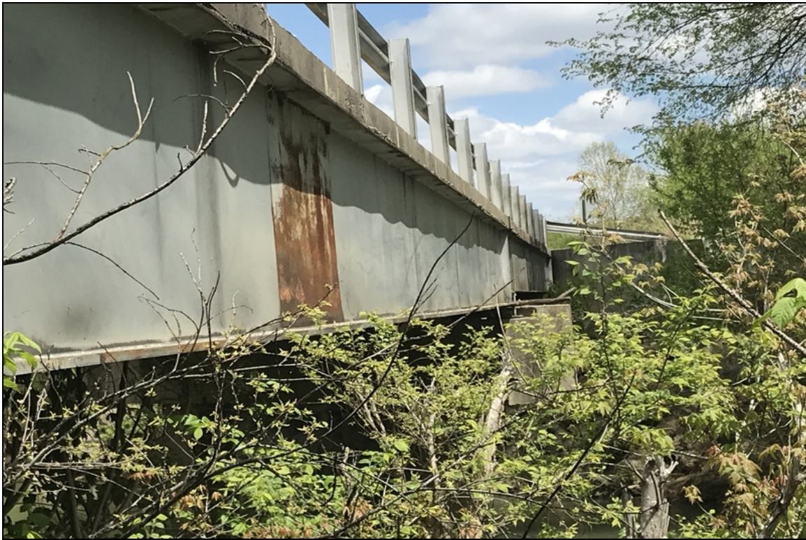
Span 1, Beam 4-Area of paint failure with rust coating.
