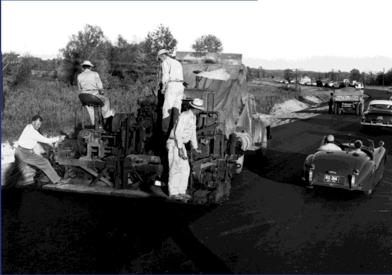
WIDENING OF HWY. 67 NEAR MALVERN
