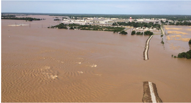
Breached Levee near Pocahontas, Arkansas
