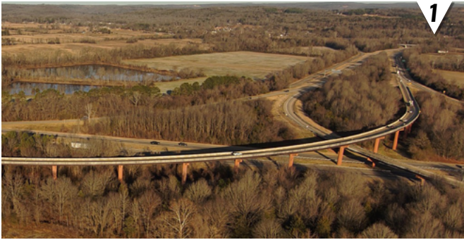
1. BRIDGE OPERATIONS — Aerial photo of Interstate 40/Interstate 49 over Frog Bayou by Austin Janes, Statewide Bridge Inspector.
