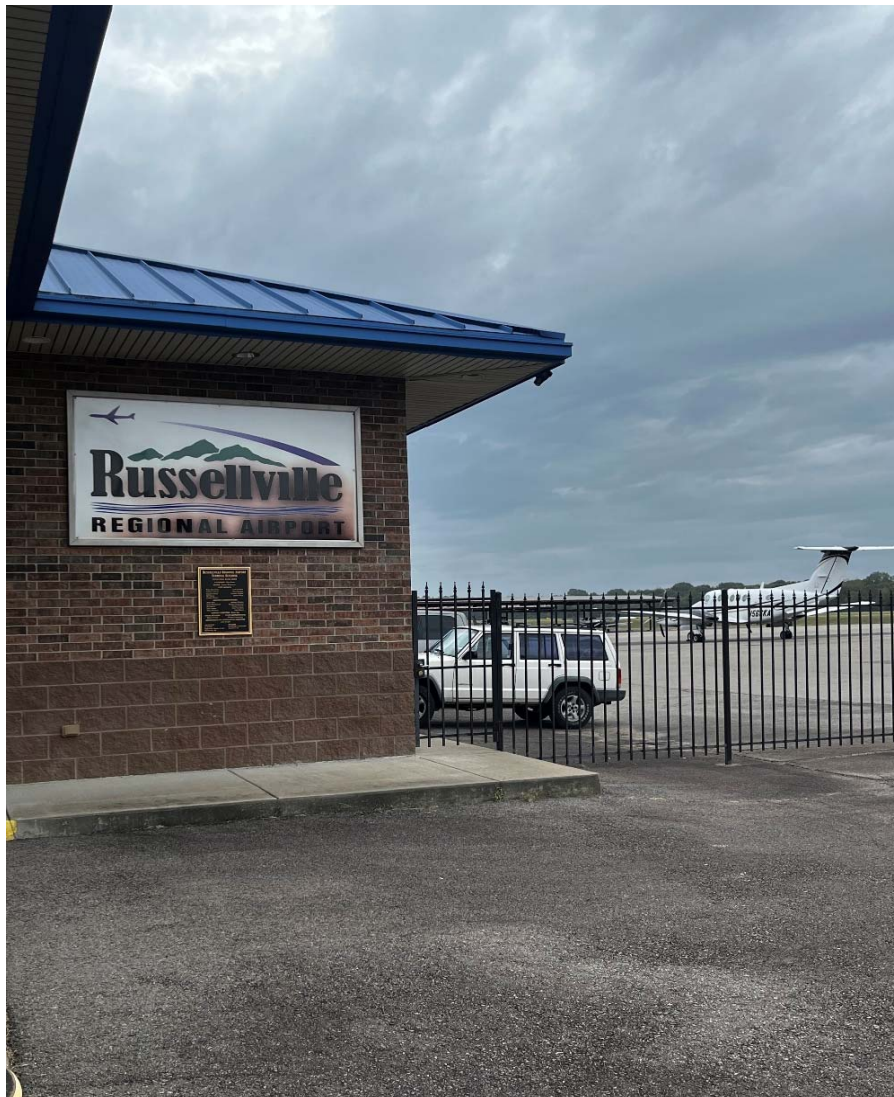
Russellville Regional Airport, Highway 980, Section 31, Pope County
