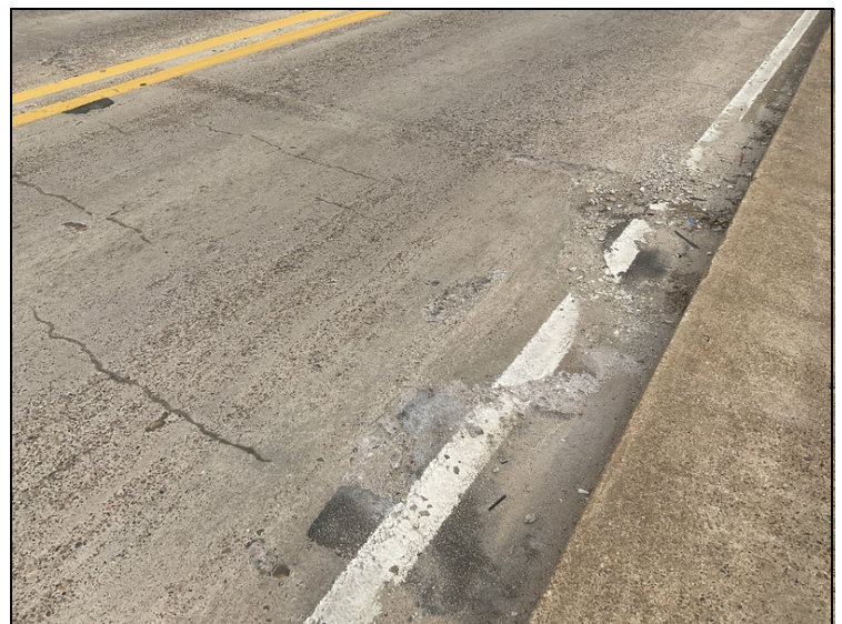
Span 3 spalls in deck
