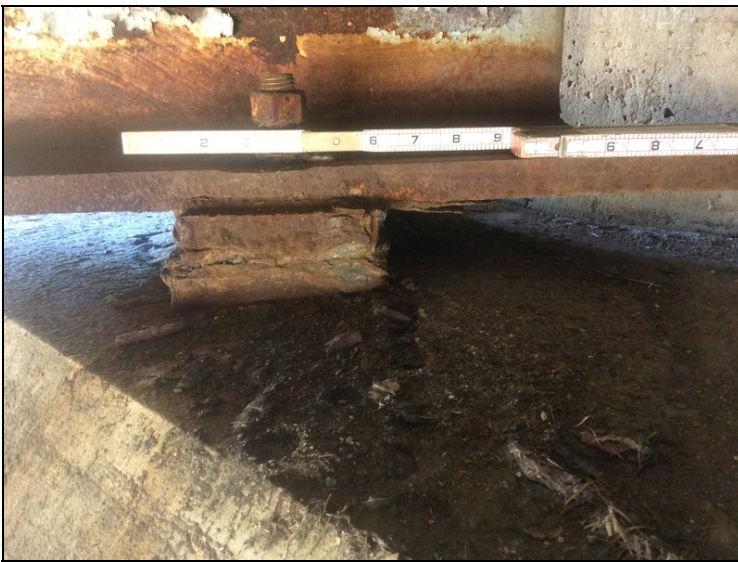
Bent 1 beam 5 bearing has corrosion.
