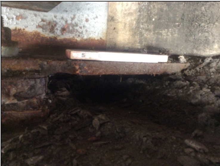
Bent1 beam 4 up to 3/16" pitting to bottom flange at bearing area.
