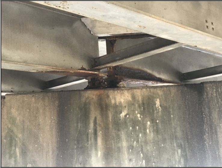
Span 3, girder 3: large area of measurable section loss to the bottom flange and lower web and at the haunch
