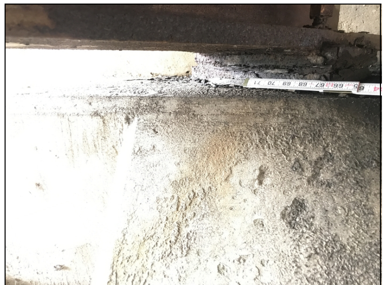
Bent 1, girder 5 bearing with extensive corrosion. Common to all bearings on this bridge.
