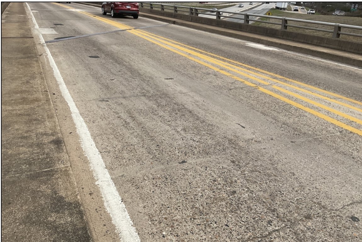
Both mines have minor abrasion/wear
