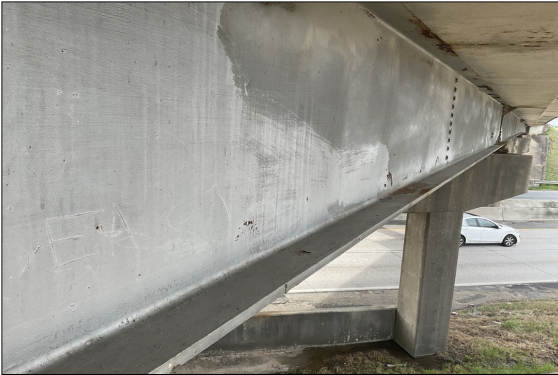
Typical paint condition
