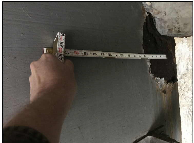
Span 4, girder 1 at bent 5: laminating rust to haunch area.
