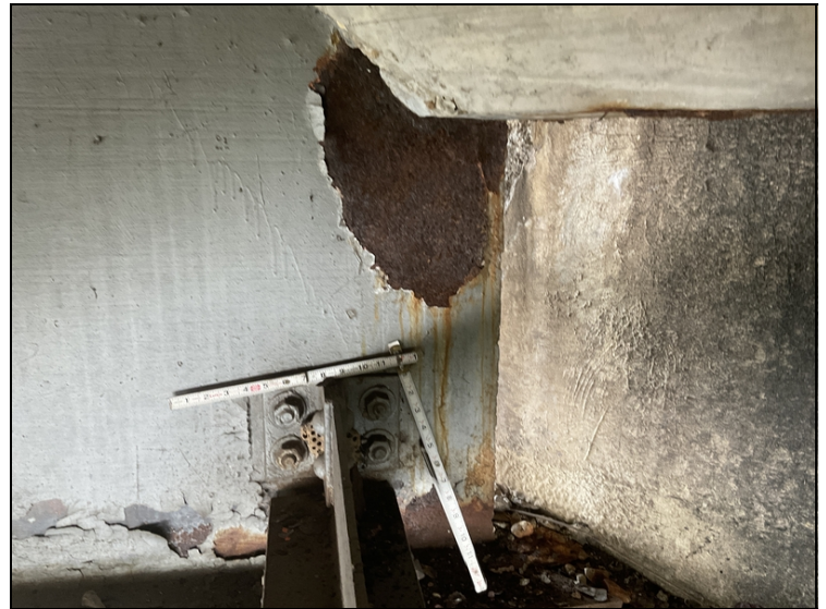
Bent 5 beam corrosion in haunch area with pitting up to 3/16"
