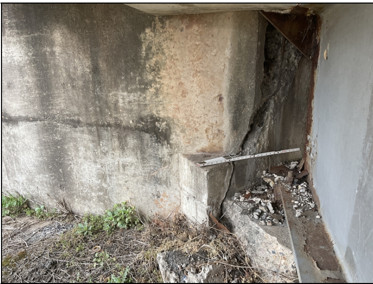
Left side of bent 5 has 1" crack and large spall with exposed rebar
