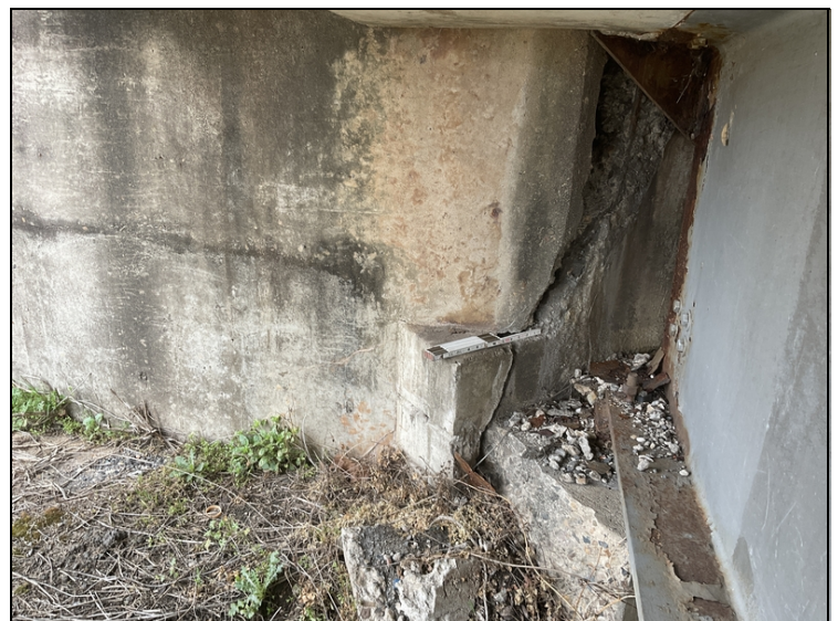
Bent 5 left side spall at left end of abutment, 1" crack & spall exposed rebar in back wall.
