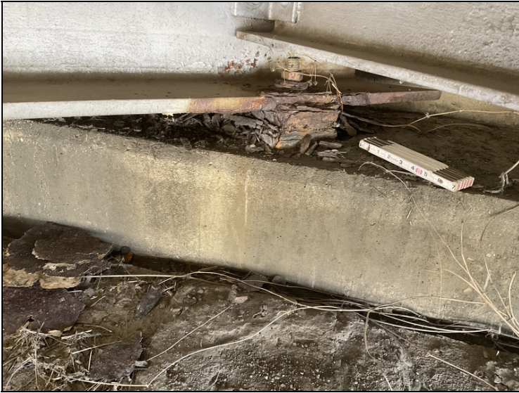
Bent 5 bearing 4 corrosion
