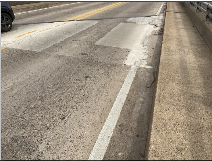
Span 2 has been patched.
